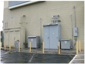
Photograph 7 - Electrical transformers and panel boxes located on the northwestern portion of the onsite structure.
