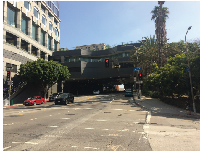
View northeast from corner of 4th Street and Olive
