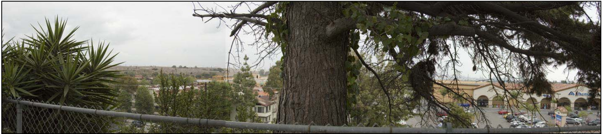
Panoramic view overlooking Western Avenue from a private residential backyard located at 21944 Pontevedra Drive. The Project site is visible to the left while Harbor features, including the Vincent Thomas Bridge, are visible to the right. As shown, the Project site is outside the viewshed of Harbor features from this location.
