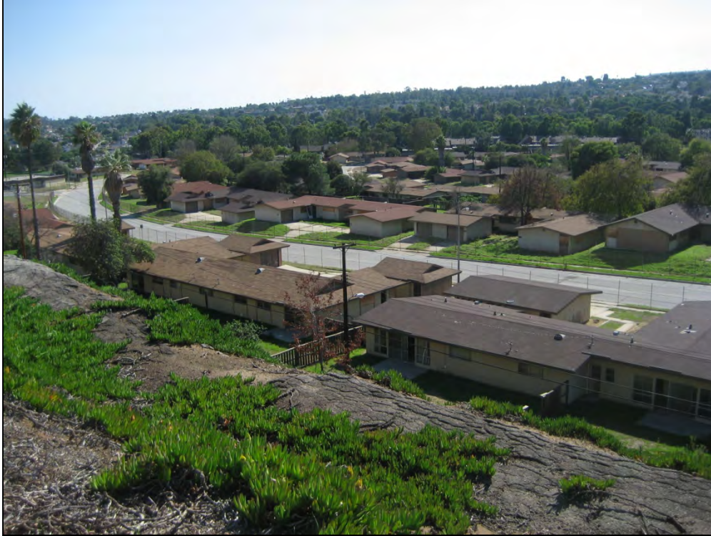
Photograph 1. Overview of housing complex, view to the southwest
