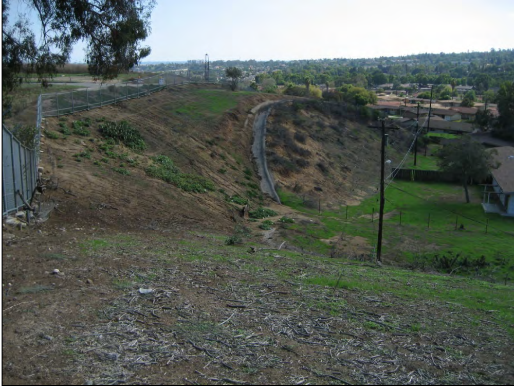
Photograph 3. Overview of sandy cut slope, view to the southeast
