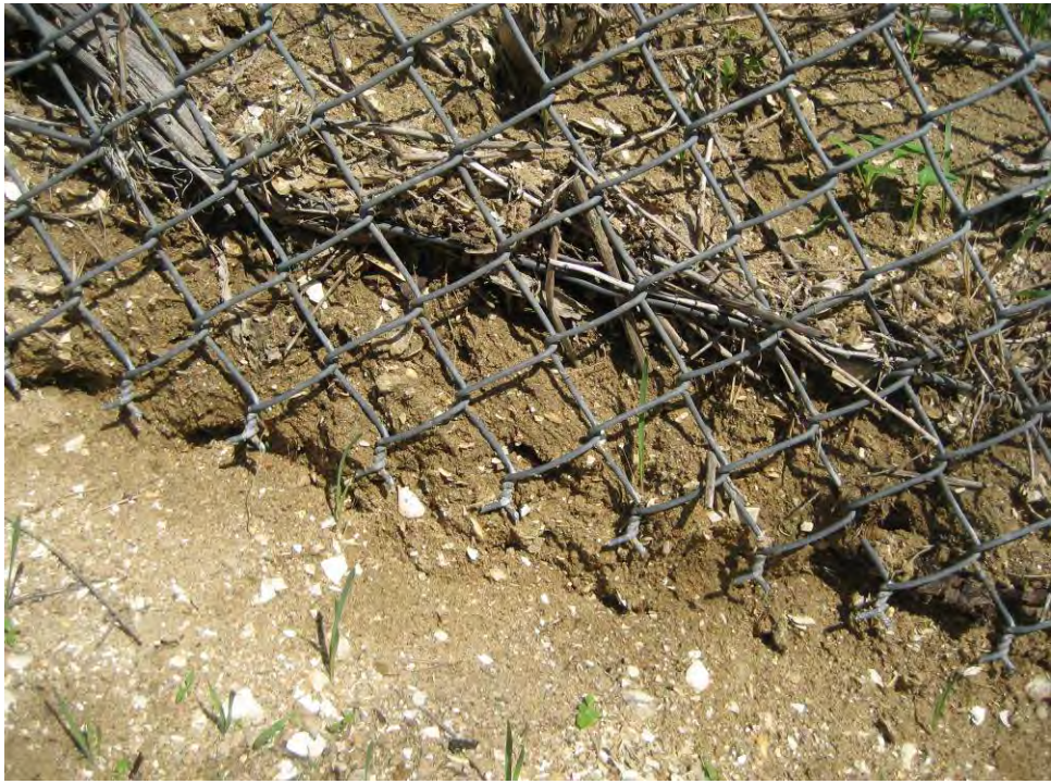
Photograph 9. Fence line along property boundary at Locality JLD102210-02.
