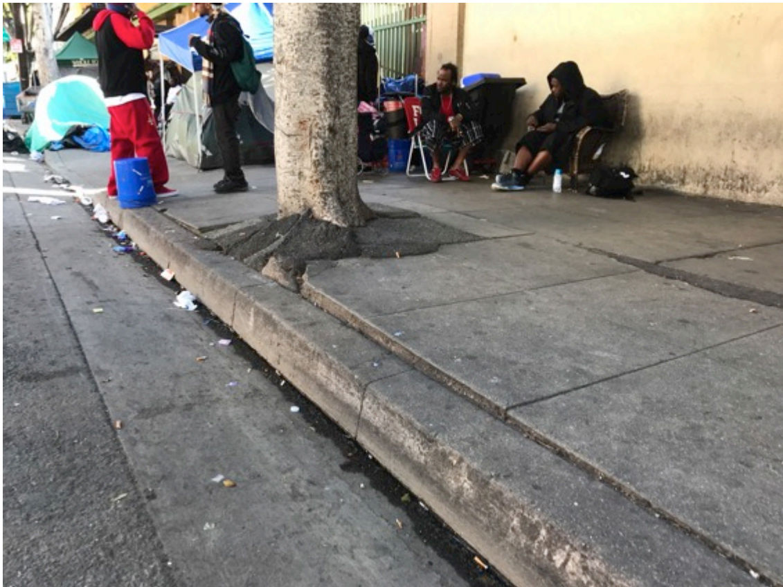
Tree well imbedded in trunk and structural damage (tree #2)
