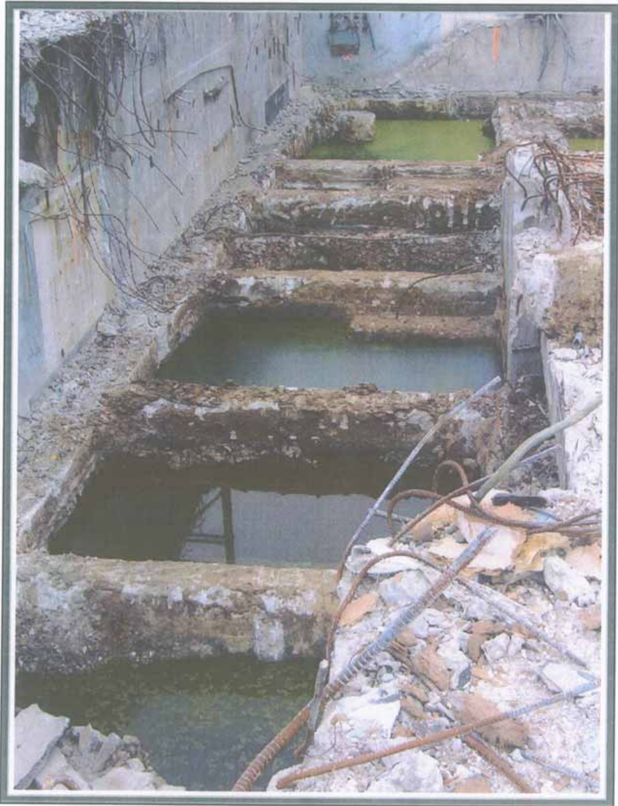
Soil Excavation and Disposal
