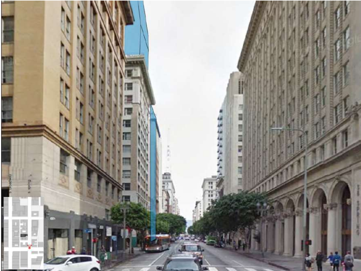
Figure 17. View Northeast Towards Project Site (Adam Sokol Architecture Practice/HLW, Inc., April 2016)
