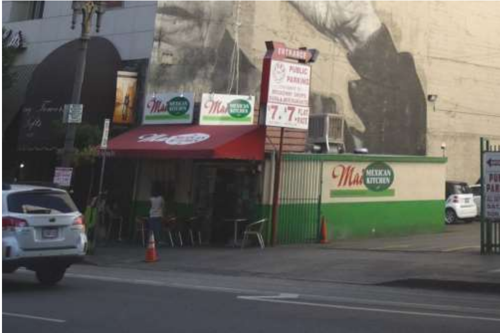
Figure 12. Mai Mexican Kitchen, a simple concrete block structure housing a small restaurant (PCR 2014)
