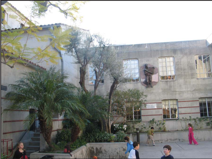
View 3: View of the 1954 building addition that created a court between the sanctuary and the Briskin wing. The concrete features slim horizontal lines of red brick on the ground floor.
