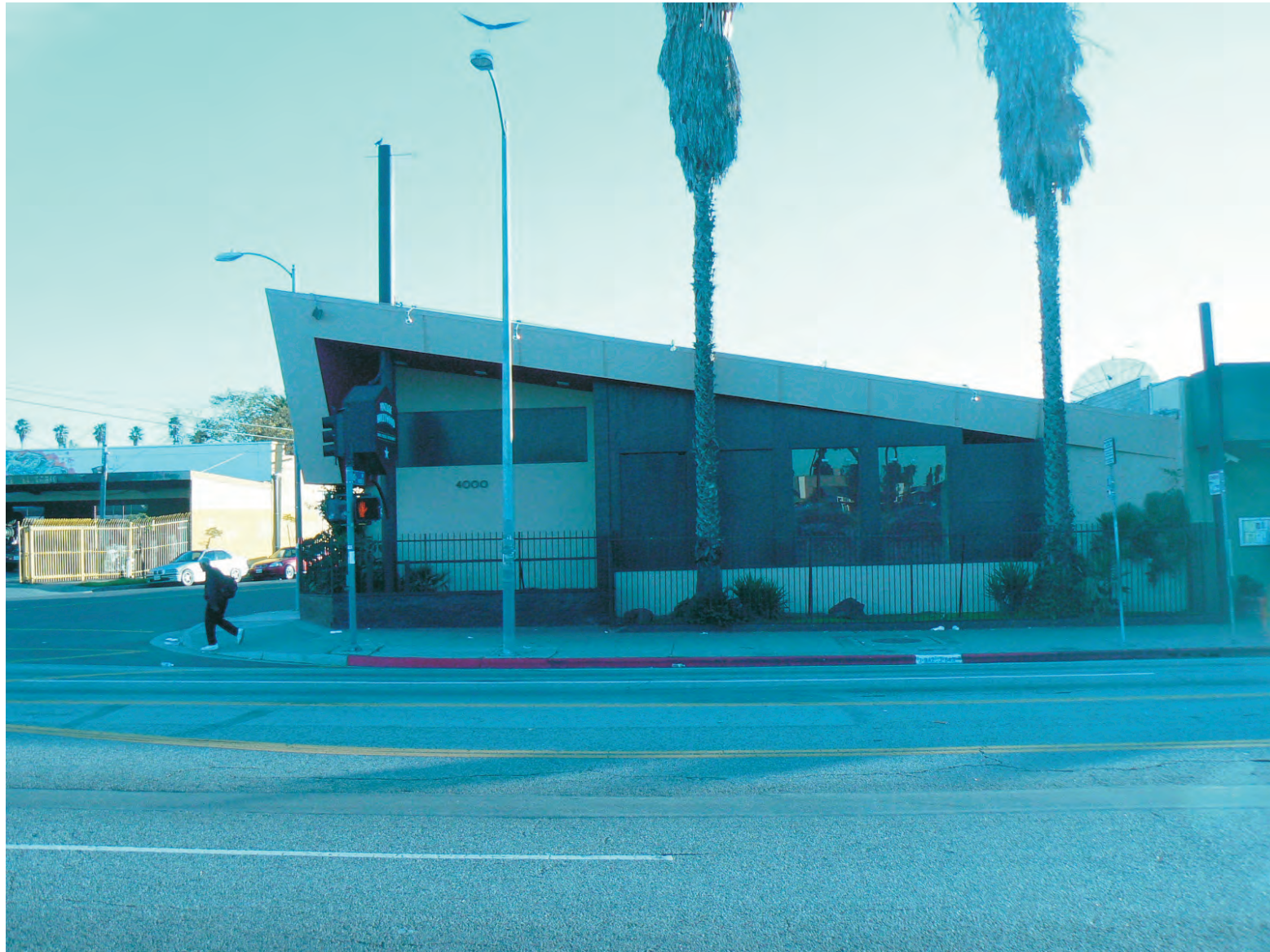
Figure 11 Southwest Corner of W. Washington Boulevard and 10th Avenue View South
