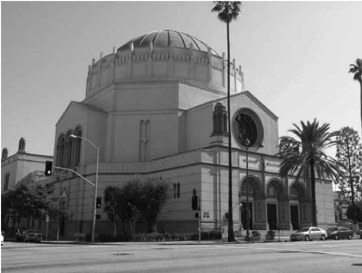
Figure 4.2: Temple Building; Sanctuary
