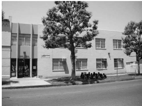
Figure 4.6: Temple Addition, School Building on Harvard Boulevard.
