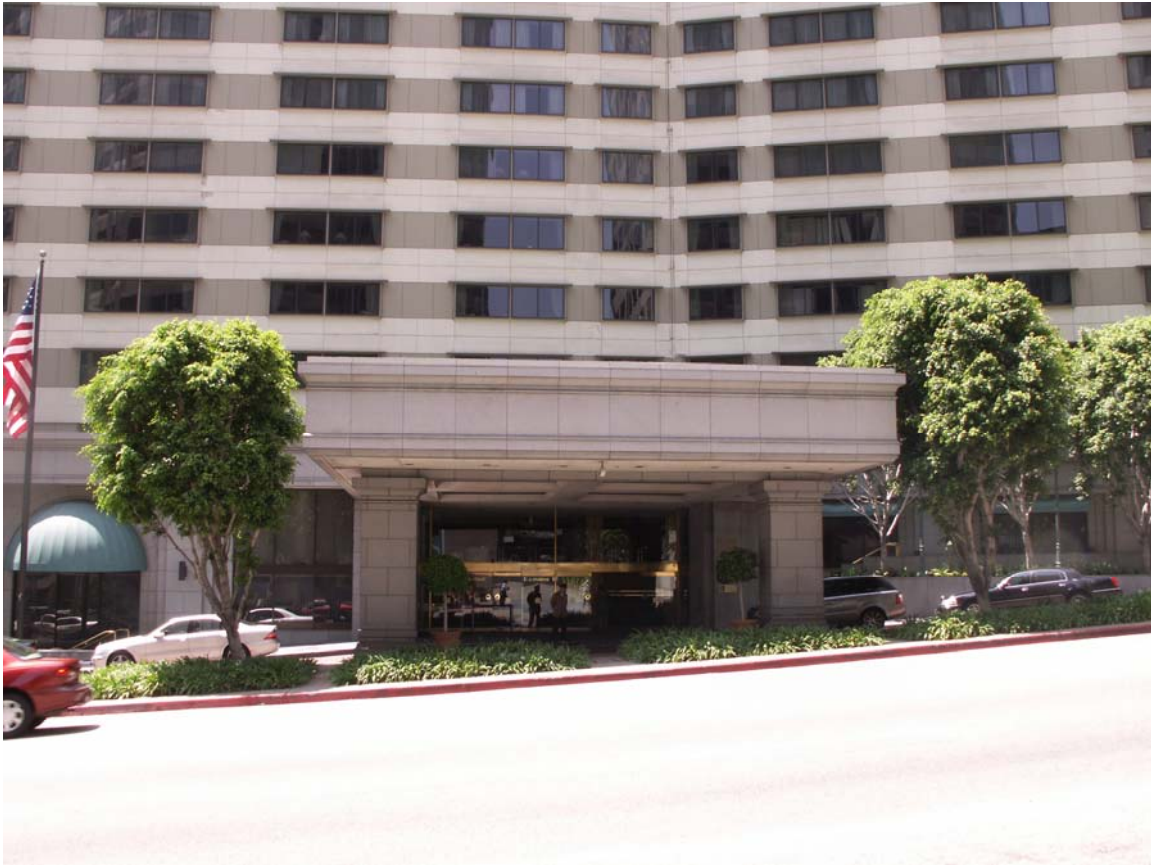
Figure 5: Close-up of New Canopy on North Façade on August 11, 2009
