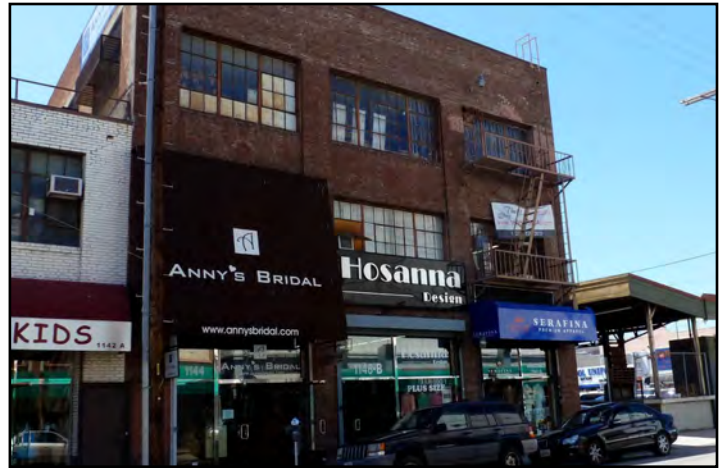
Building 7: 1146 San Julian Street, northwest elevation.
