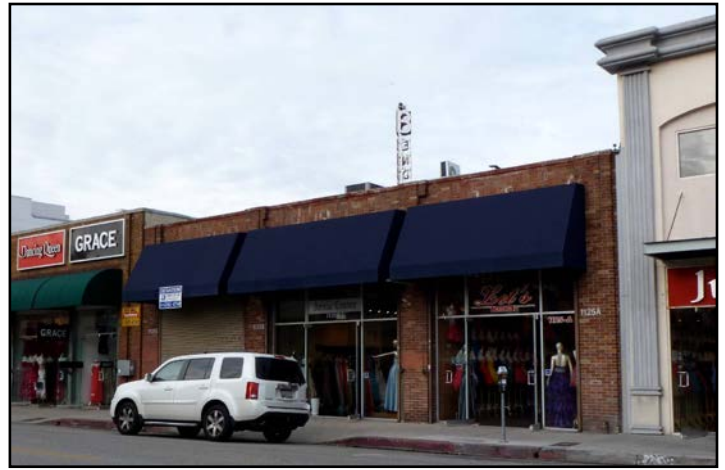
Building 2: 1125 San Julian Street, southeast elevation.
