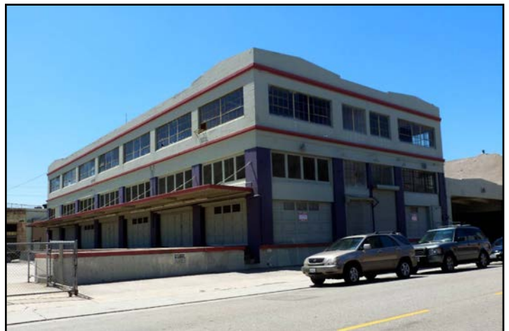
Building 5: 1122 San Julian Street, northwest and northeast elevations.
