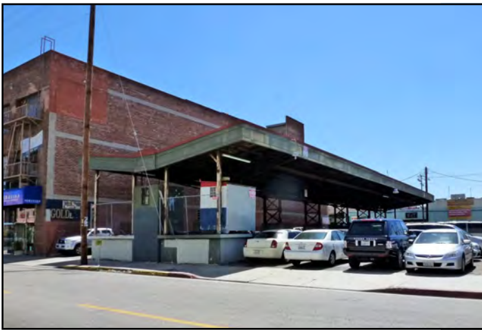
Structure 8: 1150 San Julian Street, northwest and southwest elevations
