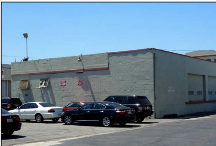
Building 4B: 1102 San Julian Street northeast and northwest elevations.
