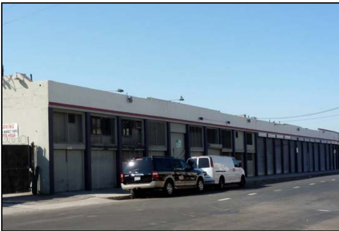
Building 3: 1040-1076 San Julian Street, northwest elevation.
