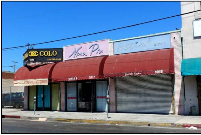
Building 1: 1015 San Julian Street, southeast elevation.
