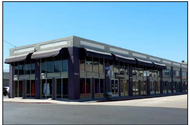
Building 4A: 1102 San Julian Street, northwest elevation.
