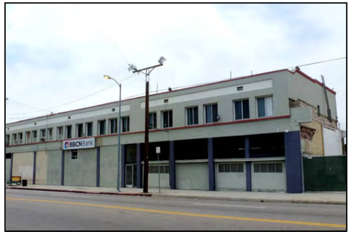
Building 9: 1051-53 South San Pedro Street, southeast elevation.
