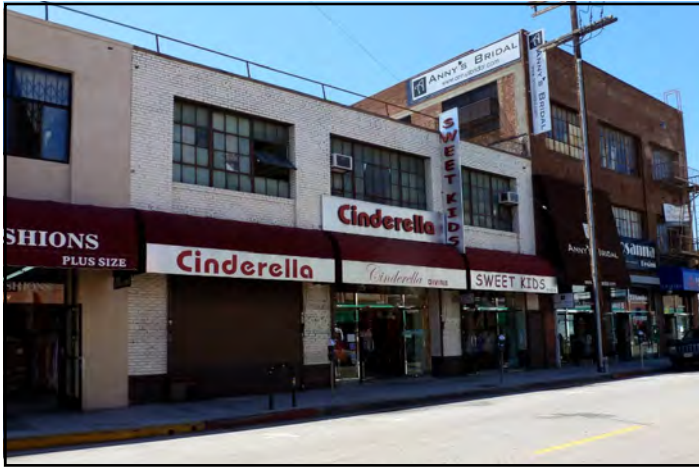
Building 6: 1142 San Julian Street, northwest elevation.
