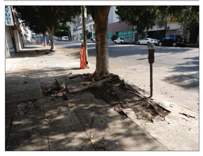
Extensive surface roots from ficus tree no. OS-3 that are causing destructive damage to surrounding sidewalk and city hardscape.
