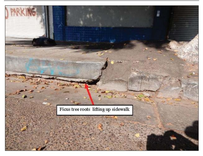
Extensive surface roots from ficus tree no. OS-2 that are causing destructive damage to surrounding sidewalk and city hardscape.
