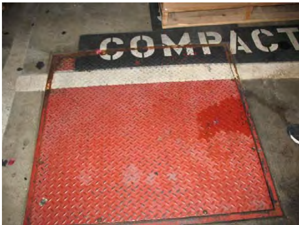
9. View of the access hatch to the sump pump.
