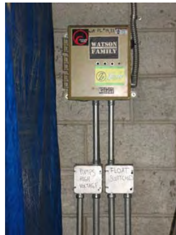
10. View of the sump pump controls observed onsite.
