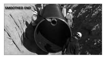
Using forks or unapproved poles inside the pipe will result in damage.
