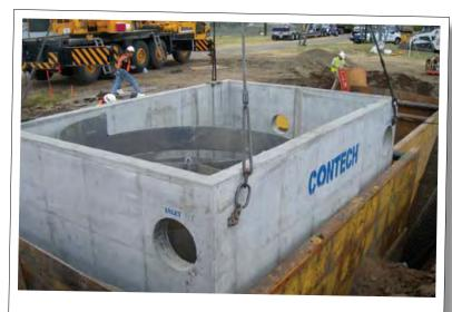
Lage diameter swirl chamber for enhancement of sediment removal in a low profile unit
