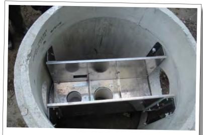
vsHS unique internal bypass design treats high flows and bypasses peak flow, eliminating washout
