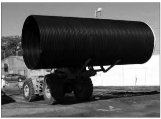
3. Use Nylon lifting slings of sufficient strength and length and specifically intended to safely handle the entire pallet or individual pipe, whichever is being lifted.
