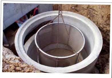
CDS removes fine sediments and trash debris
