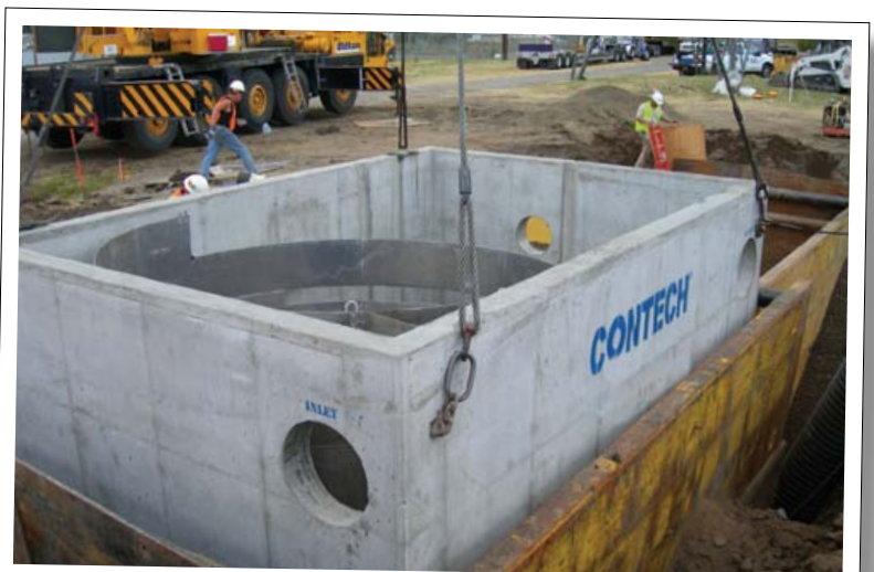
Large diameter swirl chamber for enhancement of sediment removal in a low profile unit
