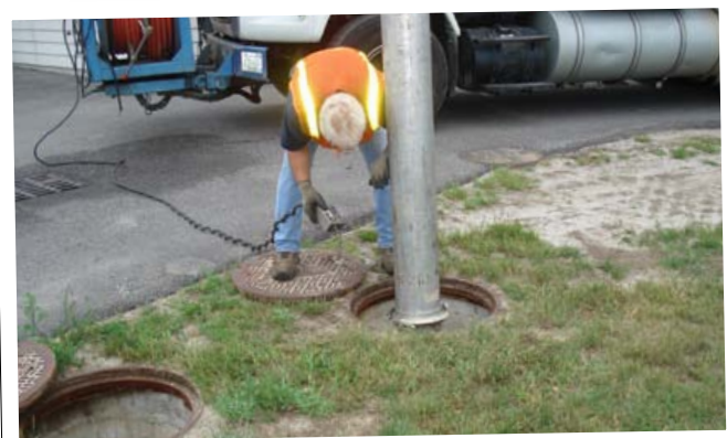
A CDS unit can be easily cleaned out in less than 30 minutes
