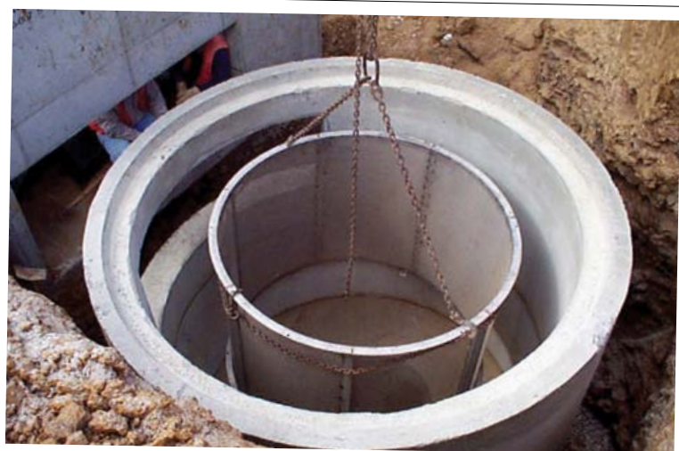
CDS removes fine sediments and trash debris
