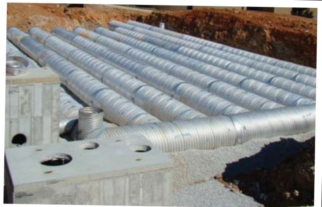
A Vortechs protects detention system from sediment build-up and reduces maintenance
