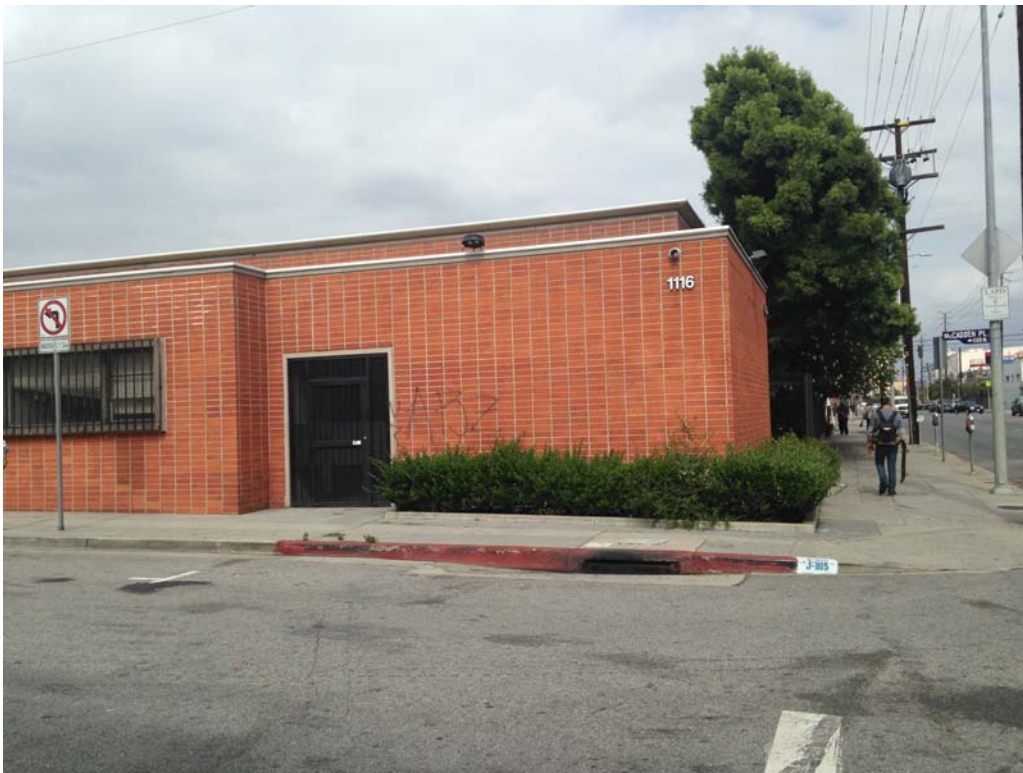
View of the southwest corner of the subject property office building looking E 1116 N McCadden Place & 6725 Santa Monica Blvd, Los Angeles
