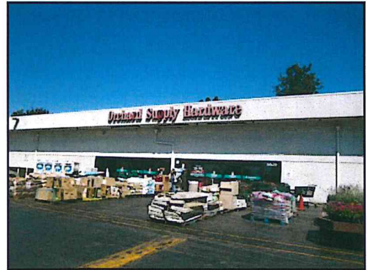
2 : Front entrance to the site building
