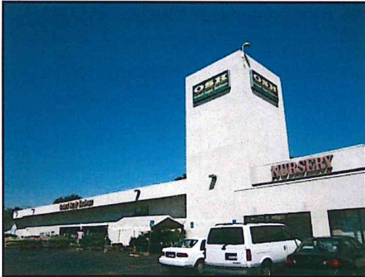
1 : Front (southern) facade of the site building
