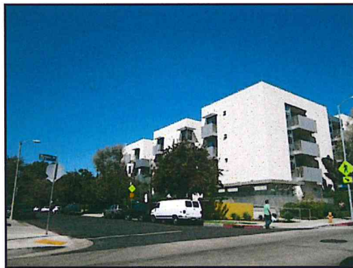
17 : North adjacent apartment building
