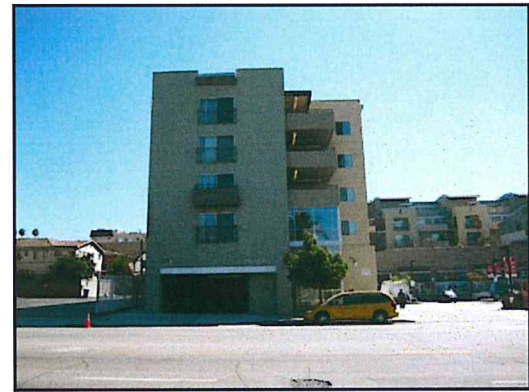
18 : East adjacent retail center and apartments
