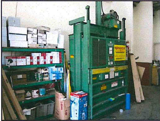
13 : Box bailer in rear utility area
