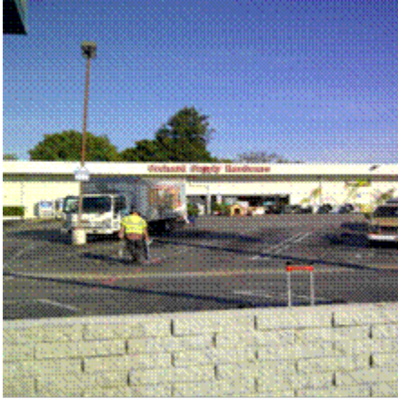
Photo #1: Front of building
