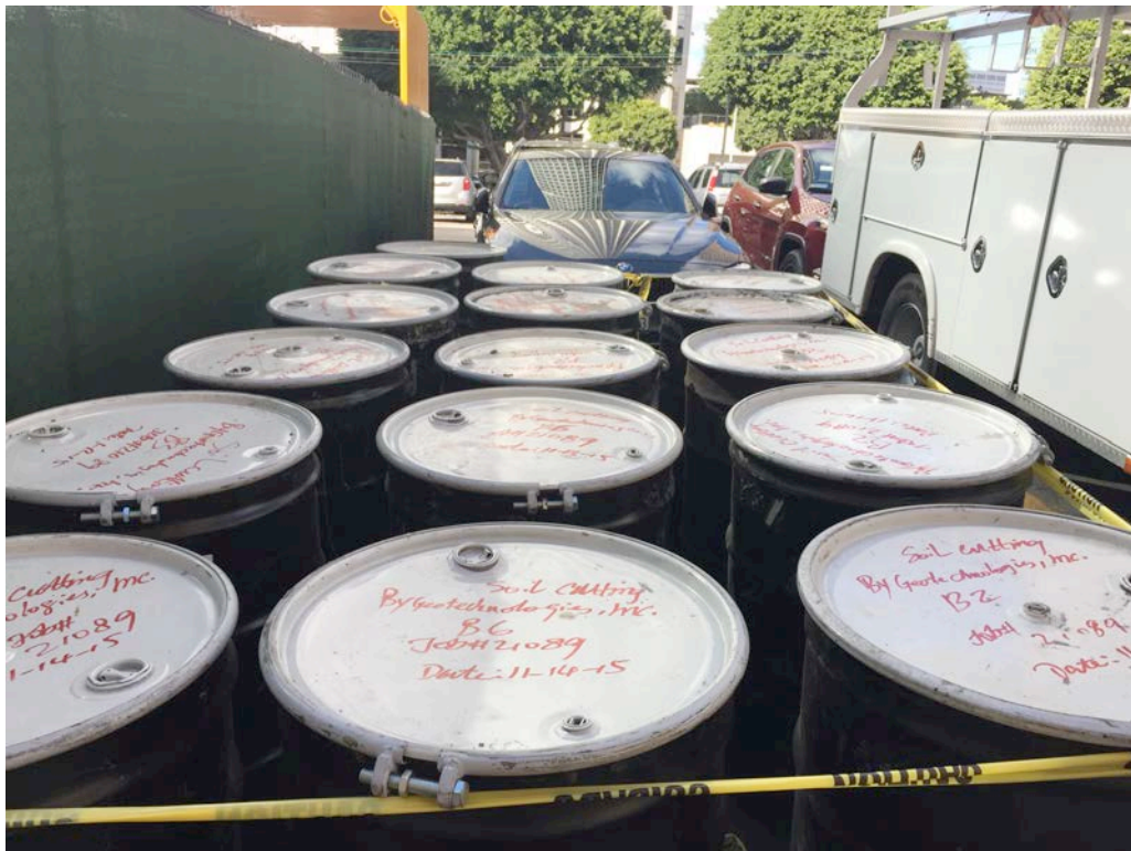
Soil cuttings storage on the southern edge of the property Figueroa Street & W 8 th Street, Los Angeles, CA 94105
