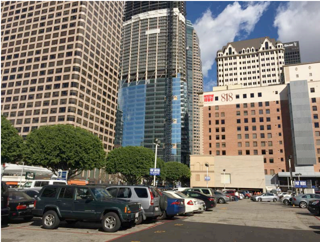
Southwest portion of the subject property; view to the north Figueroa Street & W 8 th Street, Los Angeles, CA 94105
