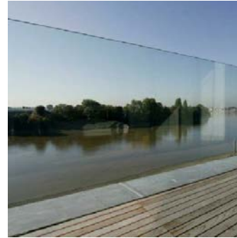
GLAZING #3: TEMPERED GLASS GUARDRAIL, LOW REFLECTIVE
