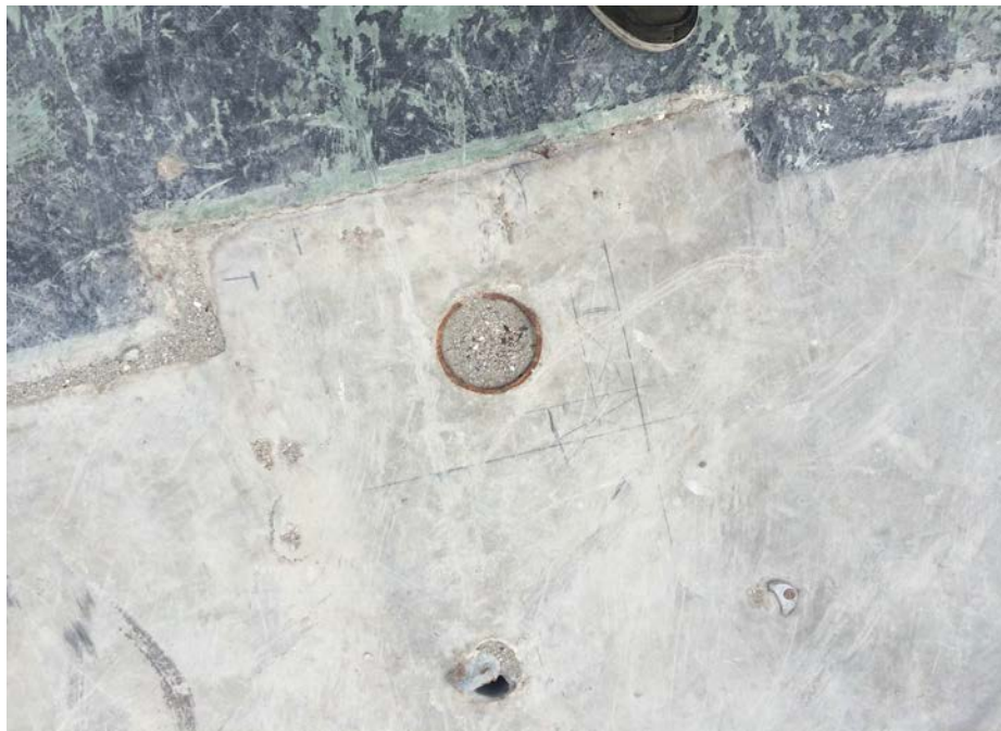
Photo 11 – View of remnant pipe stubs observed on the subject property.
