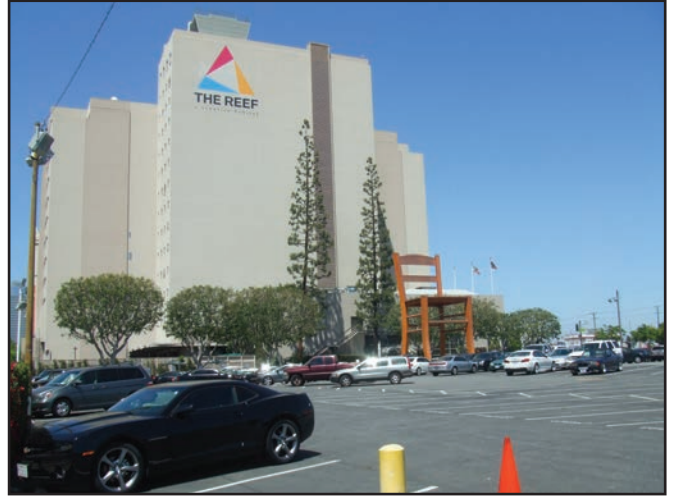
View 2: View of The Reef building from Hill Street with West Block parking lot in foreground.
