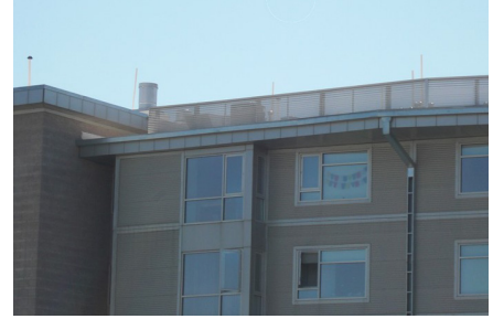
Metal screens could be utilized to hide utilities located on the rooftop. (Figure A.4.l)
