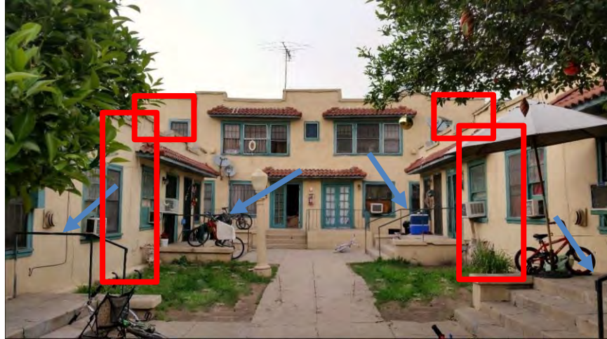
Figure 10 4059-4065 Oakwood Avenue with red boxes showing additions and blue arrows pointing out added metal railings on porches
