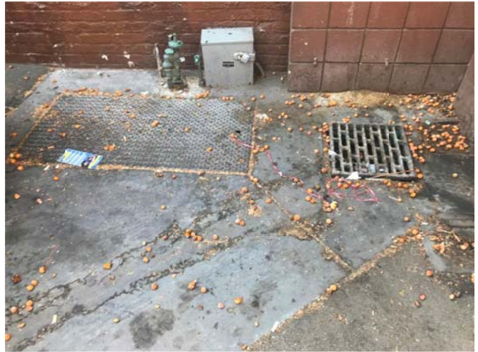
32. View of an area drain at the Site.
