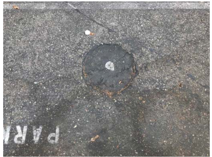
34. View of a patched boring at the Site.
