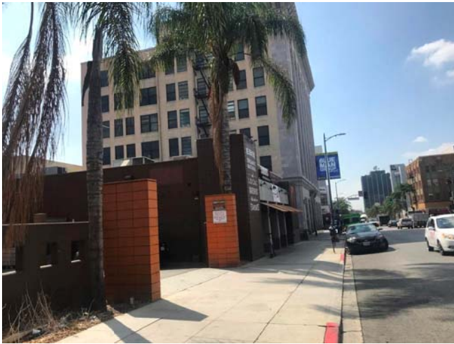
1. View southeast of the 1716 and 6381 buildings.
