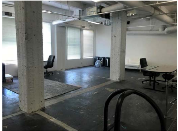
14. Typical vacant office space at the 6381 building.
