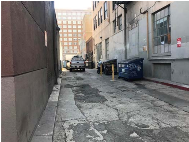
33. View of the alley and dumpsters between the 6381 and 1716 buildings.
