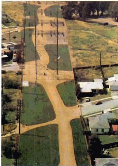
Multiple Use of Open Space
