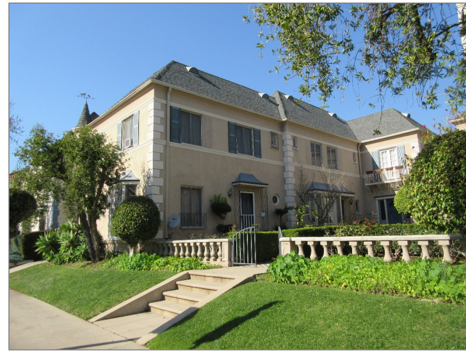
2 stories, portion of building along street
