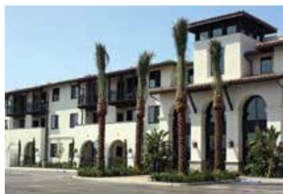
Dana Strand Phase III - Senior Apartments
