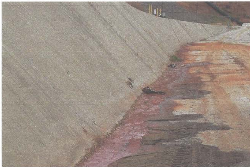
Photo 4: Water flowing out between floor slab and wall joints at Terminal basin
