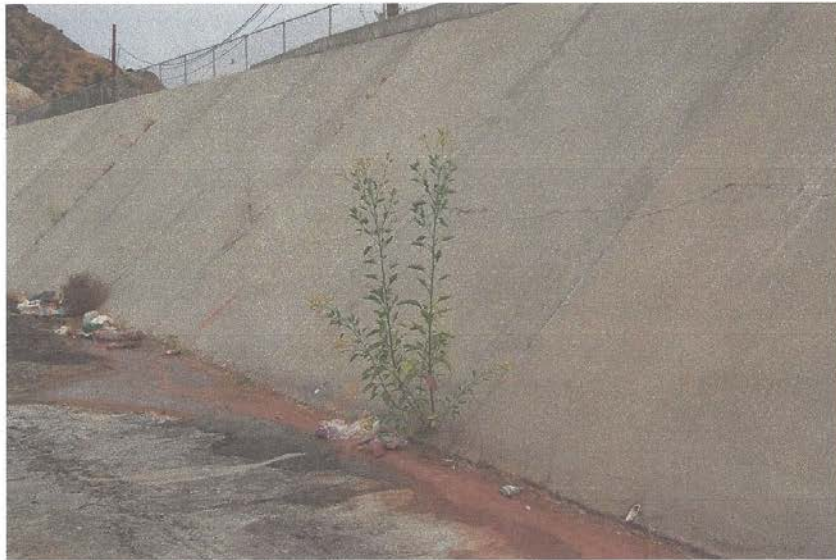
Photo 7: Vegetation growing in weep hole and cracks of Terminal basin wall
