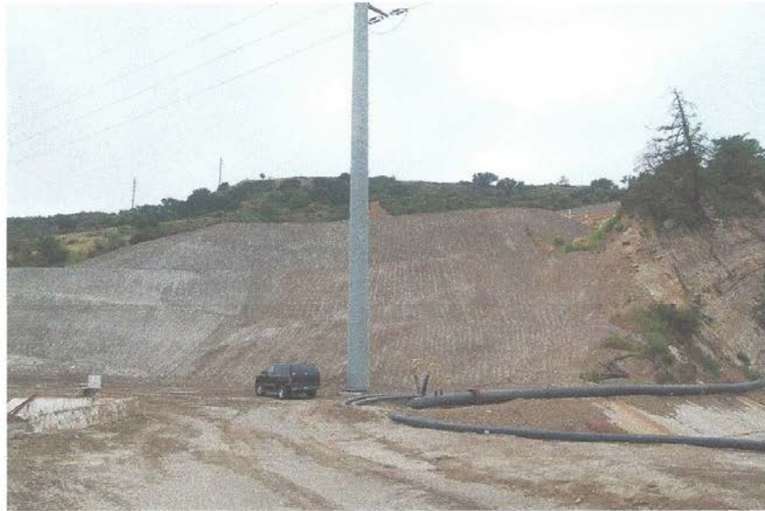
Photo 13: Reworked slopes beneath Flare 3 and near Basin A
