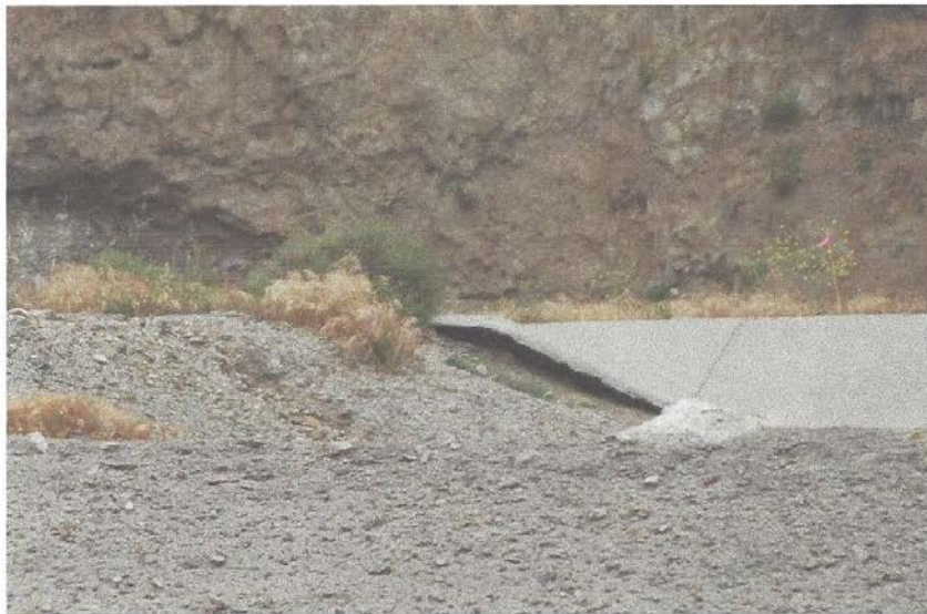
Photo 10: Undermined shotcrete spillway at Basin D
