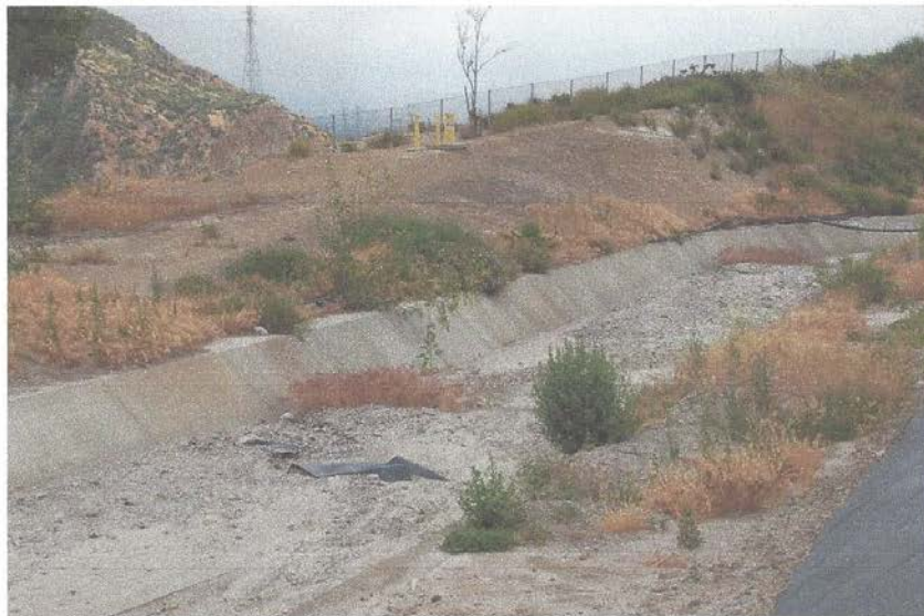
Photo 8: Vegetation, sediments, and detritus in channel between Basin B and Terminal Basin
