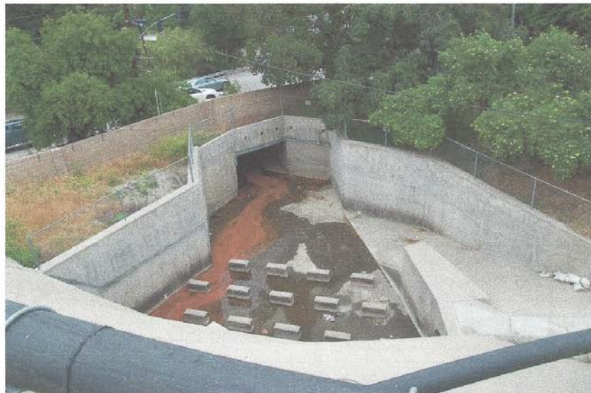
Photo 6: Reddish water leaving the landfill
