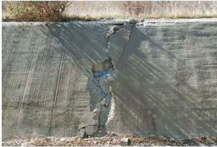
Photo 5: V Spalling and falling concrete on channel between Basin A and Basin D
