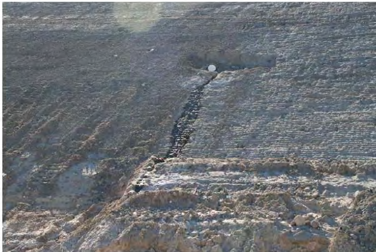
Photo 2: Erosion gully on slope
