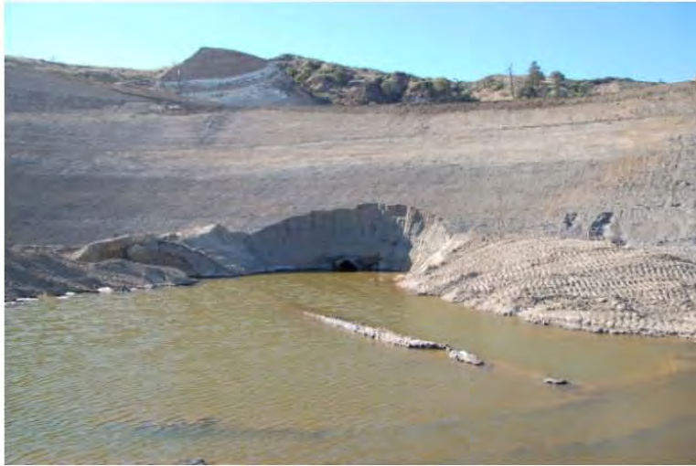
Photo 1: Seep and ponding water at toe of vertical cut under slope
