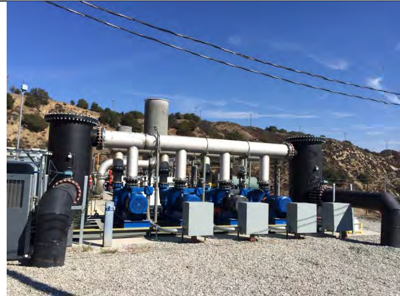
Photo 62: Flare 9 and 10 Inlet Gas Blowers: February 5, 2014
