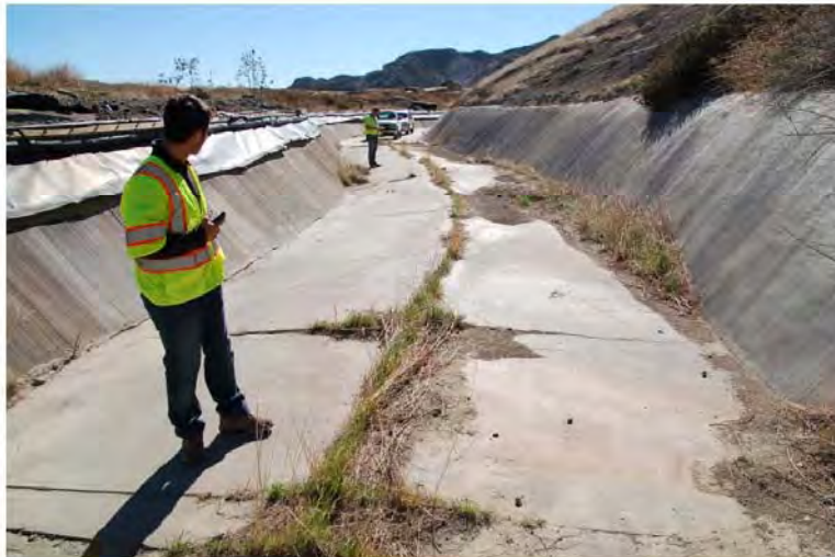
Photo 3: Cracked and uplifted bottom of concrete channel between Basin A and Basin D
