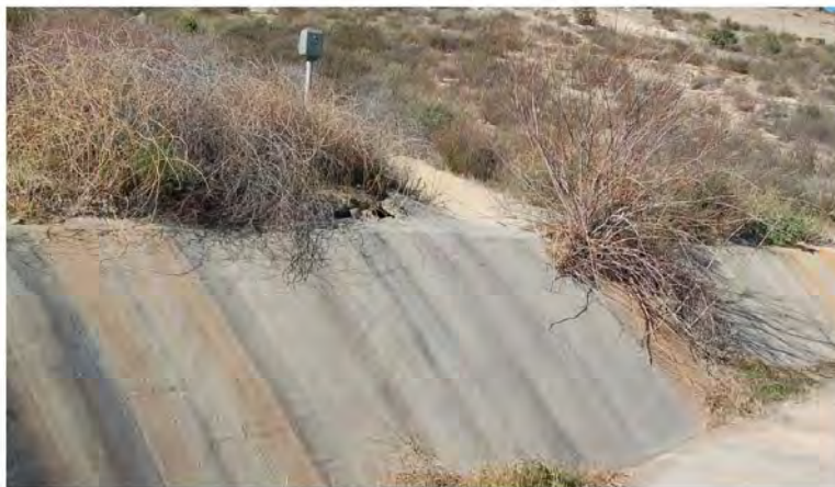
Photo 4: V ditch feeding the channel – Note gap between shotcrete and soil at connection V-ditch channel
