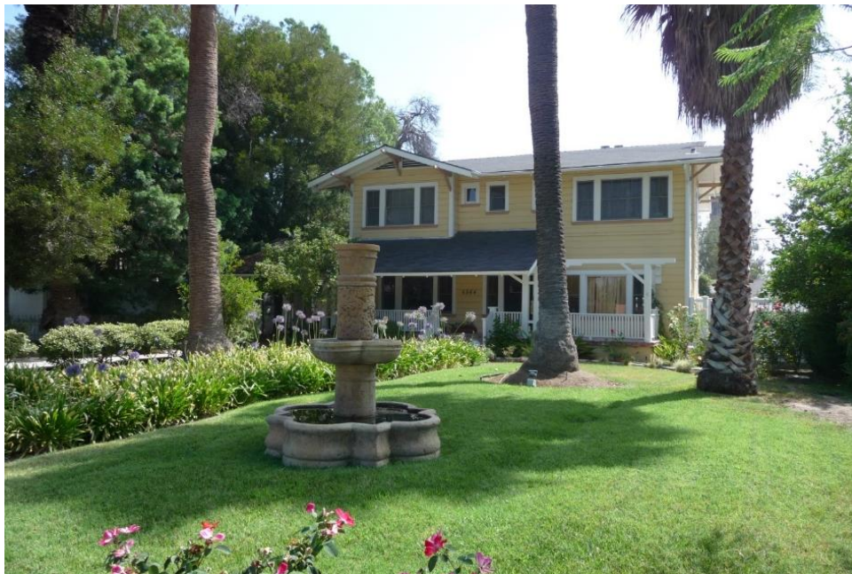
Craftsman House, 1914 6964 N. Shoup Avenue, West Hills (SurveyLA)
