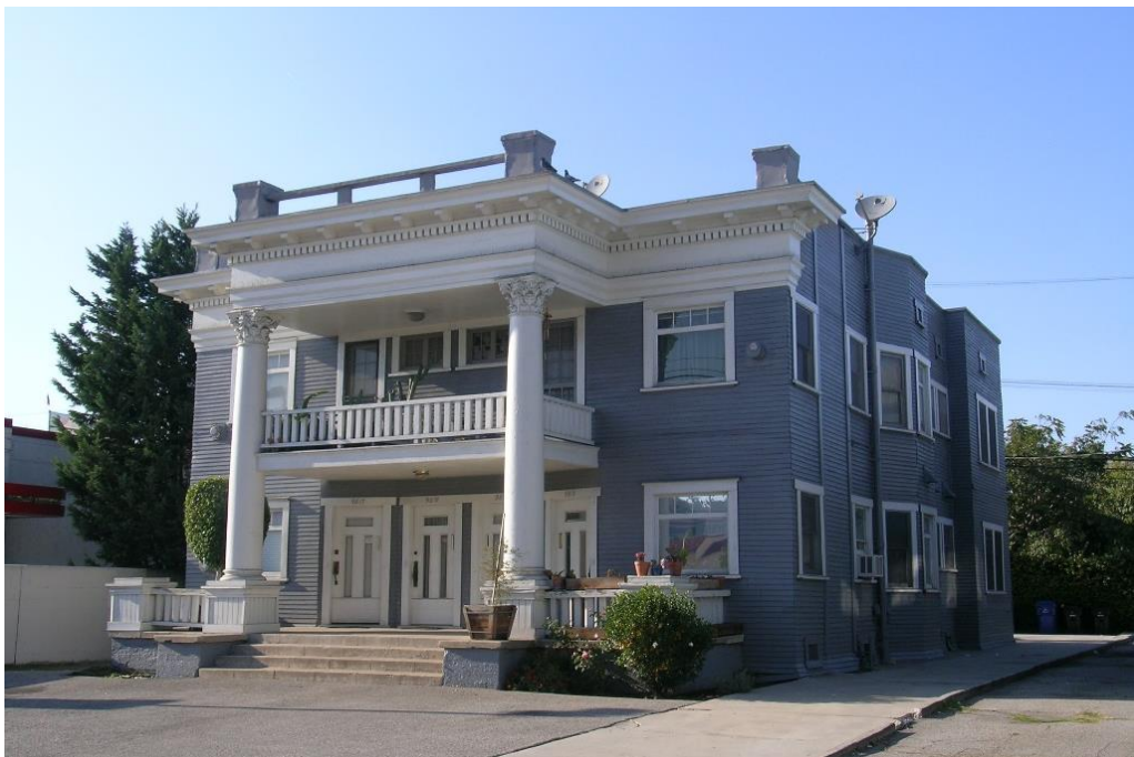
Neoclassical Apartment House, 1915 9813-19 W. Venice Blvd., Palms (SurveyLA)
