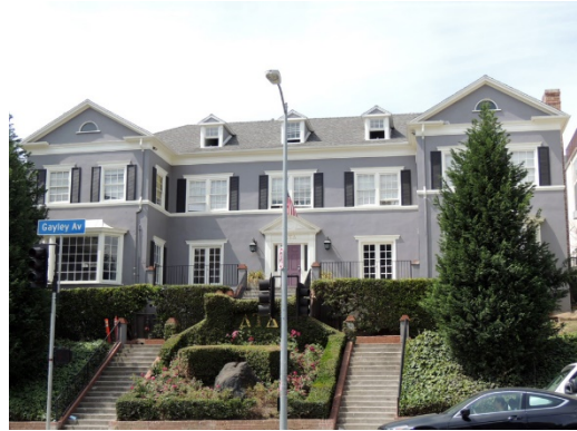
Address: 649 S. Gayley Avenue Name: Delta Tau Delta Fraternity House Architect: G.G. McAllister Date: 1939
