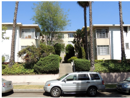
Address: 670 S. Kelton Avenue Date: 1951
