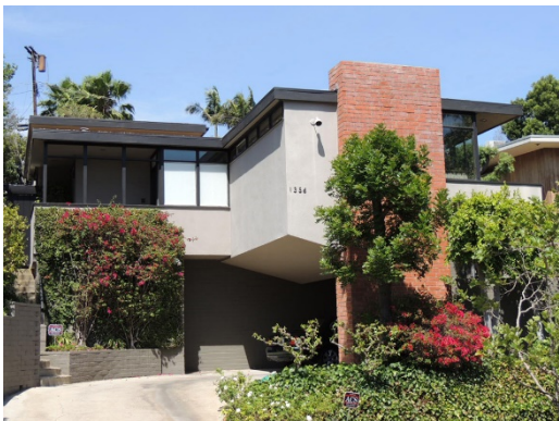
Address: 1356 S. Comstock Avenue Architect: Morris D. Verger Date: 1953
