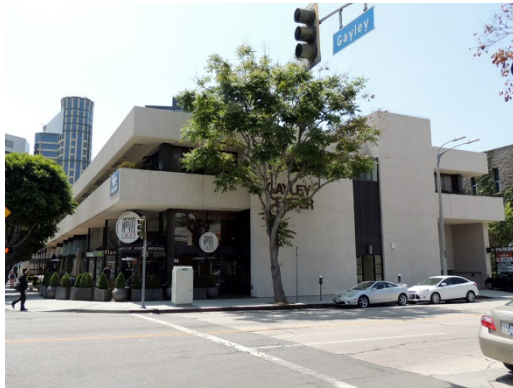
Address: 1101 S. Gayley Avenue Name: Gayley Center Architect: Krisel-Shapiro & Assoc. Date: 1979
