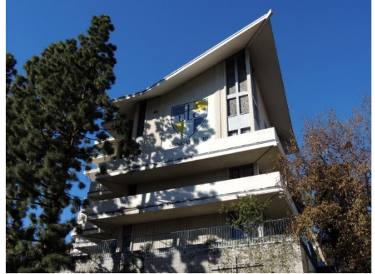
Address: 10915 Strathmore Drive Name: University Lutheran Chapel Architect: Wilkes & Steinbrueck Date: 1965
