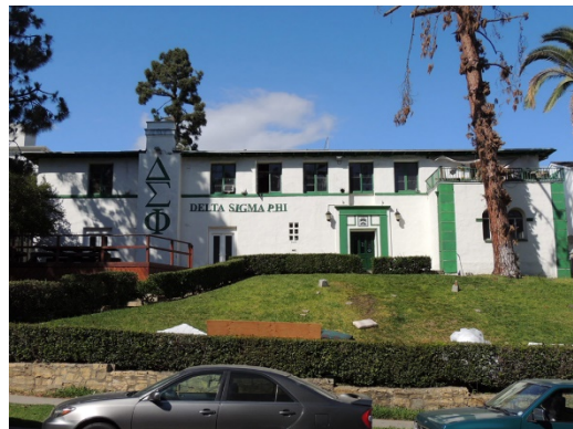
Address: 620 S. Landfair Avenue Name: Delta Sigma Phi Fraternity House Architect: Milton J. Black Date: 1930
