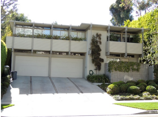
Address: 1001 S. Westholme Avenue Architect: Richard K. Fleming (for Buff & Hensmen) Date: 1966
