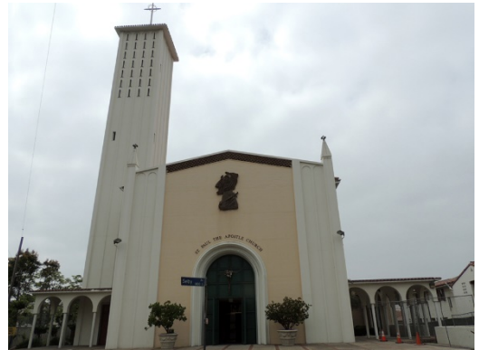
Address: 10750 Ohio Avenue Name: St. Paul the Apostle, Main Church Architect: Chaix & Johnson Date: 1958
