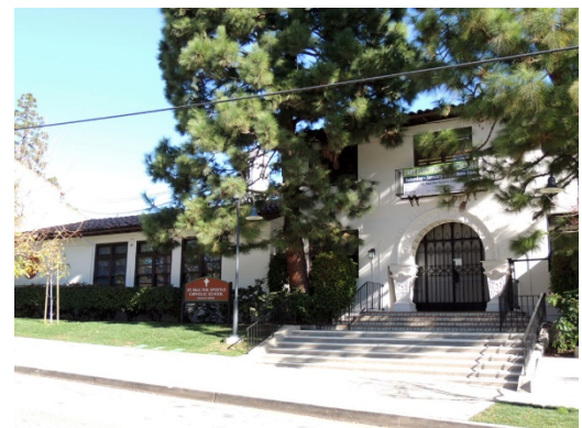
Address: 10750 Ohio Avenue Name: St. Paul the Apostle, School Date: 1935
