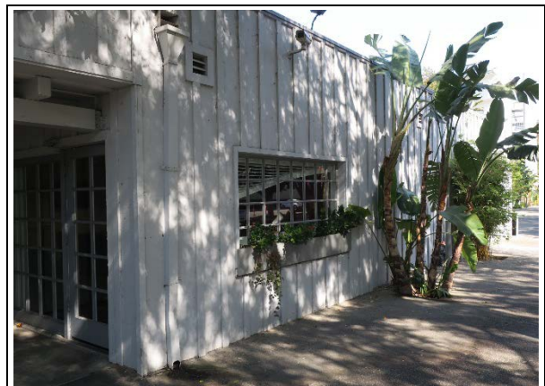
Detail of east elevation, view northwest. The one-story volume is an addition. Note channel siding and wood frame windows (ARG, 2020)
