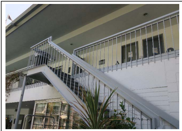
East elevation, detail of cantilevered balcony, staircase, and metal balustrade (ARG, 2020)
