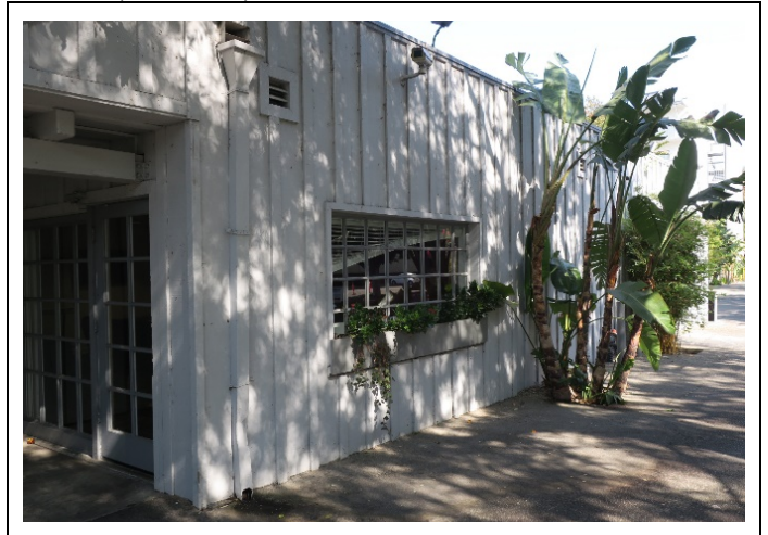
Image 7. Detail of east façade, view northwest (ARG, 2020)
