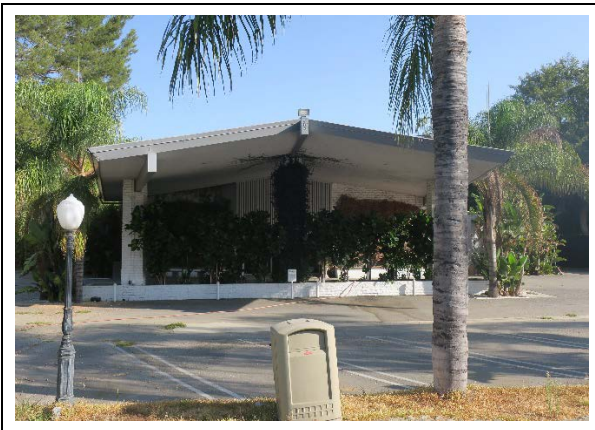
Porte cochere on primary (south) façade, view north. Note post-and-beam details (ARG, 2020)
