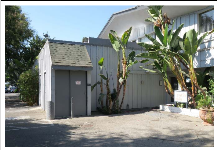
Image 6. Detail of east façade, view southwest (ARG, 2020)
