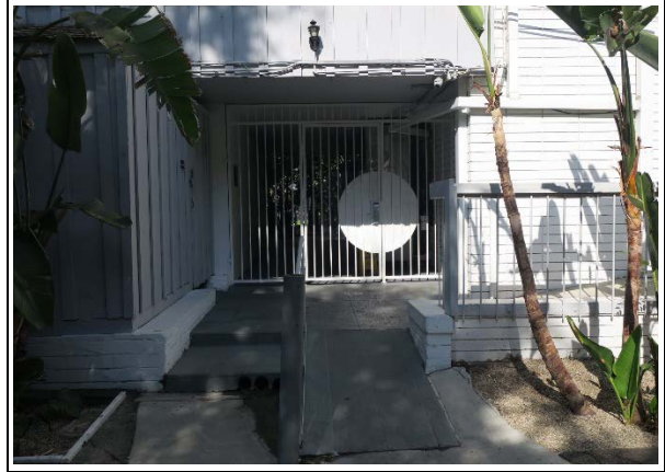
East elevation, detail of breezeway and security gate, view west (ARG, 2020)
