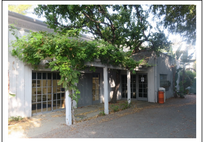
Image 5. East façade, view northwest. The one-story volume is an addition (ARG, 2020)
