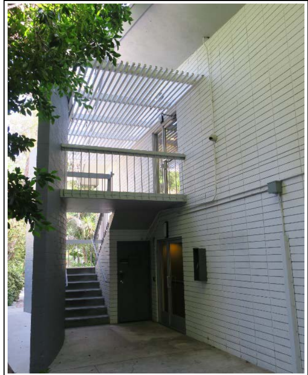
West elevation, detail of exterior stairwell, concave concrete block wall, and overhead wood trellis, view northeast (ARG, 2020)
