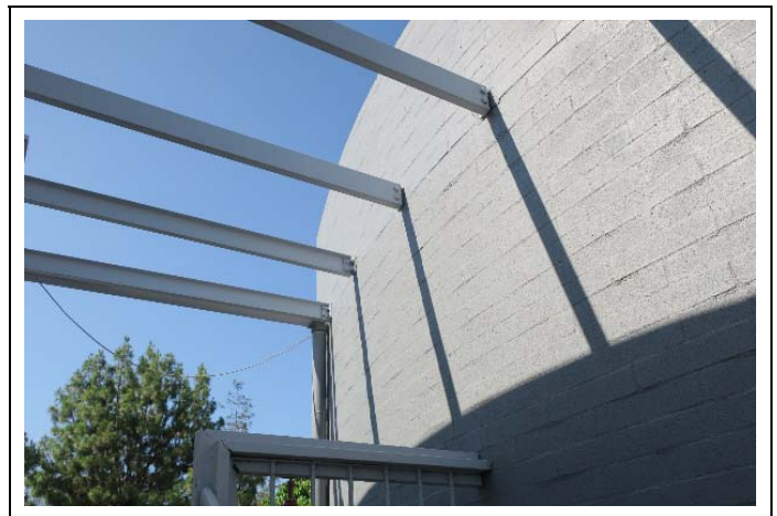
Image 13. Detail of interior courtyard, view east (ARG, 2019)
