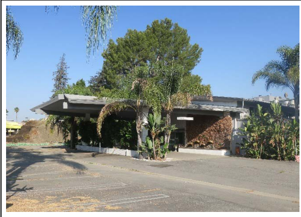
Primary (south) façade and porte cochere, view northwest (ARG, 2020)
