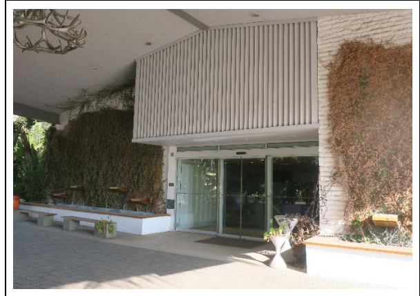
Primary façade and balcony, set within porte cochere, view northwest (ARG, 2020)
