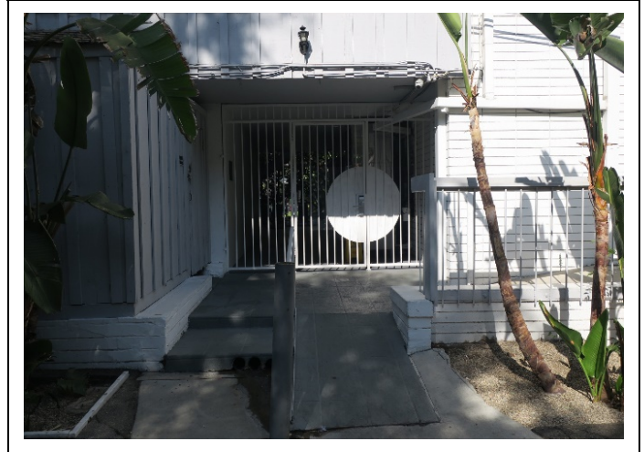
Image 9. East façade, detail of breezeway and security gate, view west (ARG, 2020)
