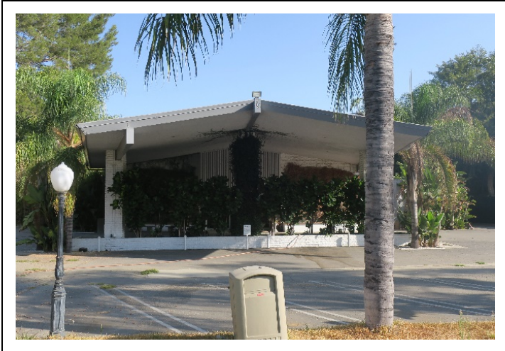
Image 4. Porte cochere on primary/south façade, view north. Note post-and-beam details (ARG, 2020)
