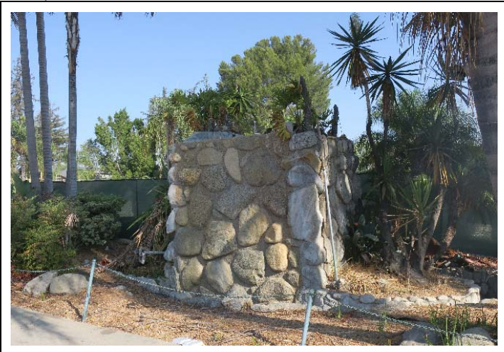
Image 22. Detail of stone wall, view northwest (ARG, 2020)
