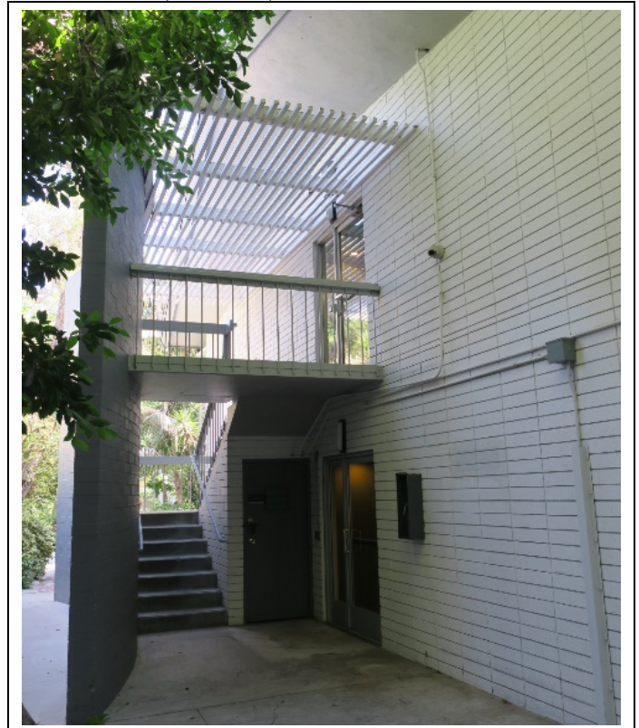
Image 17. West façade, detail of exterior stairwell, concave concrete block wall, and trellis, view northeast (ARG, 2020)
