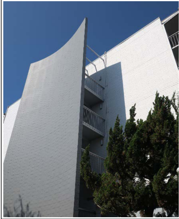
East elevation, detail of exterior stairwell and concave concrete block wall, view southwest (ARG, 2020)
