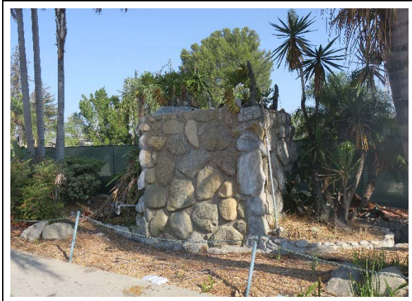
Detail of stone hardscape features at front (south) end of property, view northwest (ARG, 2020)
