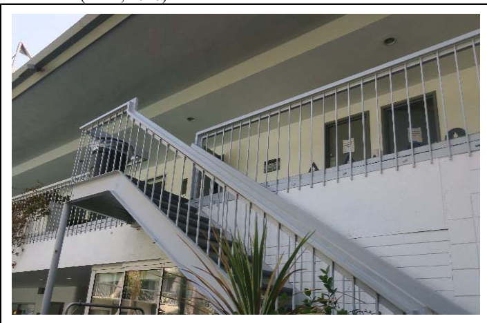
Image 12. Detail of interior courtyard, view east (ARG, 2019)
