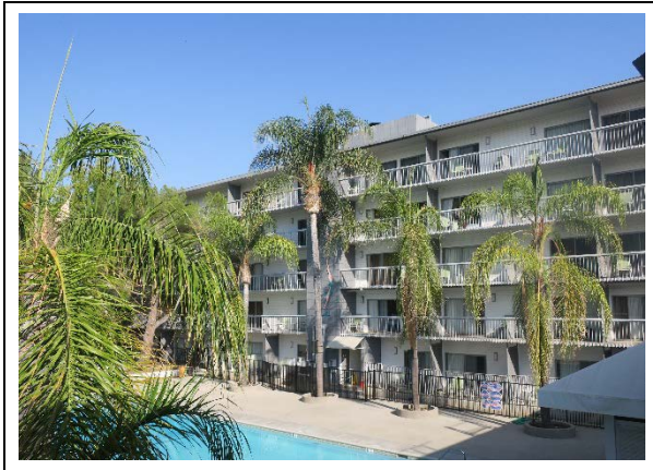
North (5-story) wing as seen from courtyard, view northwest (ARG, 2020)
