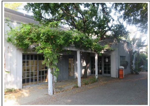
East elevation, view northwest. The one-story volume is an addition (ARG, 2020)
