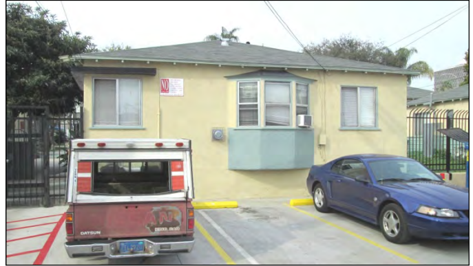
Typical east elevation, view to the west.
