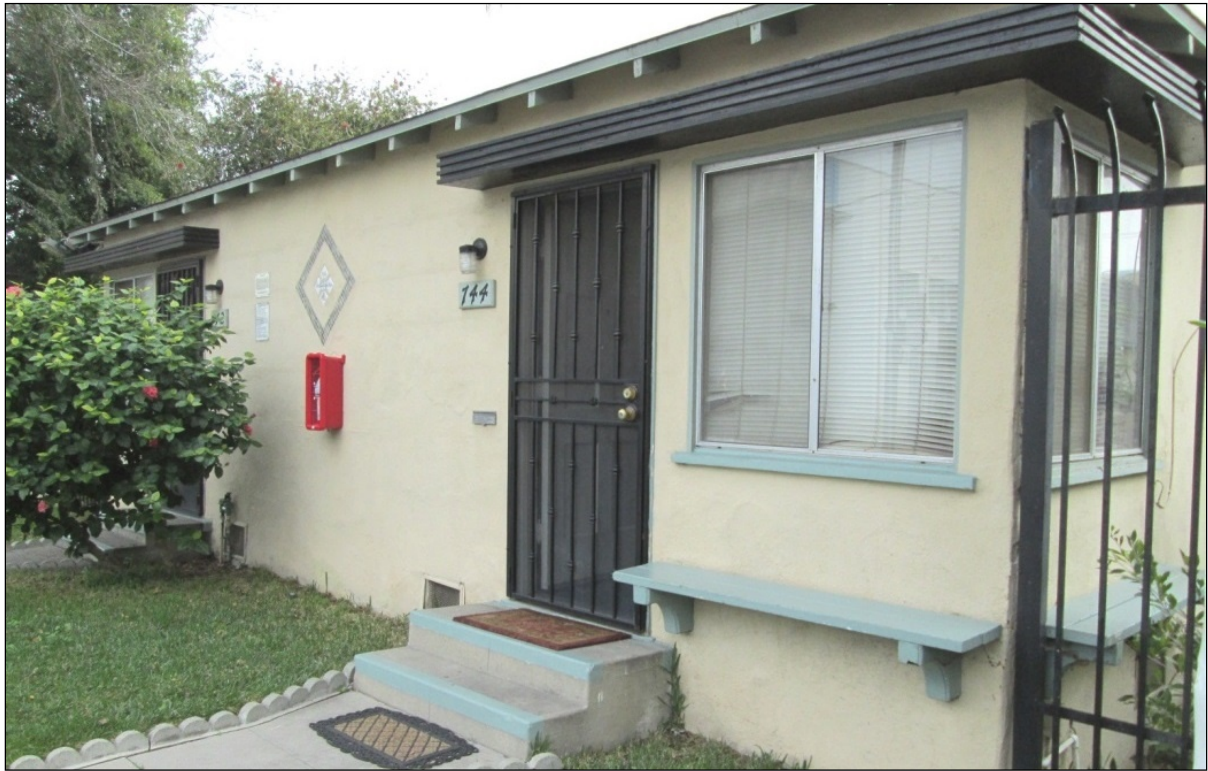
Figure 6: 744 South Grand View Street. Close up of wrap around “coping”. Note non-original tile accents and windows (view to the northeast, 1/18/17).
