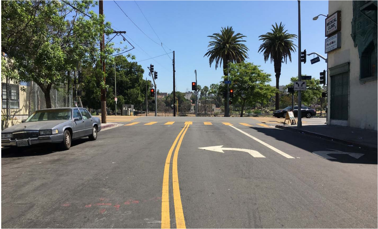
5. Condition of Grand View St., facing north towards 7 th St.
