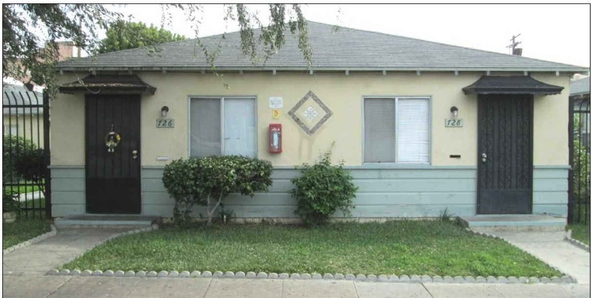
Figure 7: 726-728 South Grand View Street. Typical façade of the 12 duplexes flanking the 6 center duplexes. Note non-original windows and tile accent (view to the east, 1/81/17)
