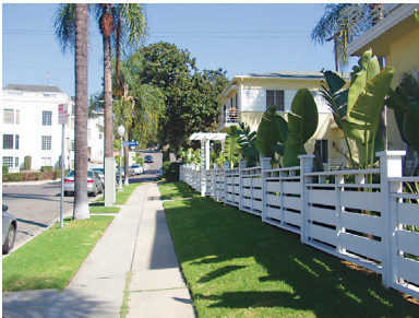
Historic forms that influence character extend from buildings to streetscapes
