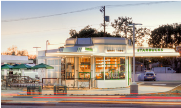
Gilmore Gas Station after
