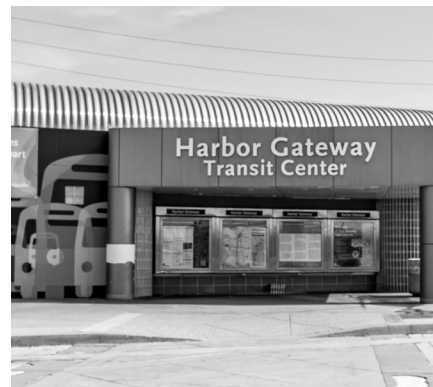
Harbor Gateway Transit Center
