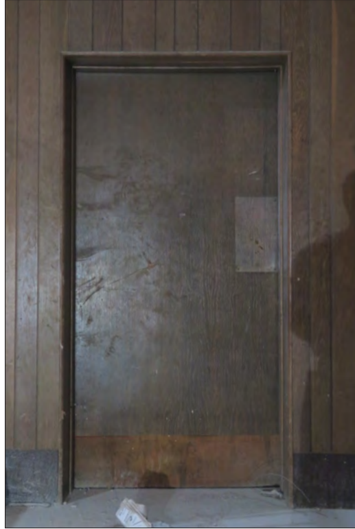
Image 30: Subject property, basement, detail of elevator door, view north (Chattel, 2019)
