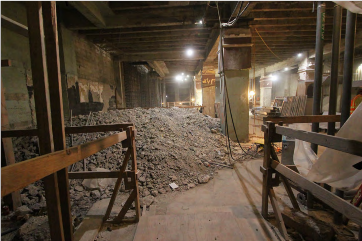
Image 25: Subject property, basement, view northwest (Chattel, 2019)
