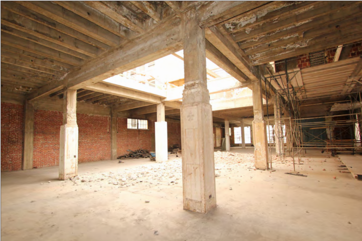
Image 116: Subject property, floor 6, view west (Chattel, 2019)
