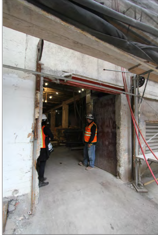
Image 9: Subject property, east elevation, entryway at rear, view northwest (Chattel, 2019)
