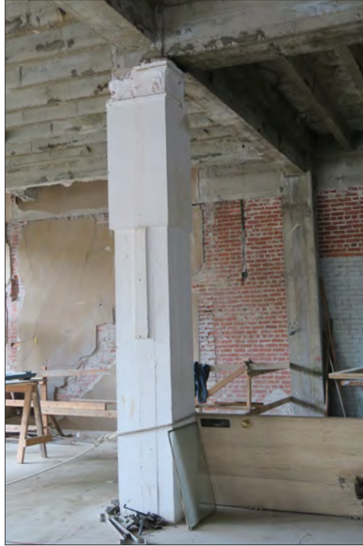
Image 100: Subject property, floor 5, column (Chattel, 2019)
