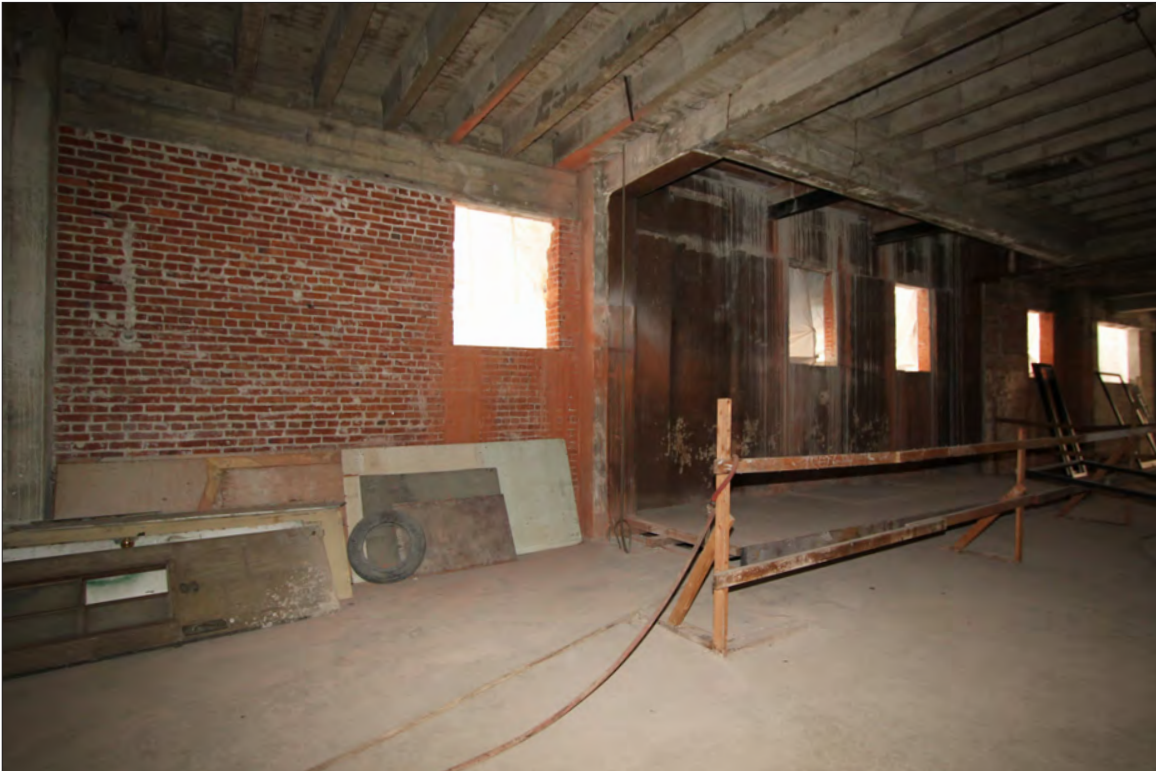
Image 69: Subject property, floor 3, view west (Chattel, 2019)
