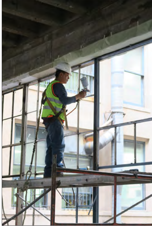
Image 84: Subject property, floor 4, construction work at steel windows (Chattel, 2019)
