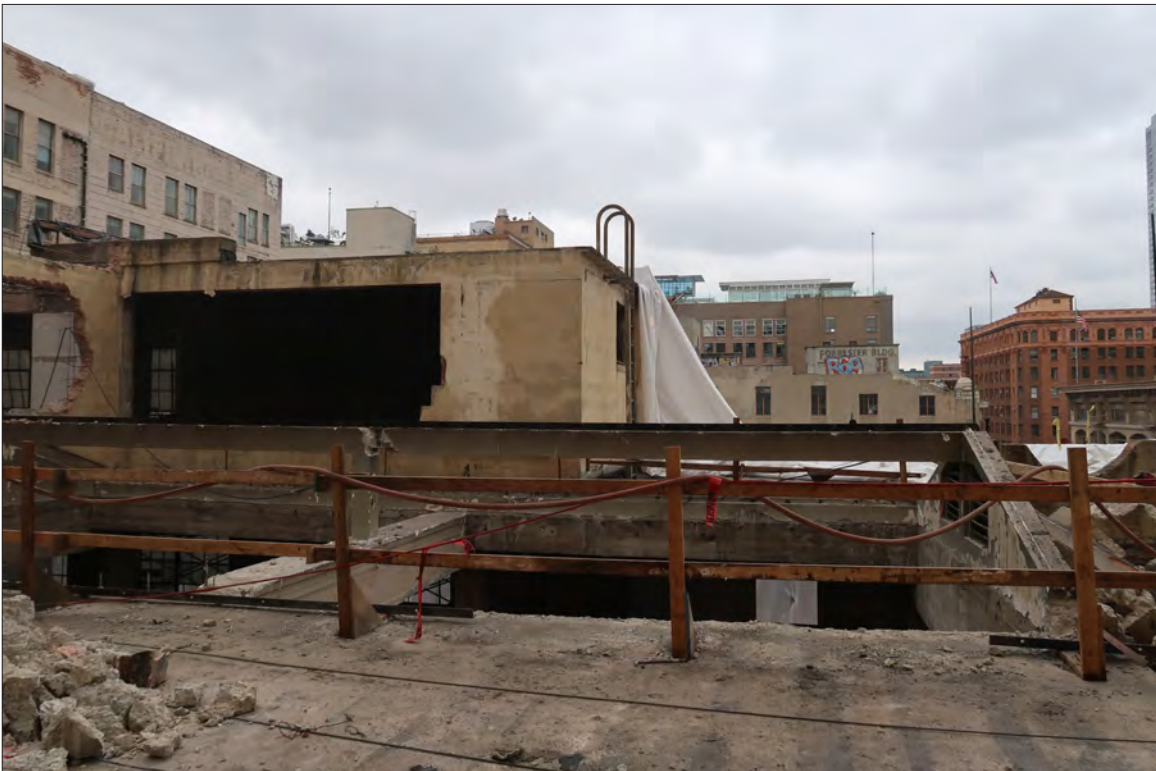
Image 141: Subject property, roof, view southwest (Chattel, 2019)
