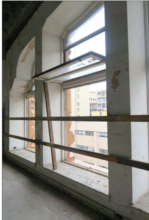
Image 126: Subject property, floor 6, windows at west elevation, view west (Chattel, 2019)
