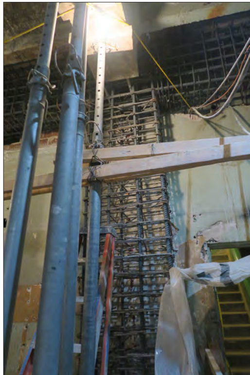
Image 37: Subject property, basement, work on moment frame (Chattel, 2019)
