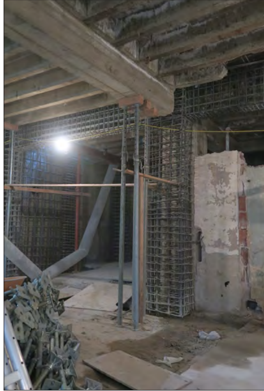
Image 36: Subject property, basement, work on moment frame (Chattel, 2019)
