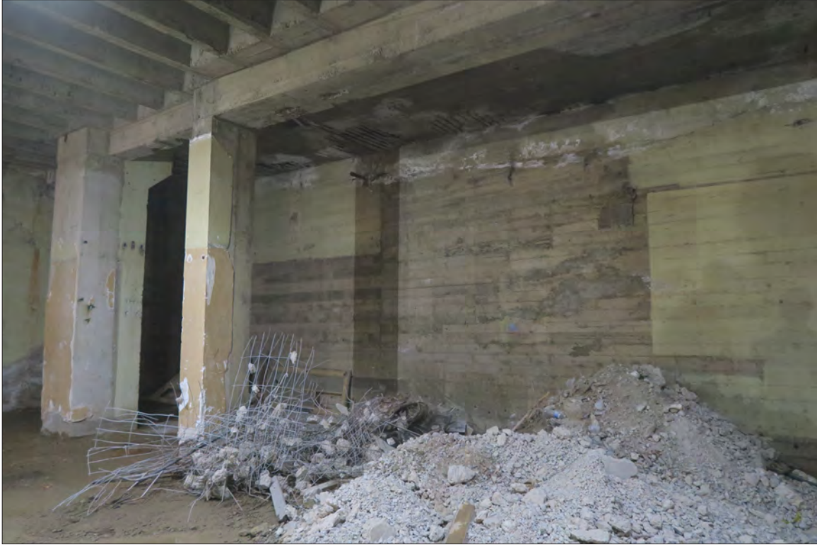
Image 38: Subject property, basement, view north (Chattel, 2019)
