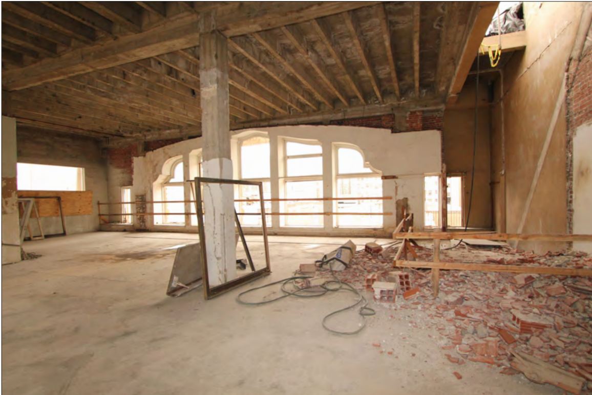
Image 123: Subject property, floor 6, view west (Chattel, 2019)
