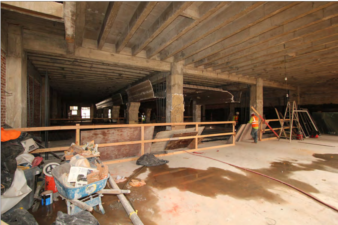
Image 51: Subject property, floor 2, view north (Chattel, 2019)
