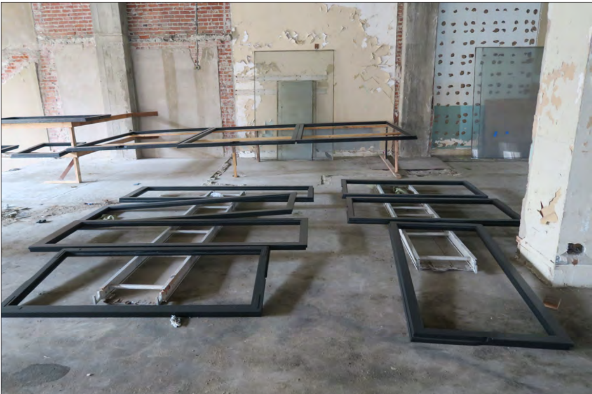
Image 83: Subject property, floor 4, restored window sashes (Chattel, 2019)
