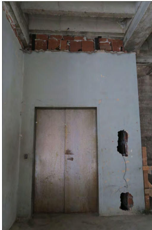
Image 91: Subject property, floor 5, elevator , view southwest (Chattel, 2019)
