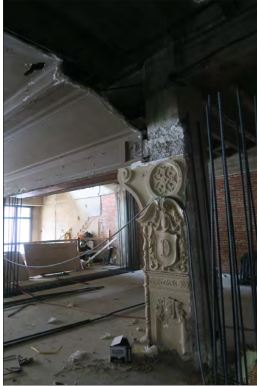
Image 54: Subject property, floor 2, detail of mezzanine column, view north (Chattel, 2019)
