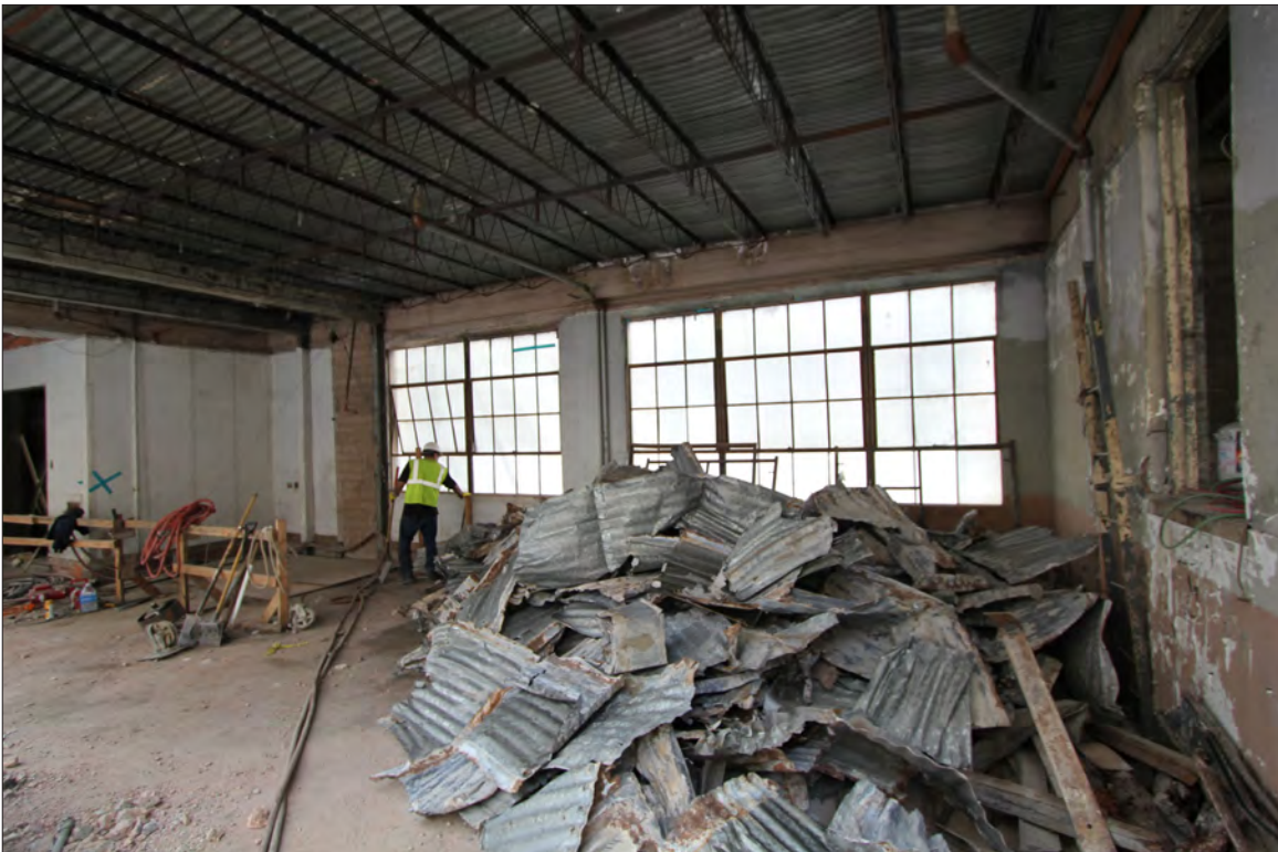
Image 137: Subject property, roof, view south (Chattel, 2019)
