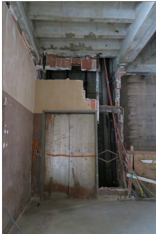
Image 67: Subject property, floor 3, elevator , view southwest (Chattel, 2019)
