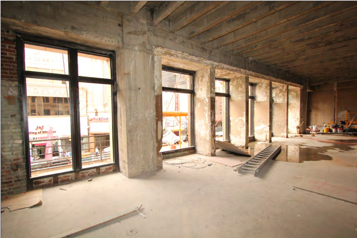
Image 59: Subject property, floor 2, windows at west elevation, view north (Chattel, 2019)
