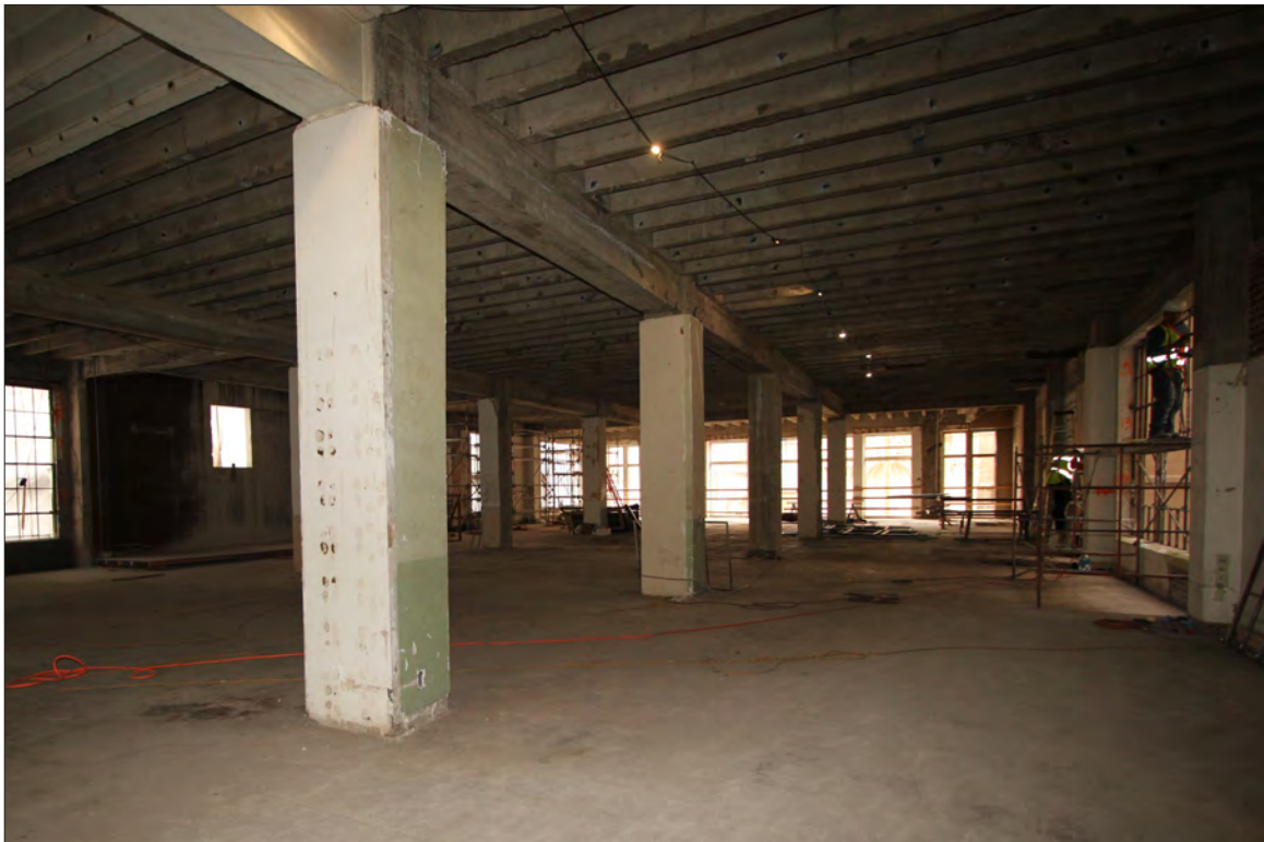
Image 81: Subject property, floor 4, view west (Chattel, 2019)
