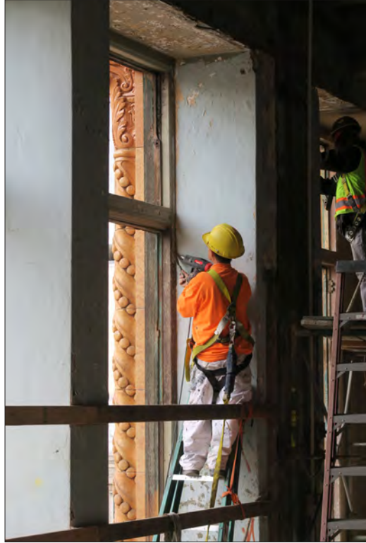
Image 108: Subject property, floor 5, construction work at windows (Chattel, 2019)
