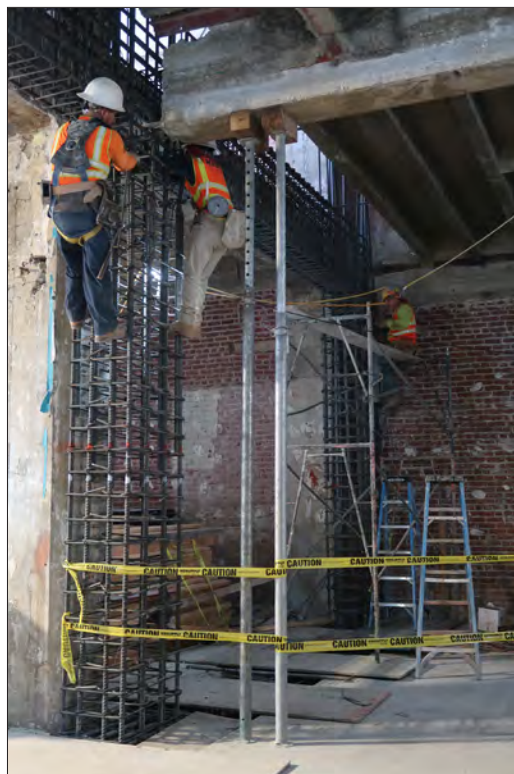
Image 19: Subject property, floor 1, work on moment frame (Chattel, 2019)
