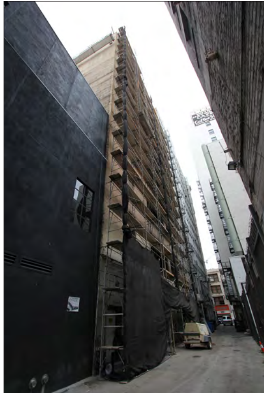
Image 8: Subject property, east elevation, view north (Chattel, 2019)
