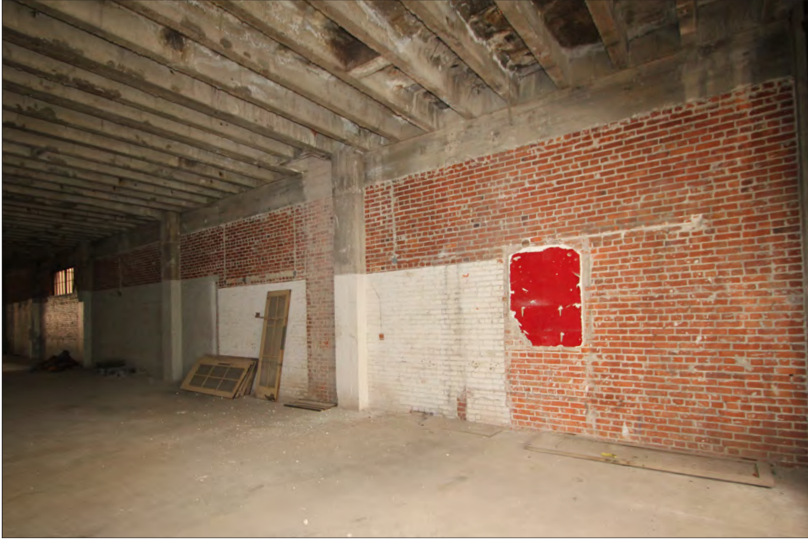
Image 94: Subject property, floor 5, view north (Chattel, 2019)
