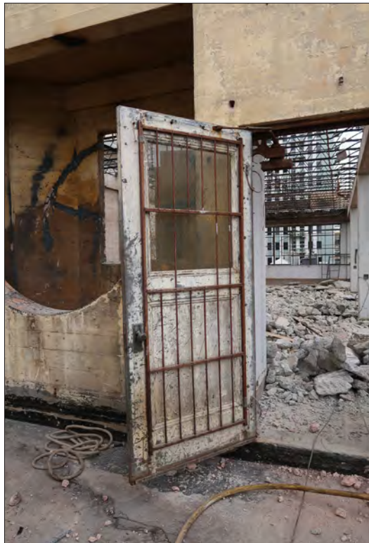
Image 139: Subject property, roof, view east (Chattel, 2019)
