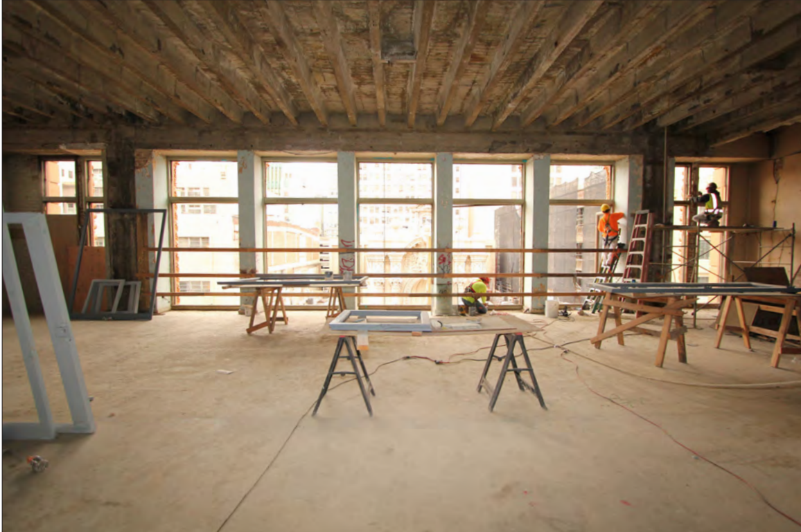
Image 104: Subject property, floor 5, windows at west elevation, view northwest (Chattel, 2019)
