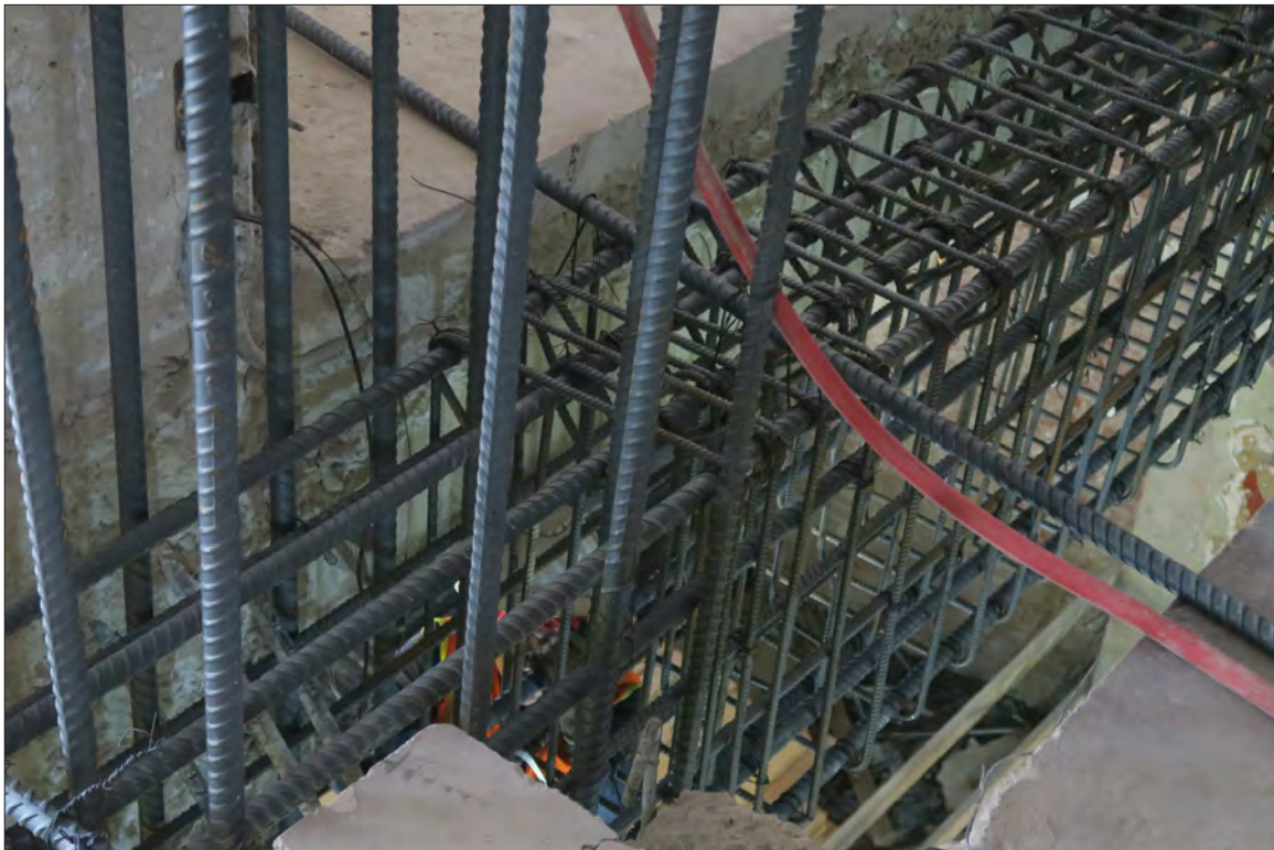
Image 53: Subject property, floor 2, work on moment frame (Chattel, 2019)
