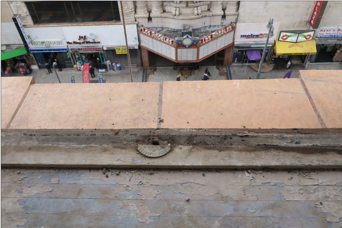
Image 127: Subject property, floor 6 exterior , detail of pivot window hardware at west elevation, view northwest (Chattel, 2019)
