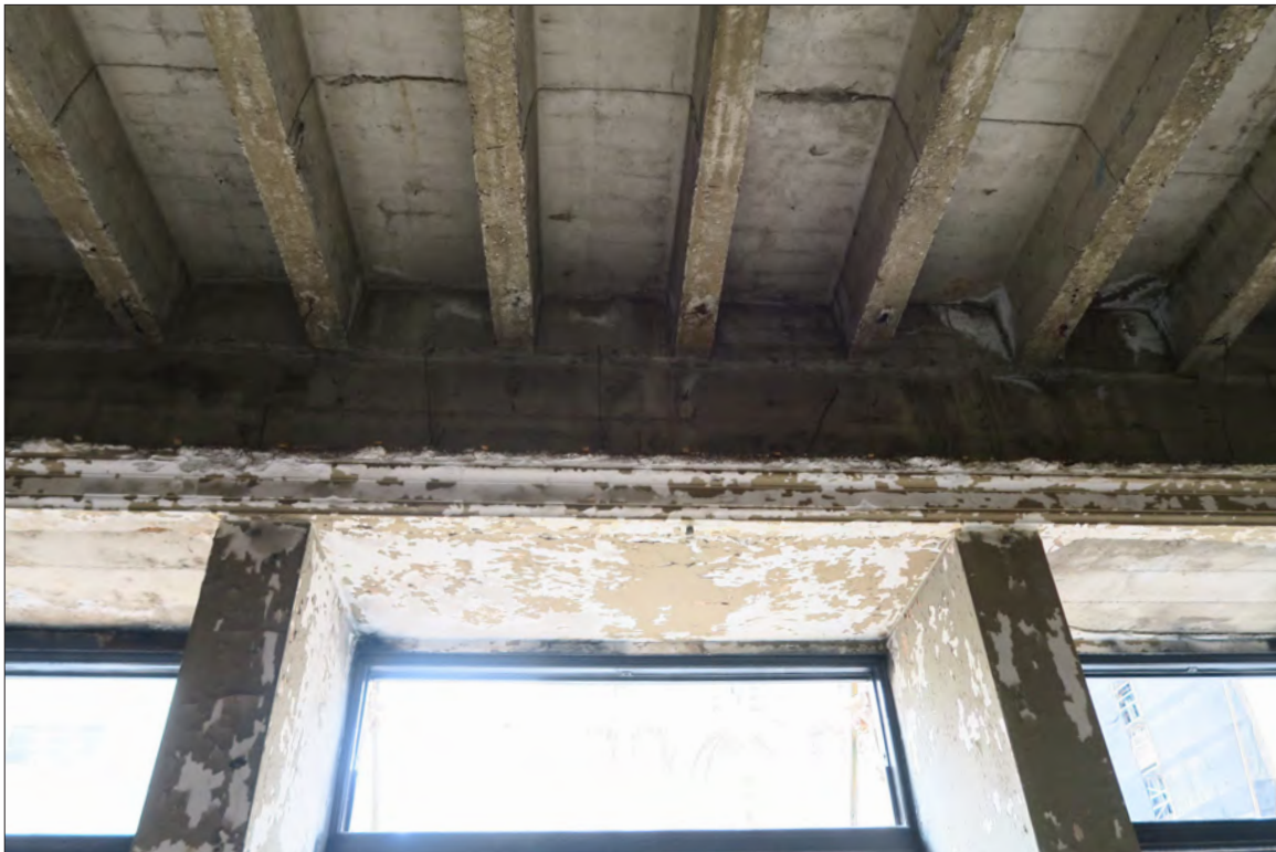
Image 61: Subject property, floor 2, detail of window and ceiling, view northwest (Chattel, 2019)
