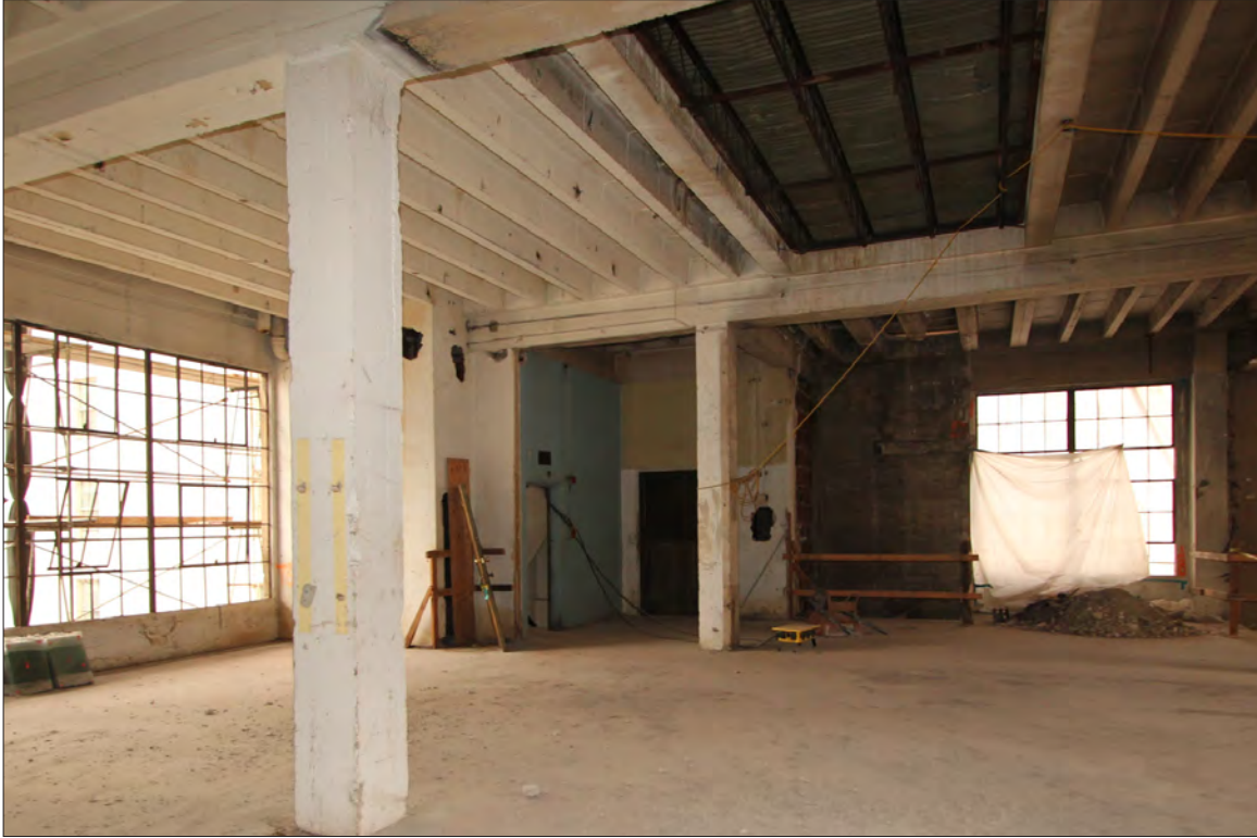
Image 111: Subject property, floor 6, rear staircase and elevator, view south (Chattel, 2019)
