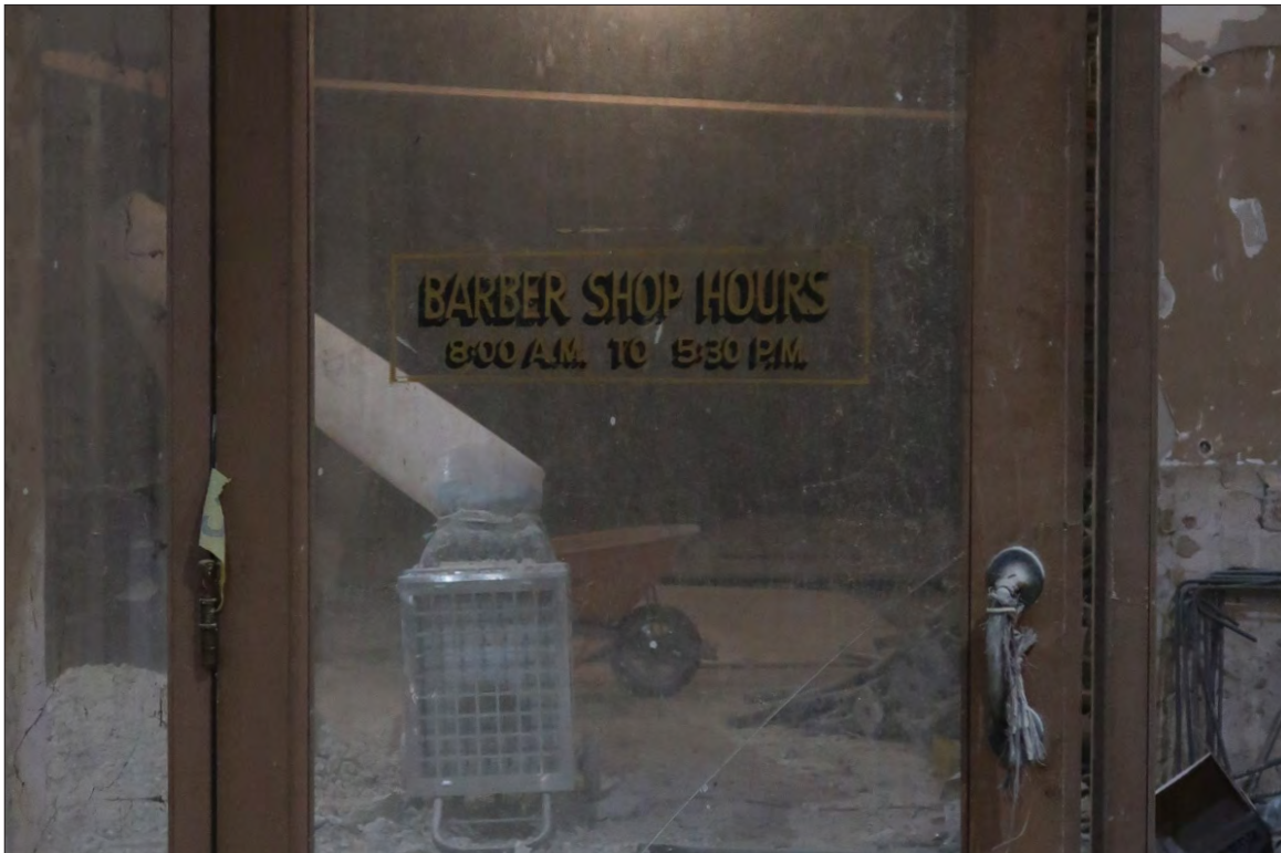
Image 33: Subject property, basement, detail of original barber shop door with posted hours (Chattel, 2019)
