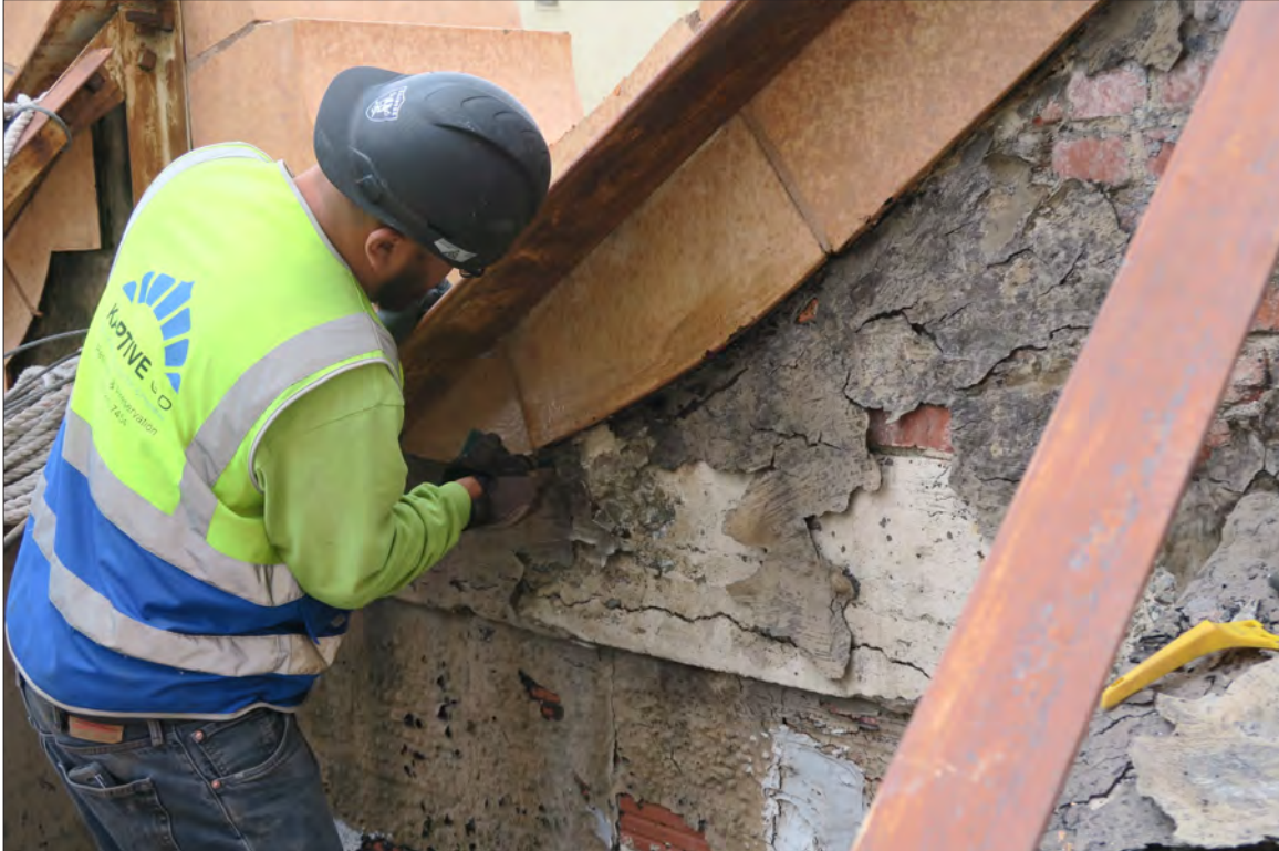
Image 150: Subject property, roof, work at parapet on facade, view west (Chattel, 2019)
