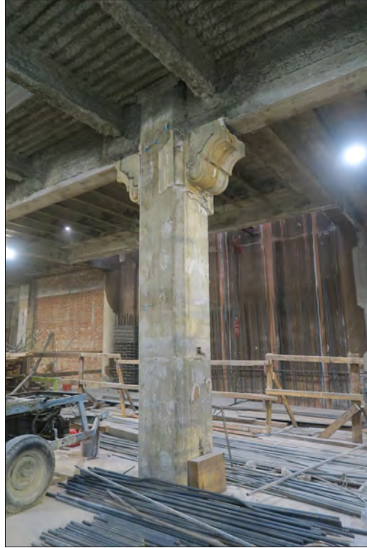
Image 14: Subject property, floor 1, column (Chattel, 2019)
