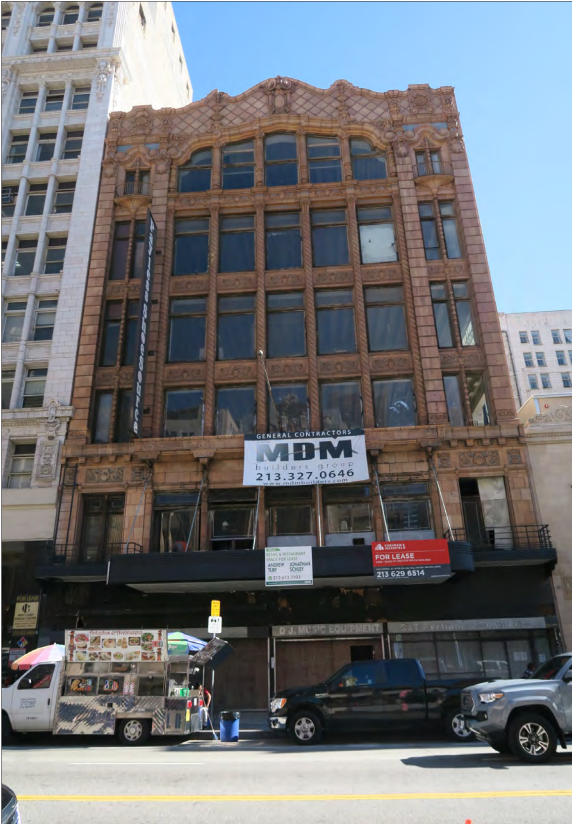
Image 1: Subject property, west elevation, view southeast (Chattel, 2019)
