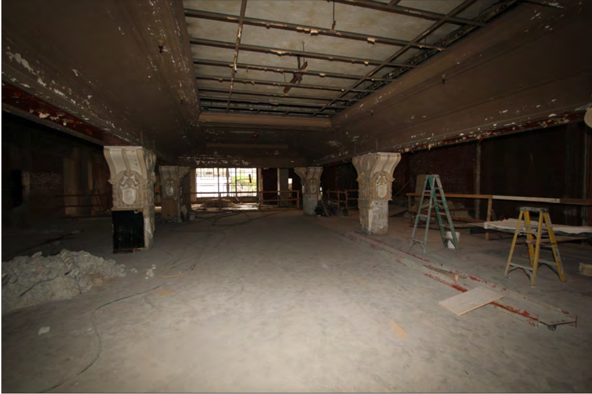
Image 48: Subject property, floor 2, view northwest (Chattel, 2019)
