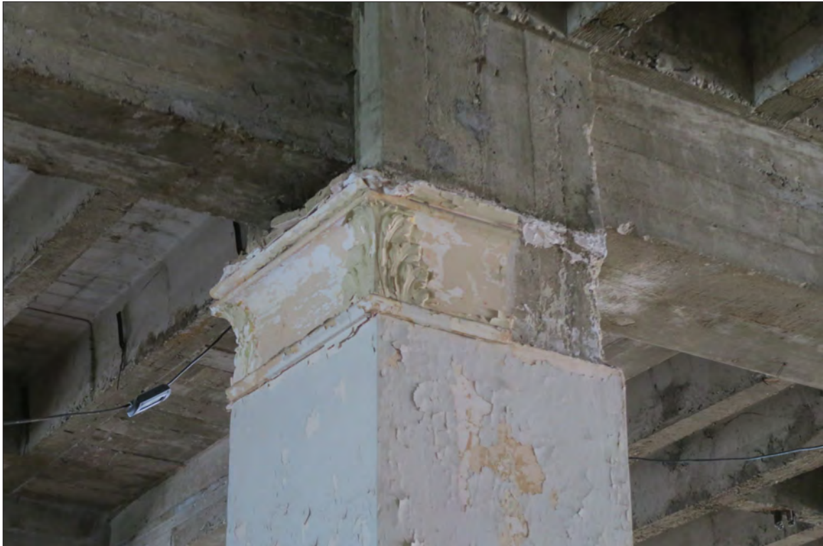
Image 71: Subject property, floor 3, detail of column (Chattel, 2019)
