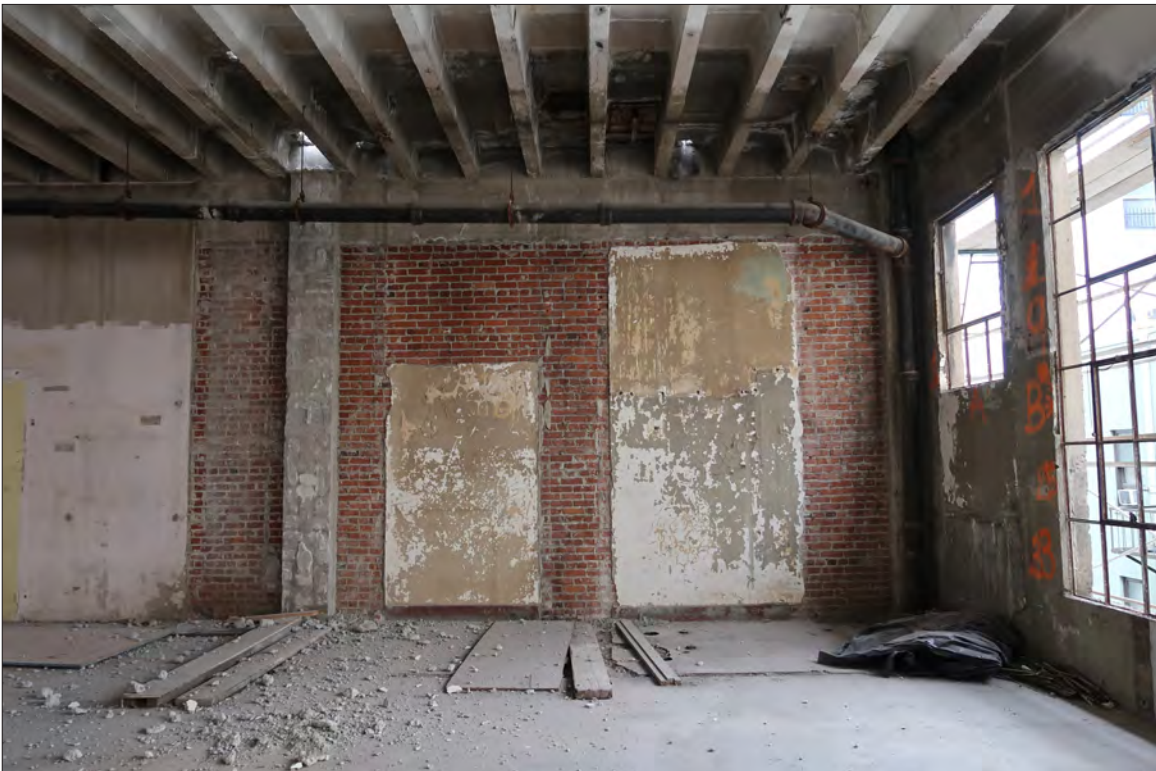
Image 114: Subject property, floor 6, view northeast (Chattel, 2019)
