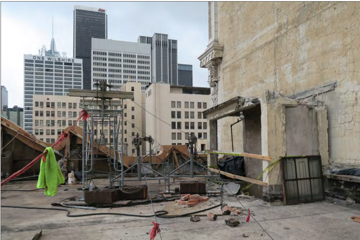
Image 143: Subject property, roof, view northwest (Chattel, 2019)
