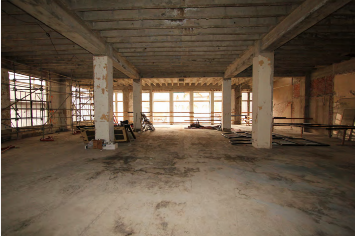
Image 86: Subject property, floor 4, view northwest (Chattel, 2019)
