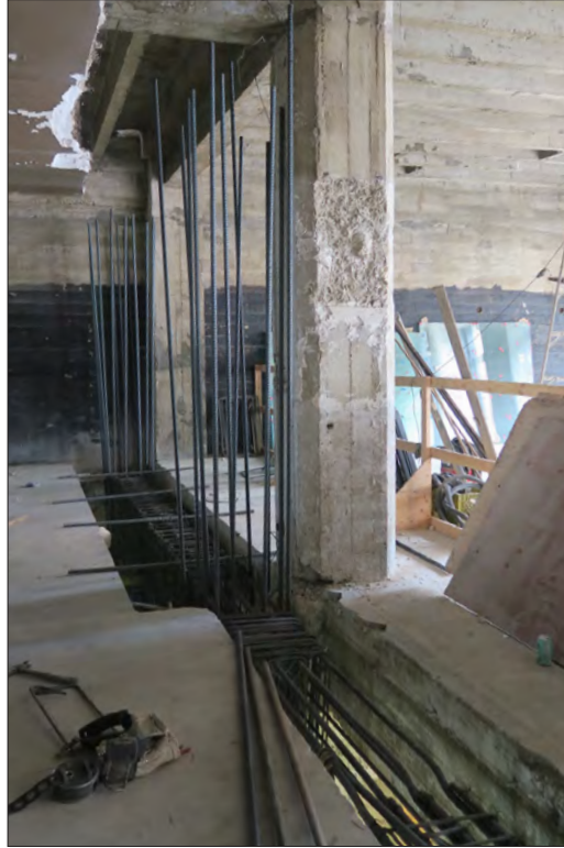
Image 52: Subject property, floor 2, work on moment frame (Chattel, 2019)
