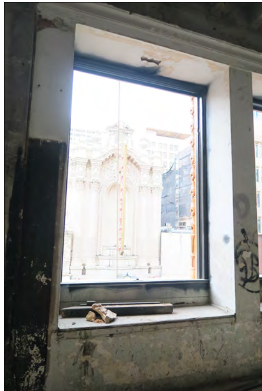
Image 75: Subject property, floor 3, window at west elevation, view north (Chattel, 2019)
