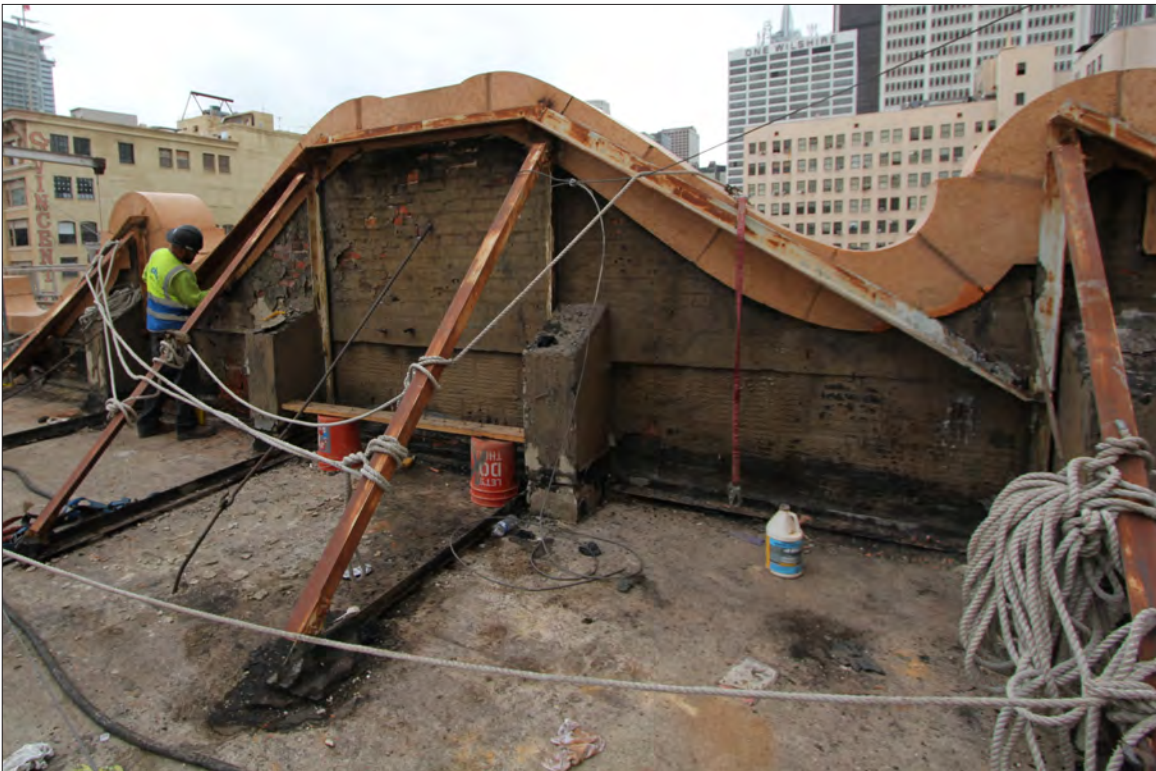
Image 149: Subject property, roof, work at parapet on facade, view west (Chattel, 2019)
