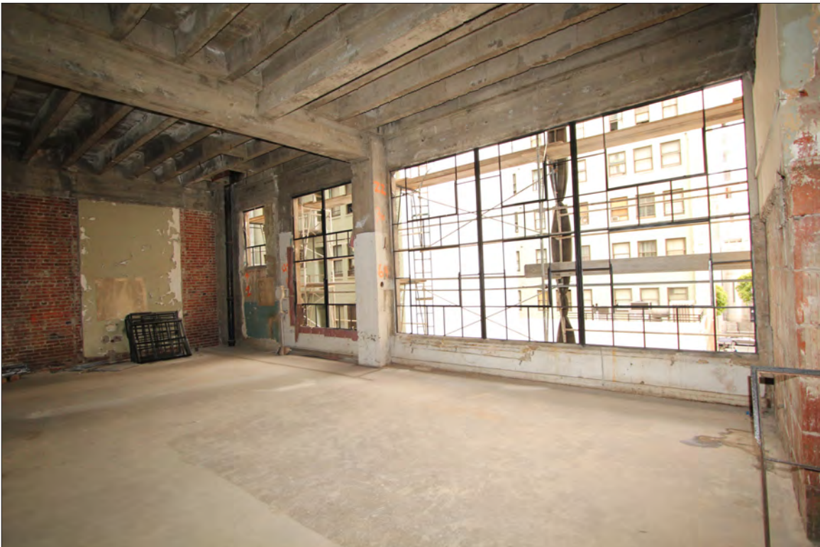
Image 65: Subject property, floor 3, windows at east elevation, view east (Chattel, 2019)
