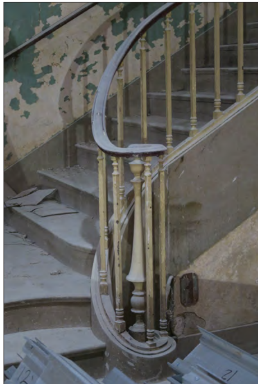
Image 31: Subject property, basement, detail of original stair balustrade, view north (Chattel, 2019)
