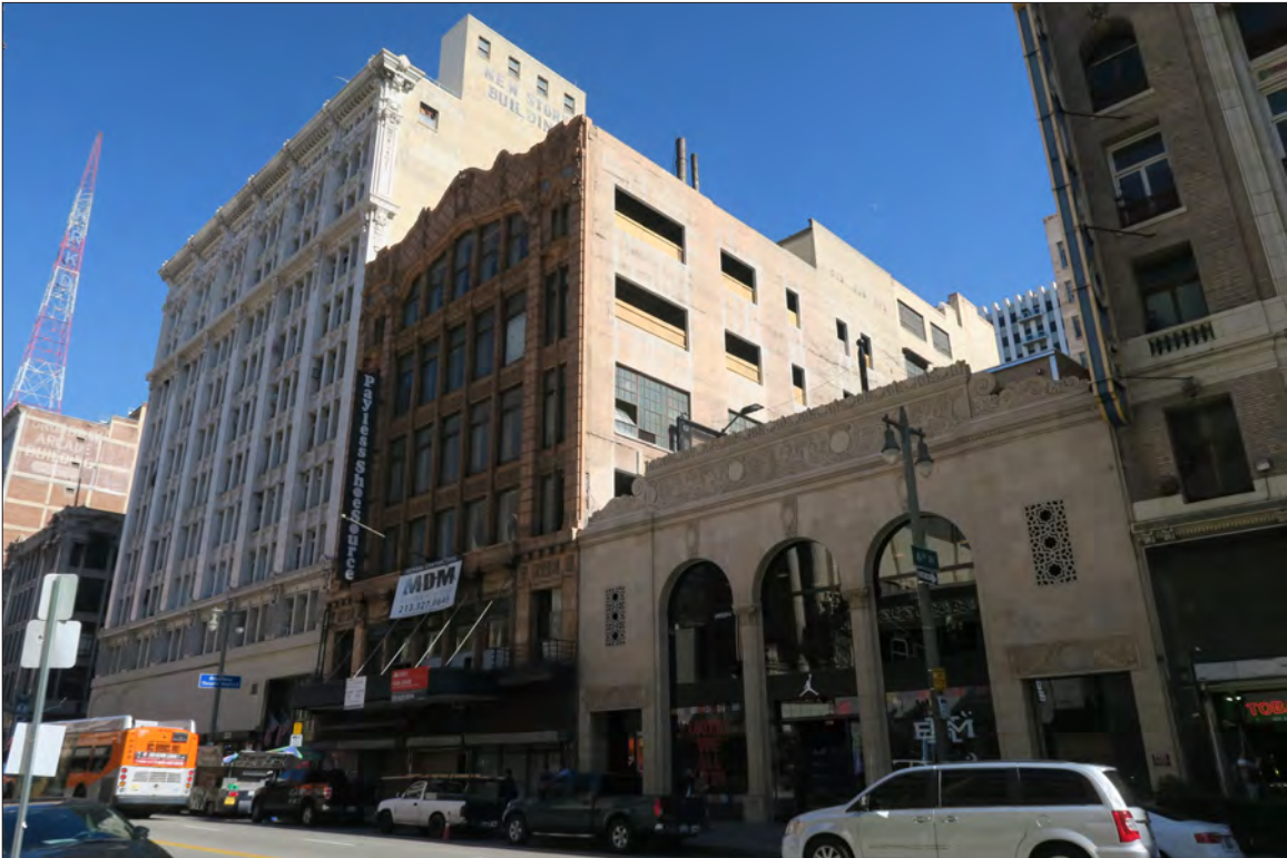
Image 3: Subject property, west elevation, view east (Chattel, 2019)
