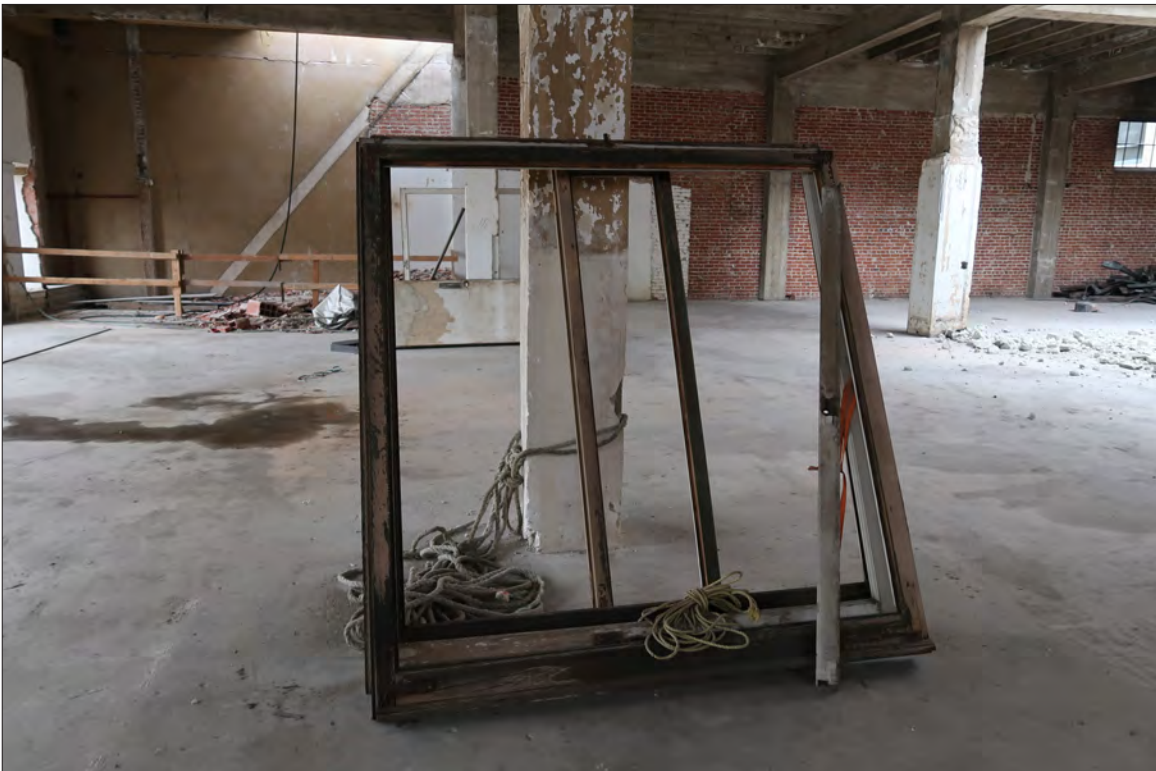
Image 120: Subject property, floor 6, detail of removed historic window (Chattel, 2019)
