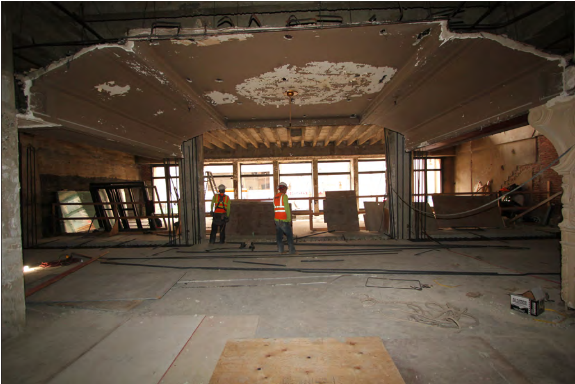
Image 50: Subject property, floor 2, view northwest (Chattel, 2019)
