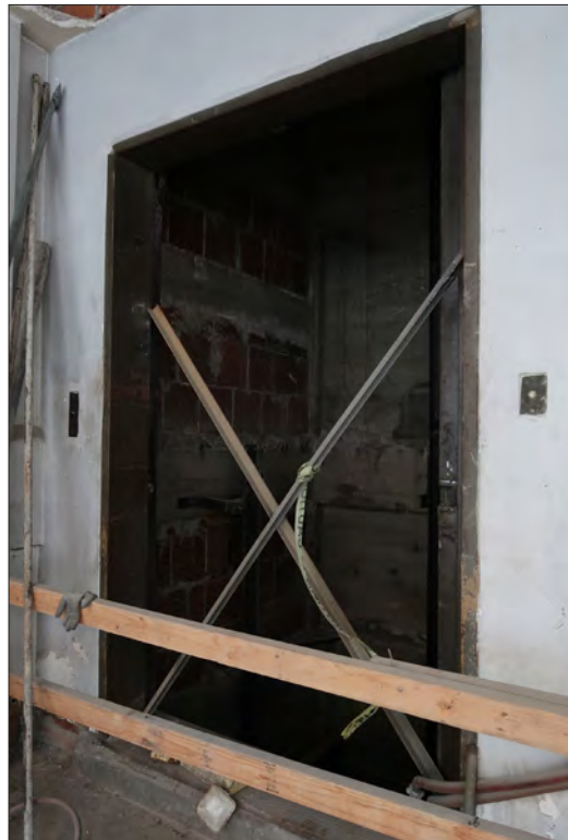
Image 133: Subject property, roof, elevator, view southeast (Chattel, 2019)
