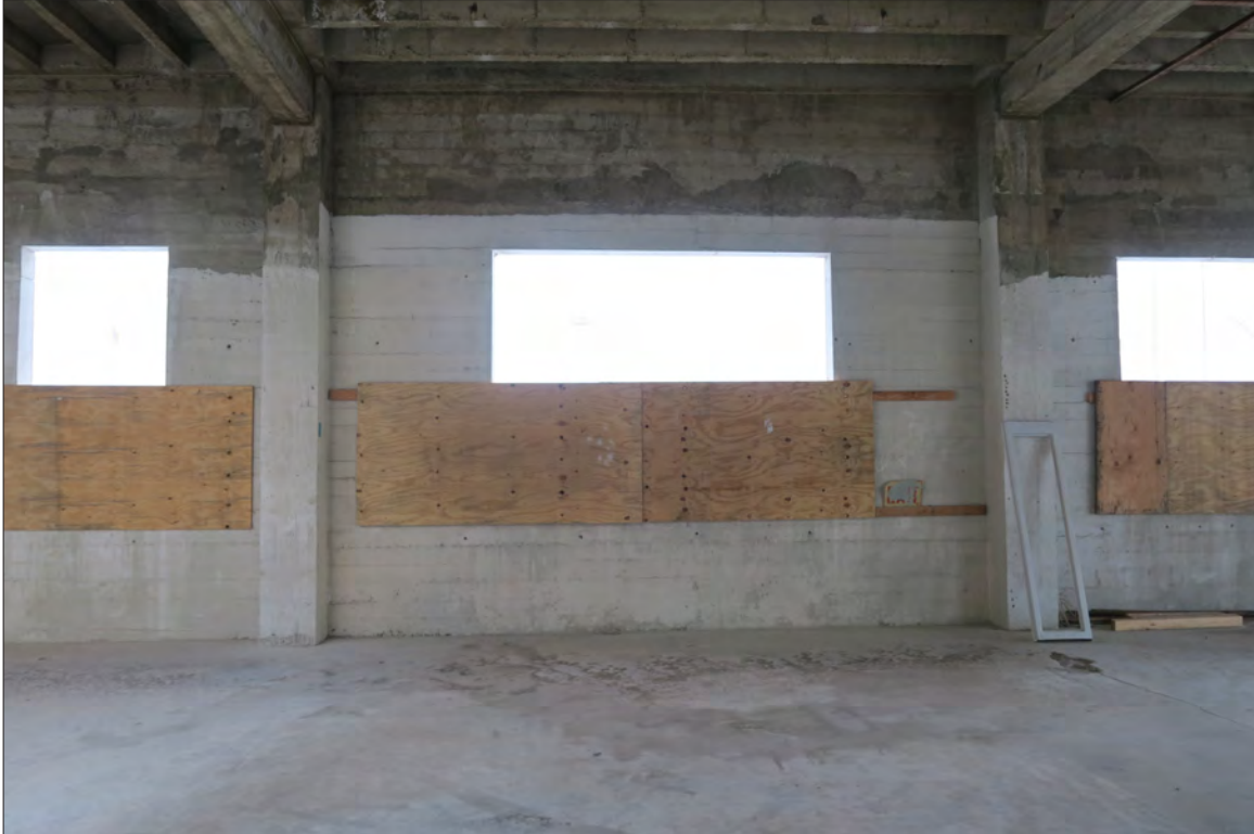
Image 119: Subject property, floor 6, view southwest (Chattel, 2019)
