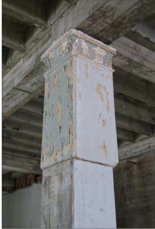
Image 102: Subject property, floor 5, detail of column (Chattel, 2019)
