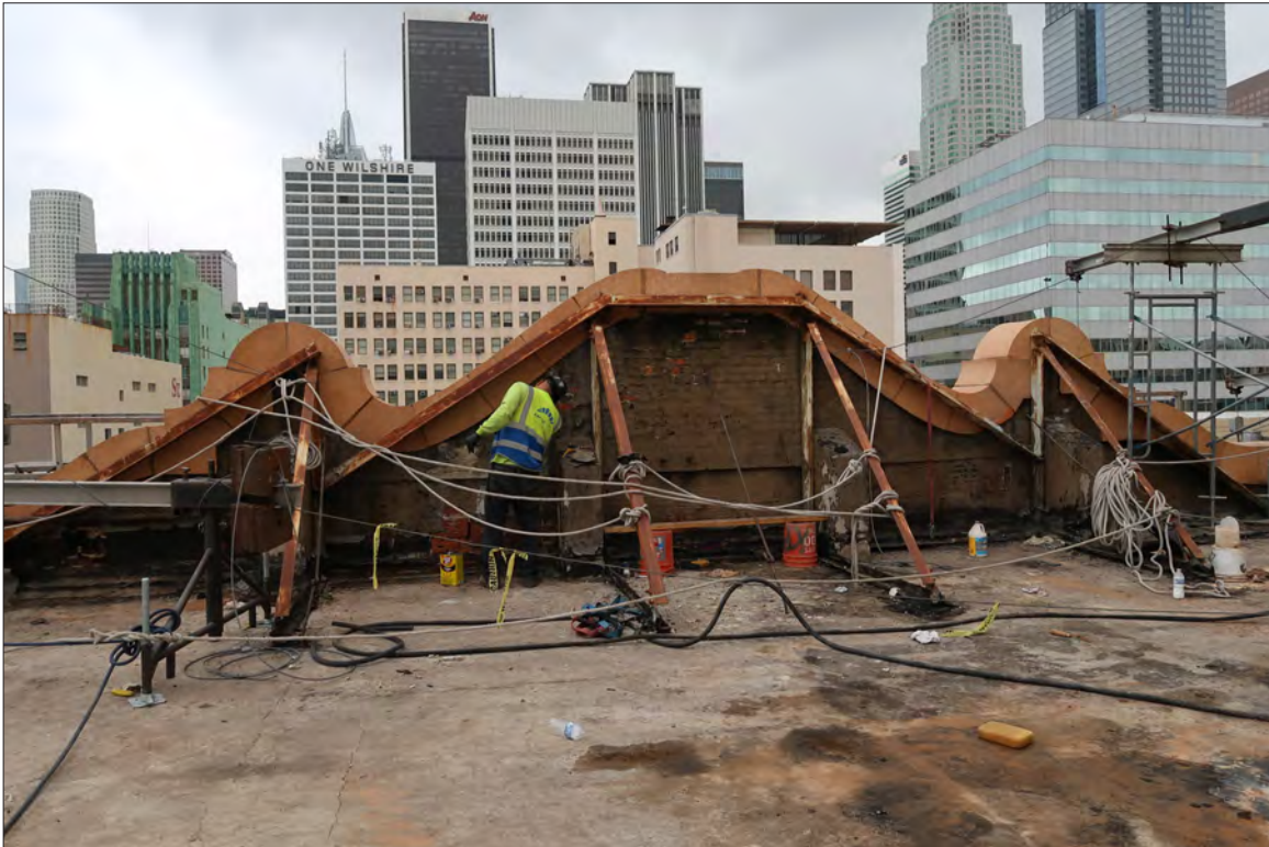
Image 148: Subject property, roof, work at parapet on facade, view northwest (Chattel, 2019)
