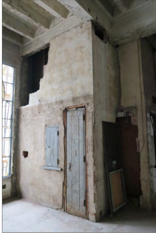
Image 80: Subject property, floor 4, view south (Chattel, 2019)
