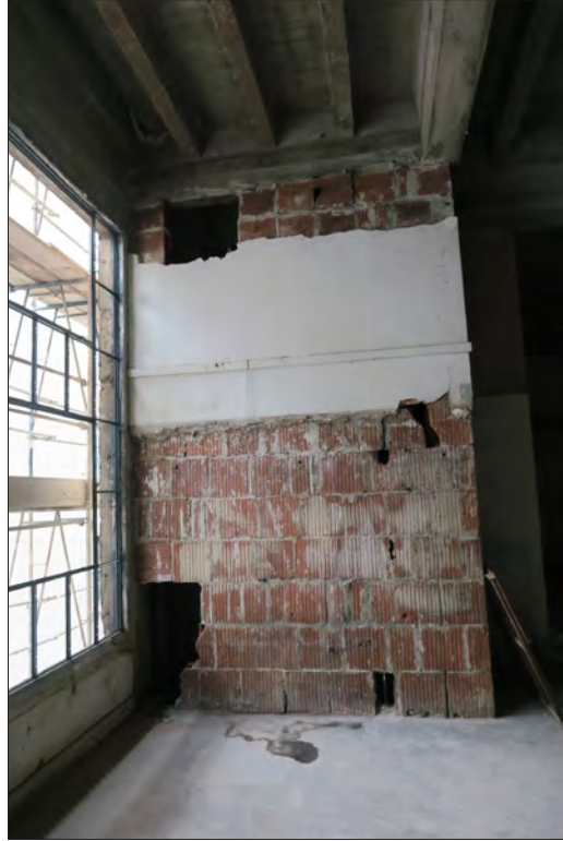
Image 66: Subject property, floor 3, view southwest (Chattel, 2019)
