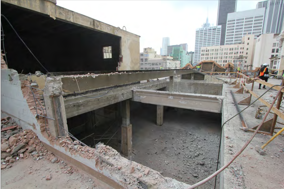
Image 140: Subject property, roof, view west (Chattel, 2019)
