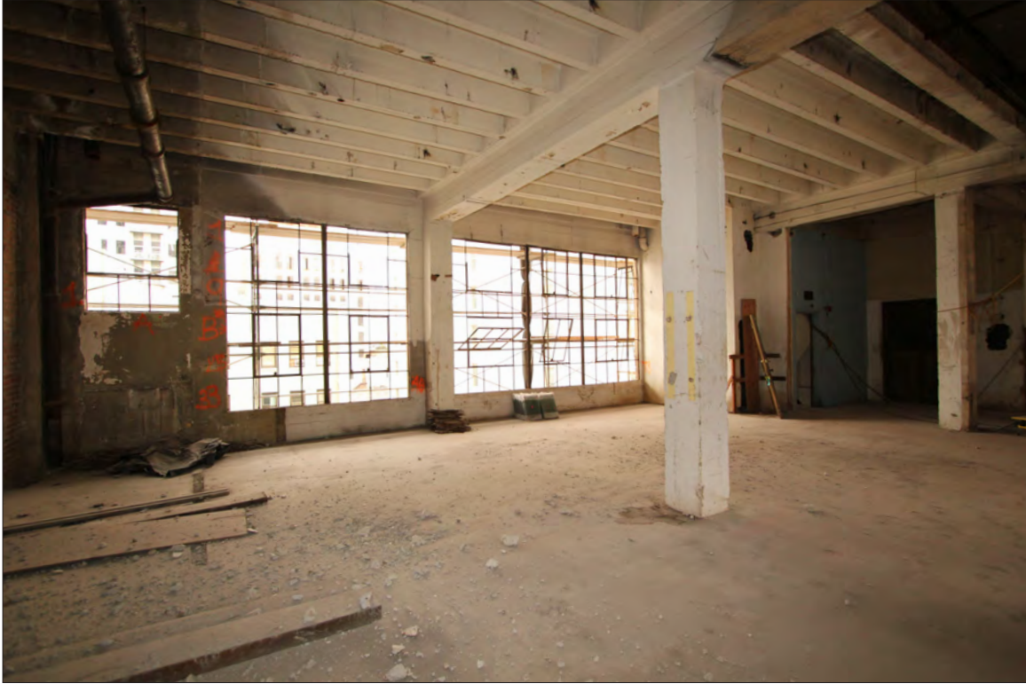
Image 113: Subject property, floor 6, windows at east elevation, view southeast (Chattel, 2019)
