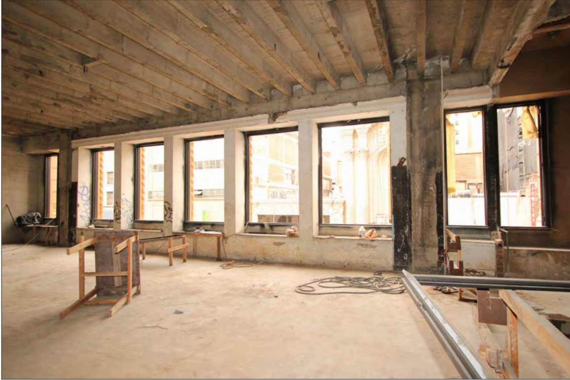
Image 74: Subject property, floor 3, windows at west elevation, view west (Chattel, 2019)
