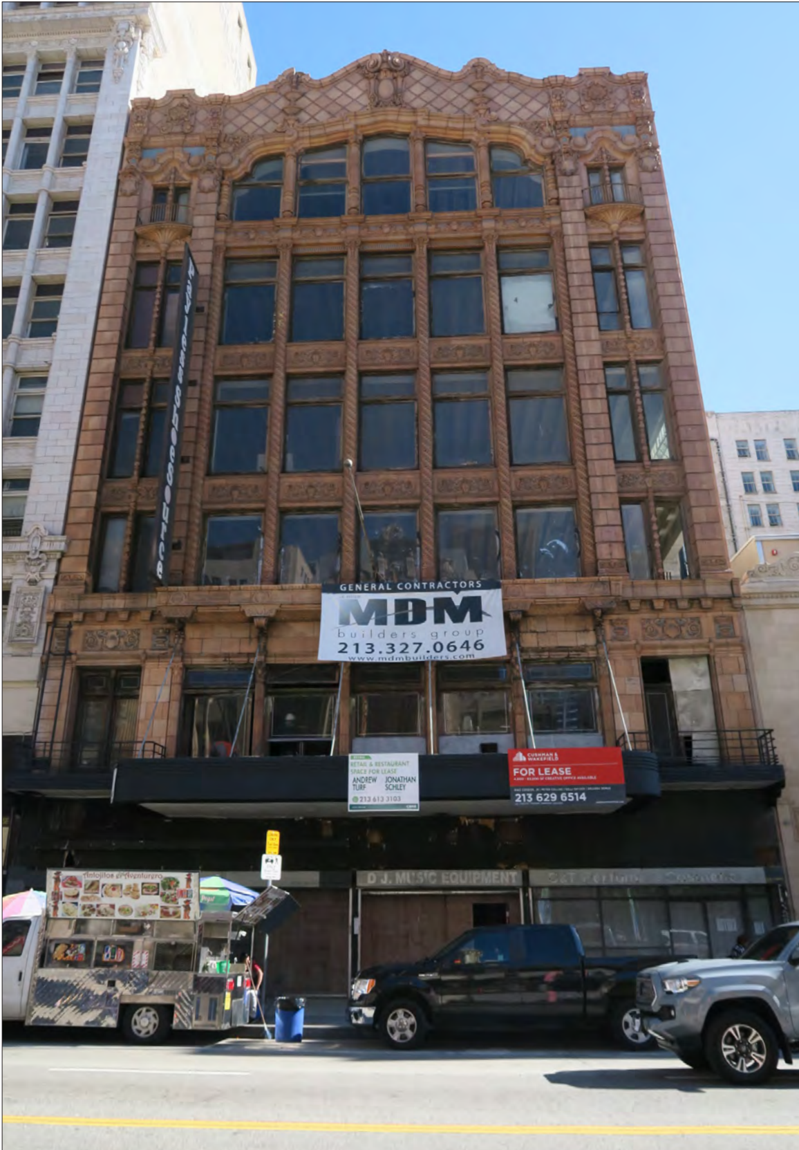
Image 1: Subject property, west elevation, view southeast (Chattel, 2019)
