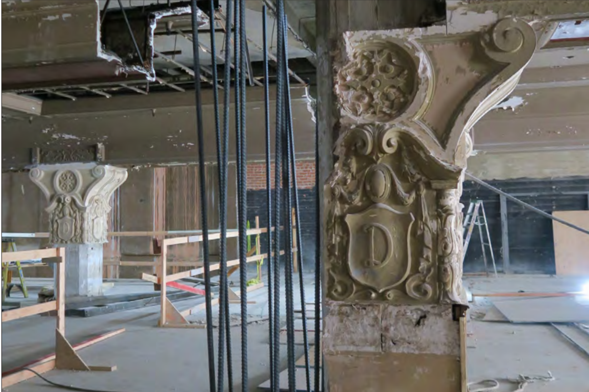
Image 56: Subject property, floor 2, detail of mezzanine column, view southwest (Chattel, 2019)
