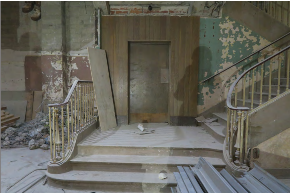
Image 29: Subject property, basement, view north (Chattel, 2019)
