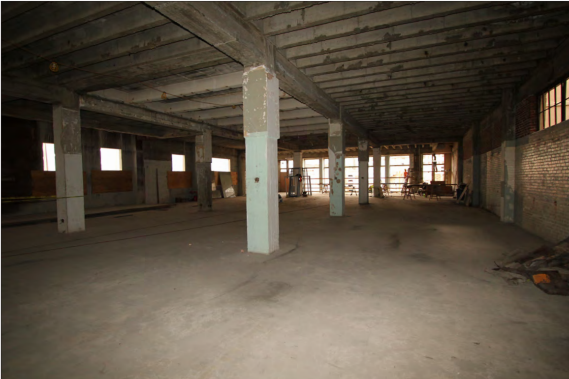
Image 95: Subject property, floor 5, view west (Chattel, 2019)
