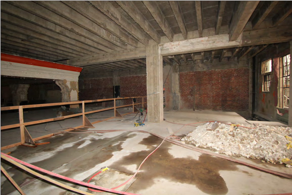
Image 43: Subject property, floor 2, view east (Chattel, 2019)
