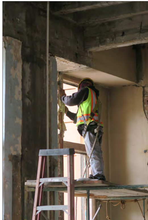
Image 107: Subject property, floor 5, construction work at windows (Chattel, 2019)
