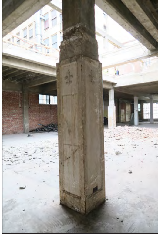
Image 117: Subject property, floor 6, column (Chattel, 2019)
