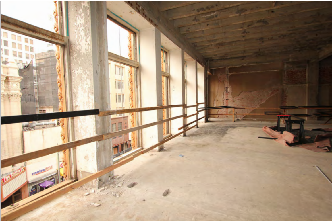
Image 89: Subject property, floor 4, windows at west elevation, view north (Chattel, 2019)
