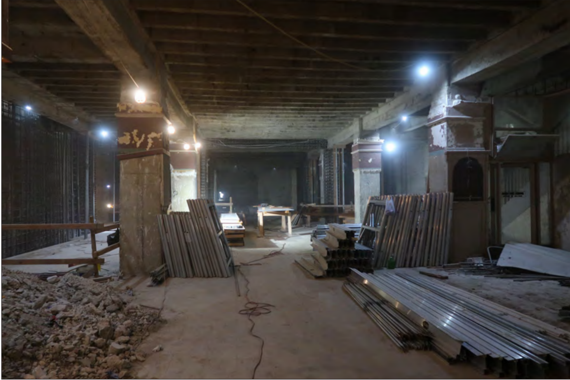
Image 26: Subject property, basement, view northwest (Chattel, 2019)
