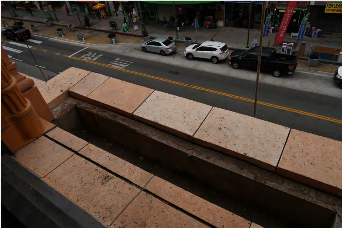
Image 76: Subject property, floor 3 exterior , detail of planters at west elevation, view west (Chattel, 2019)
