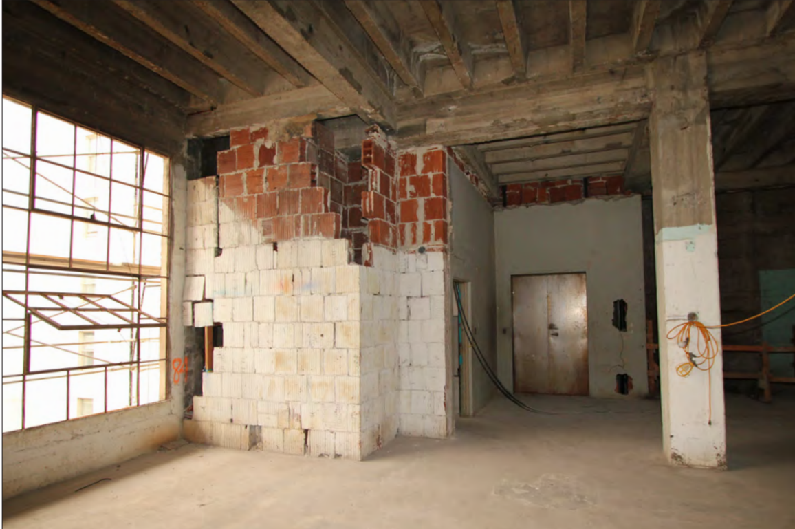
Image 90: Subject property, floor 5, rear staircase and elevator , view south (Chattel, 2019)
