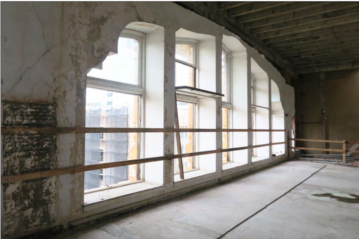
Image 124: Subject property, floor 6, windows at west elevation, view north (Chattel, 2019)
