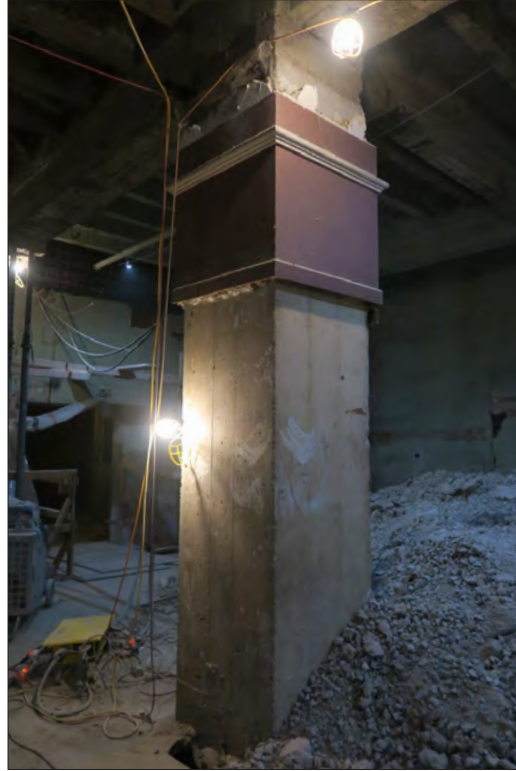
Image 40: Subject property, basement, column details (Chattel, 2019)
