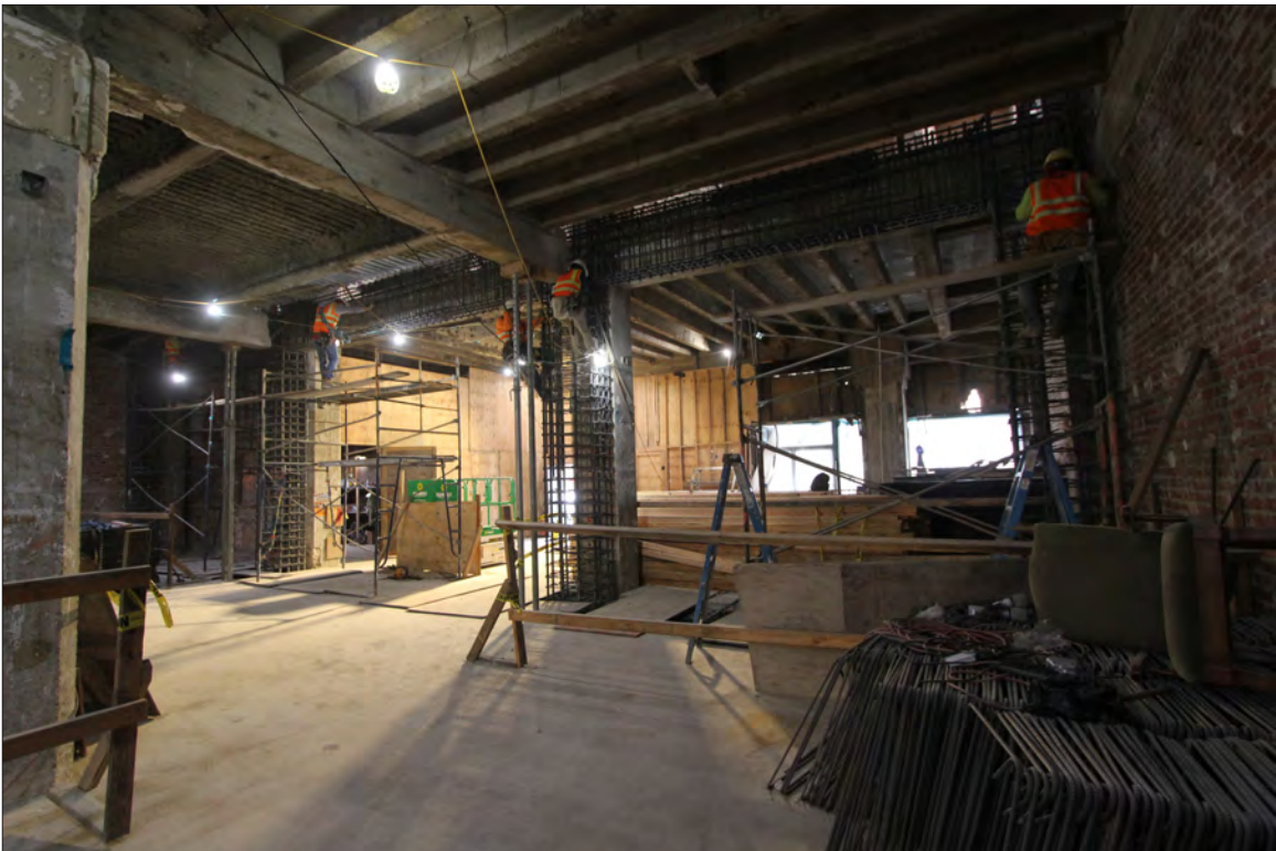
Image 13: Subject property, floor 1, work on moment frame, view west (Chattel, 2019)
