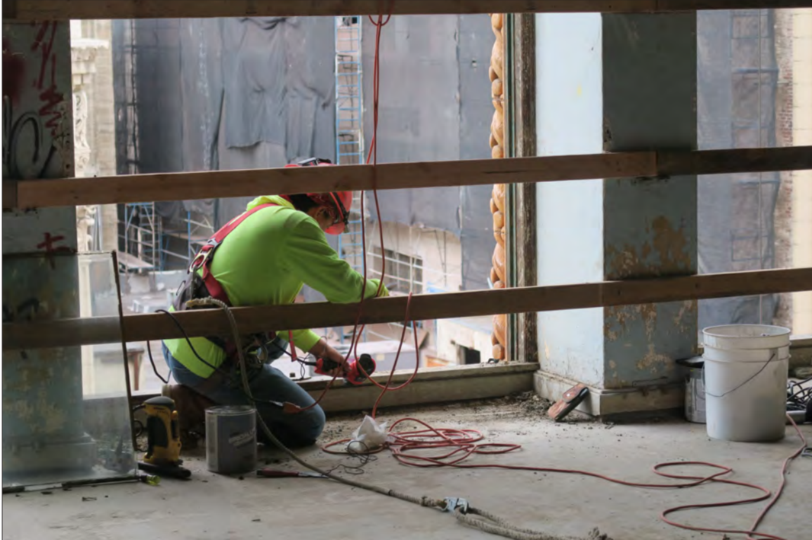
Image 106: Subject property, floor 5, construction work at windows (Chattel, 2019)
