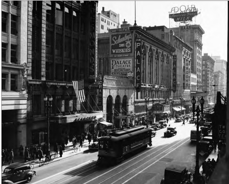
Image 5: Subject property, west elevation, view south (USC Digital Library, 1938)
