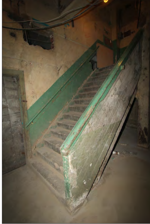
Image 22: Subject property, basement, stairs from floor 1, view south (Chattel, 2019)
