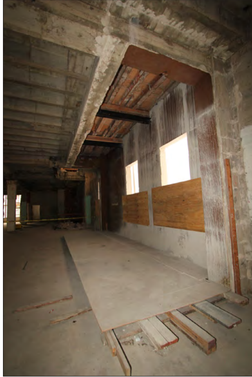
Image 98: Subject property, floor 5, windows at south elevation, view southeast (Chattel, 2019)
