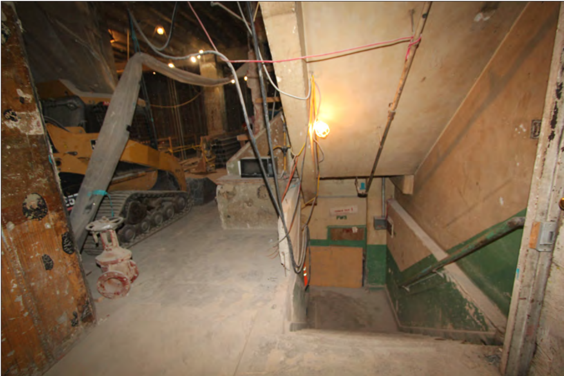
Image 21: Subject property, floor 1, stairs to basement, view north (Chattel, 2019)
