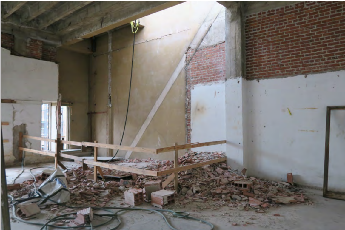
Image 122: Subject property, floor 6, removed stairs at northwest corner, typical view north (Chattel, 2019)
