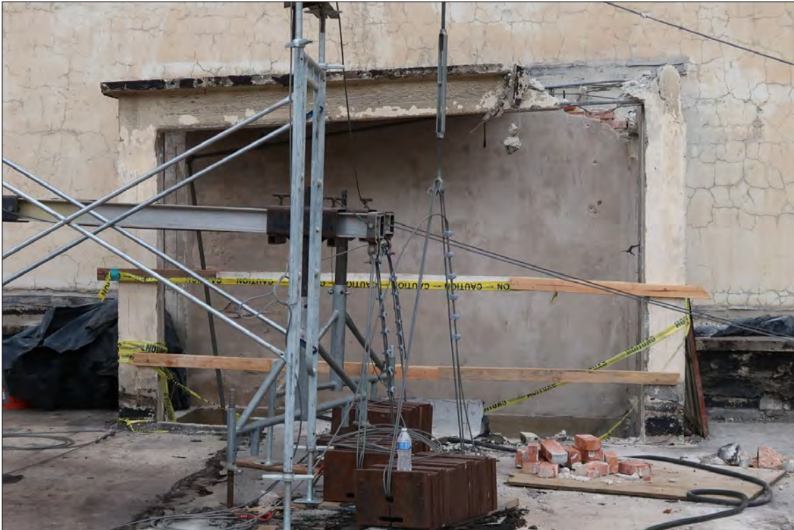
Image 144: Subject property, roof, removed staircase, view northeast (Chattel, 2019)
