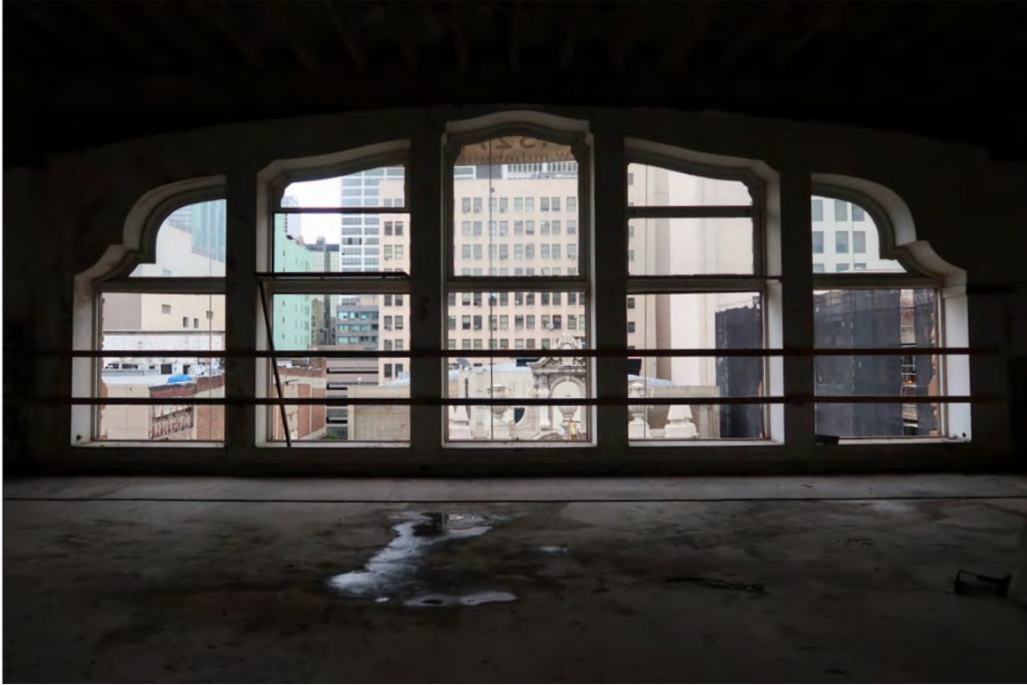
Image 125: Subject property, floor 6, windows at west elevation, view northwest (Chattel, 2019)
