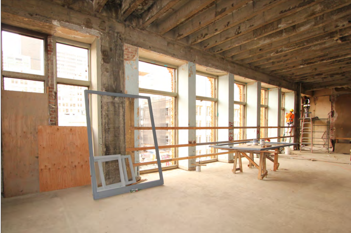
Image 109: Subject property, floor 5, windows at west elevation, view north (Chattel, 2019)
