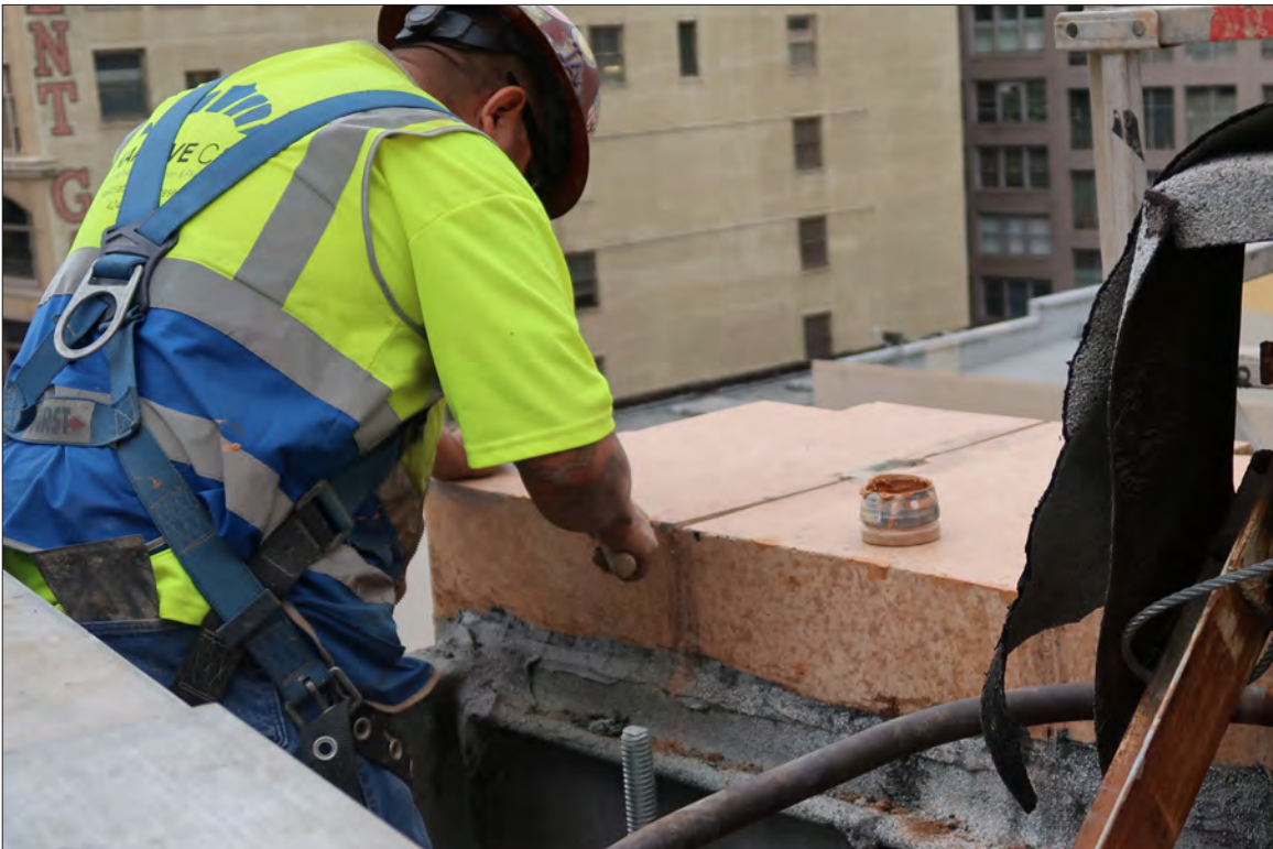
Image 151: Subject property, roof, work at parapet on facade, view west (Chattel, 2019)
