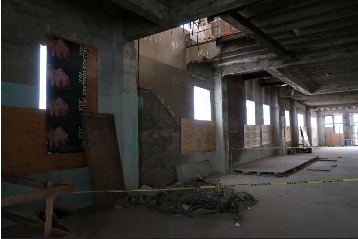
Image 96: Subject property, floor 5, view west (Chattel, 2019)
