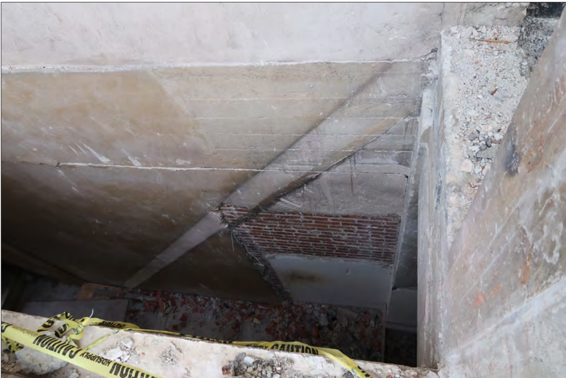
Image 145: Subject property, roof, detail of removed staircase (Chattel, 2019)
