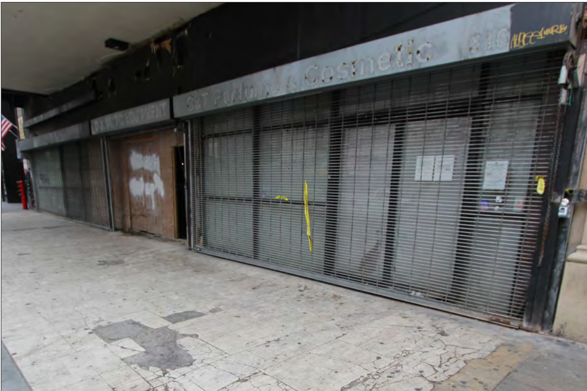
Image 5: Subject property, west elevation, storefront, view east (Chattel, 2019)
