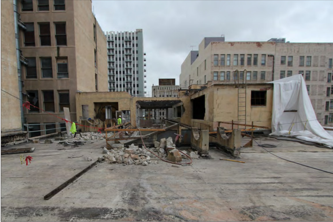
Image 142: Subject property, roof, view southeast (Chattel, 2019)
