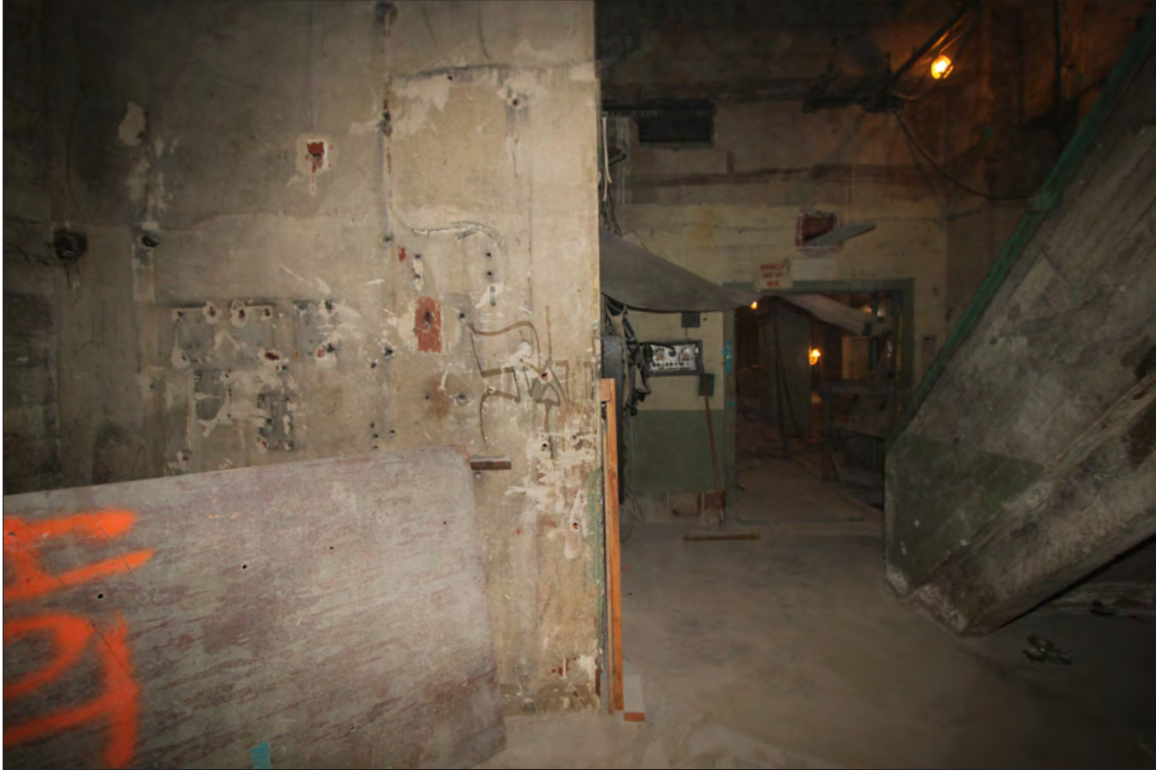
Image 24: Subject property, basement, view north (Chattel, 2019)
