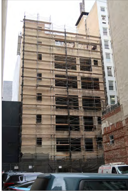
Image 7: Subject property, east elevation, view northwest (Chattel, 2019)
