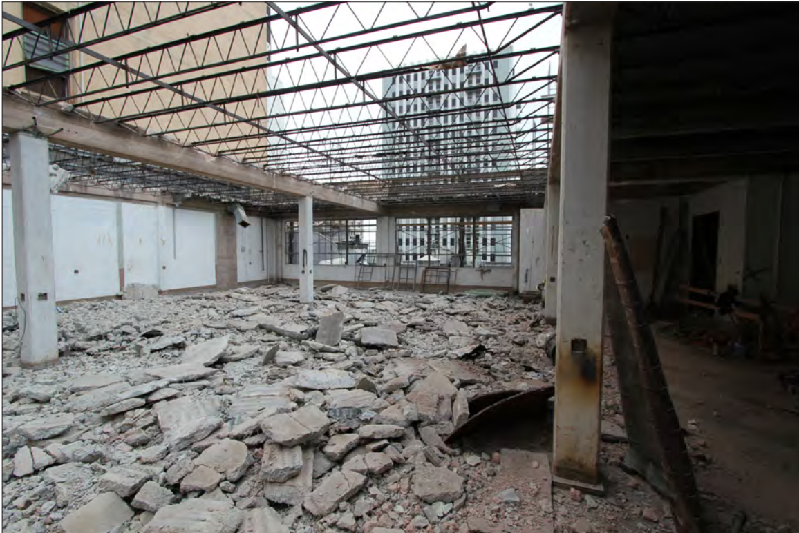
Image 134: Subject property, roof, view east (Chattel, 2019)
