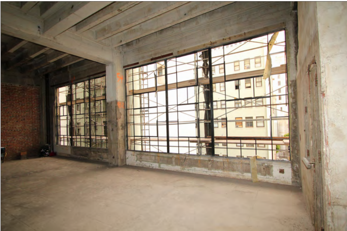
Image 79: Subject property, floor 4, windows at east elevation, view east (Chattel, 2019)
