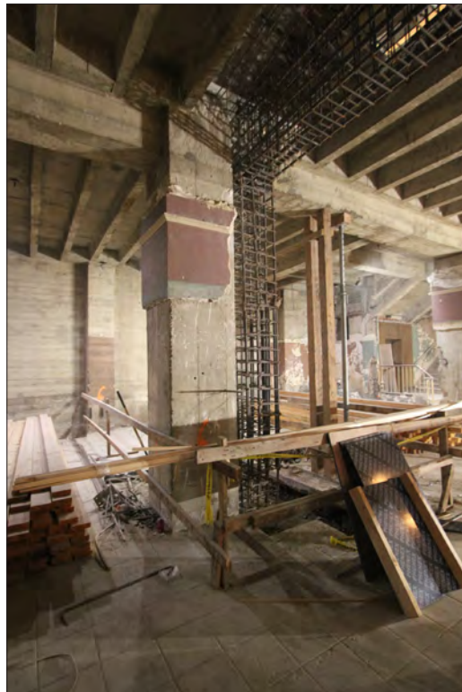
Image 39: Subject property, basement, view northwest (Chattel, 2019)
