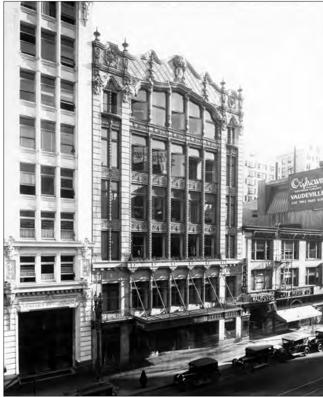
Image 1: Subject property, west elevation, view south (Water and Power Associates, c.1925)
