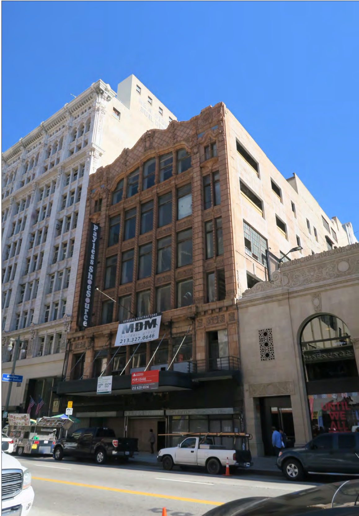
Image 2: Subject property, west elevation, view east (Chattel, 2019)
