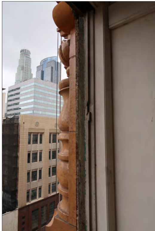
Image 128: Subject property, floor 6 exterior , detail of window frame at west elevation, view northwest (Chattel, 2019)
