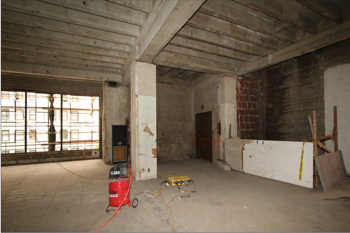
Image 78: Subject property, floor 4, view southeast (Chattel, 2019)
