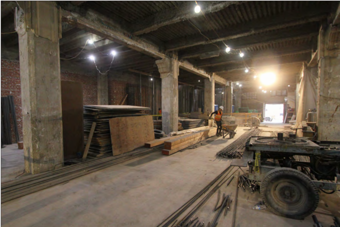
Image 12: Subject property, floor 1, view east (Chattel, 2019)
