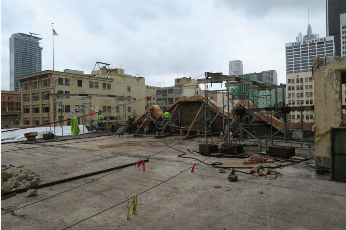
Image 146: Subject property, roof, view west (Chattel, 2019)
