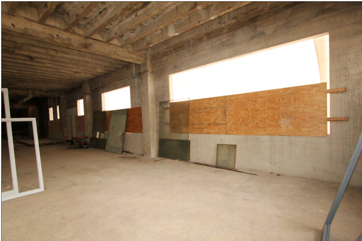
Image 99: Subject property, floor 5, windows at south elevation, view south (Chattel, 2019)
