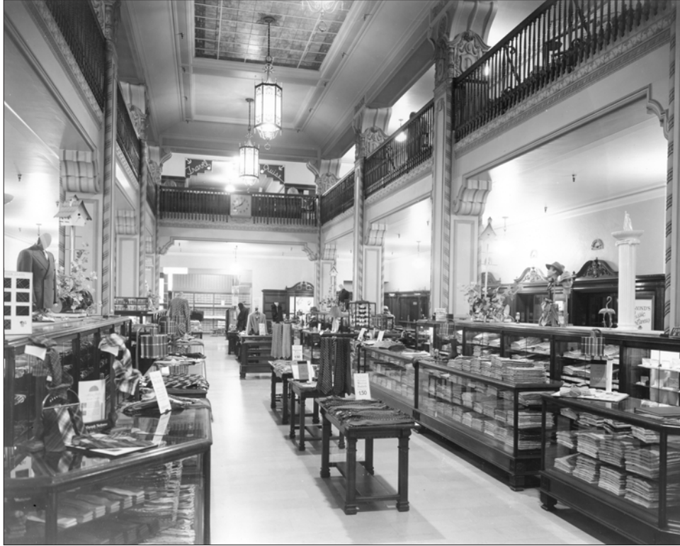
Image 9: Subject property, interior at mezzanine (date unknown)
