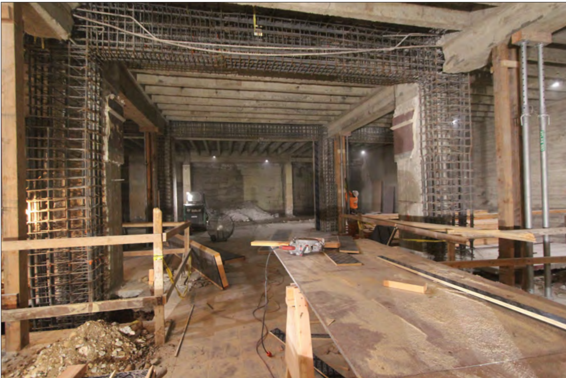
Image 35: Subject property, basement, work on moment frame, view northwest (Chattel, 2019)
