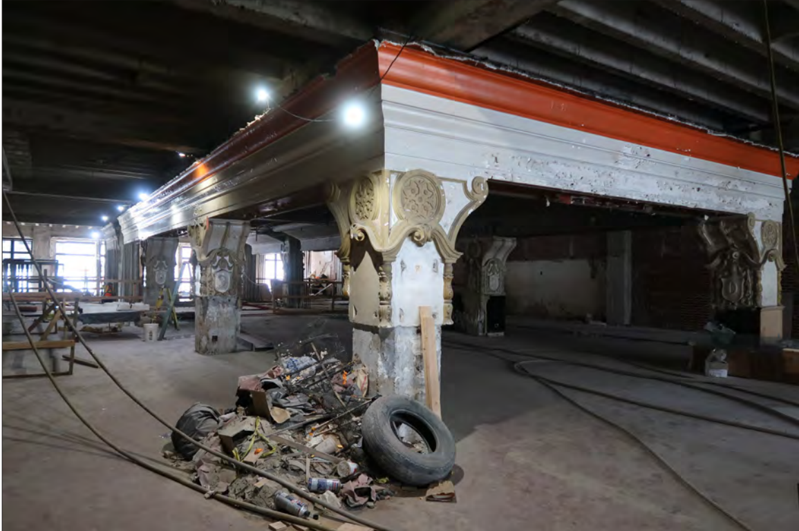
Image 44: Subject property, floor 2, mezzanine, view north (Chattel, 2019)
