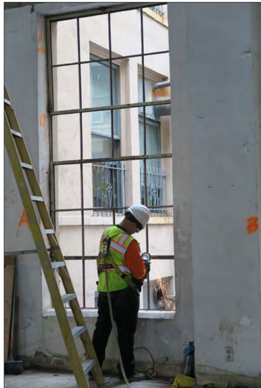
Image 85: Subject property, floor 4, construction work at steel windows (Chattel, 2019)
