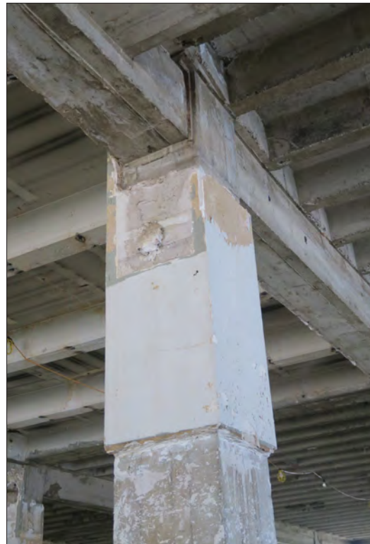
Image 103: Subject property, floor 5, detail of column (Chattel, 2019)
