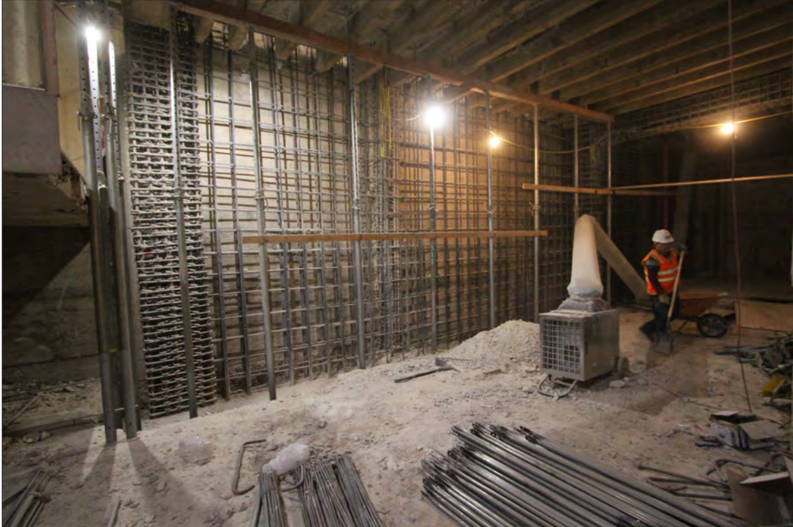
Image 34: Subject property, basement, work on shear wall, view northeast (Chattel, 2019)
