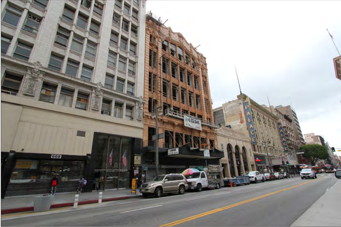
Image 2: Subject property, west elevation, view south (Chattel, 2019)
