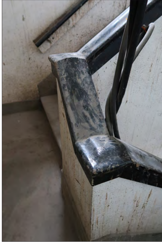
Image 131: Subject property, stairwell, detail of balustrade (Chattel, 2019)
