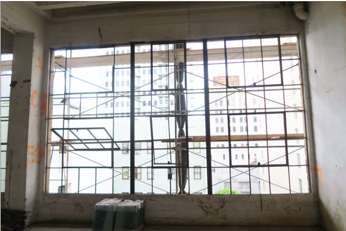
Image 112: Subject property, floor 6, windows at east elevation, view southeast (Chattel, 2019)
