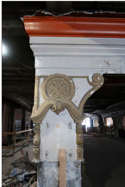
Image 45: Subject property, floor 2, detail of mezzanine corne , view northwest (Chattel, 2019)
