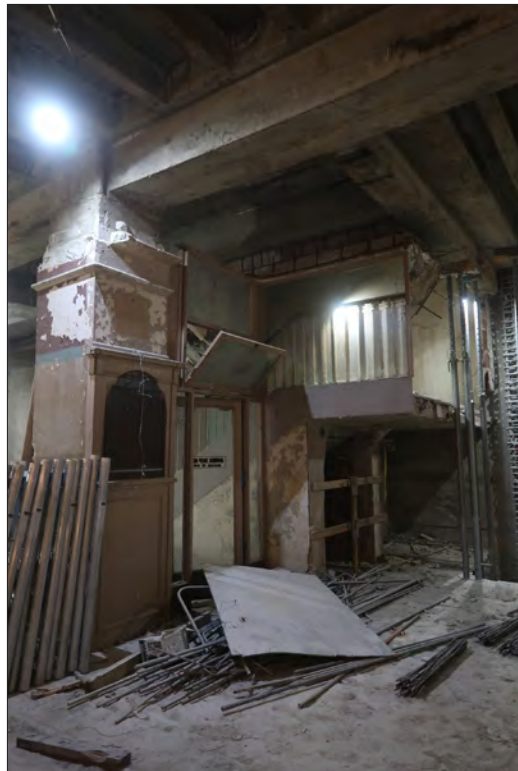
Image 27: Subject property, basement, view north (Chattel, 2019)
