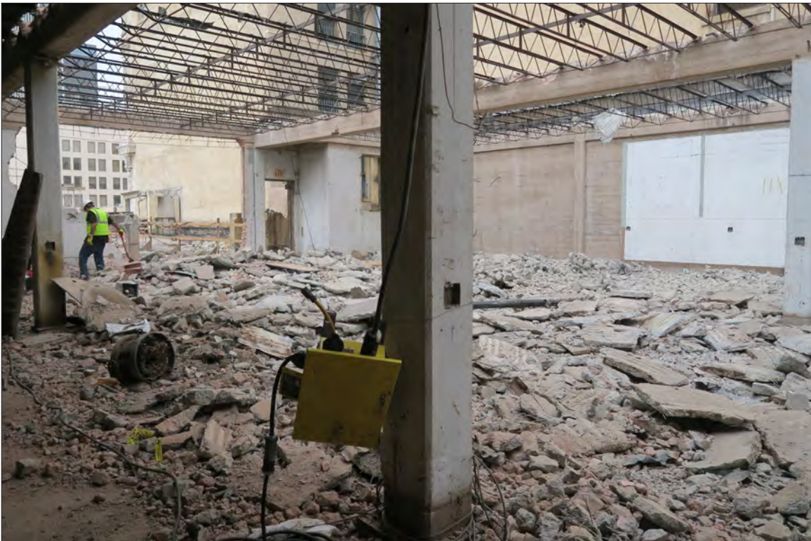
Image 135: Subject property, roof, view north (Chattel, 2019)
