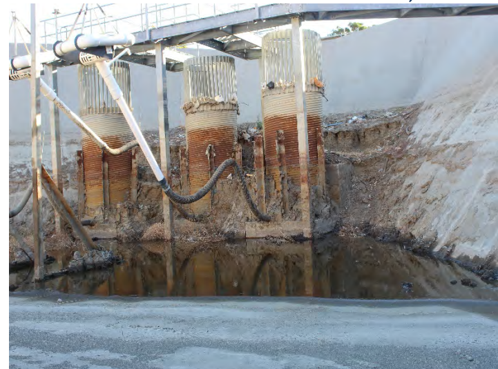
Photo 284: Terminal Basin Outlet Risers: December 16, 2020
