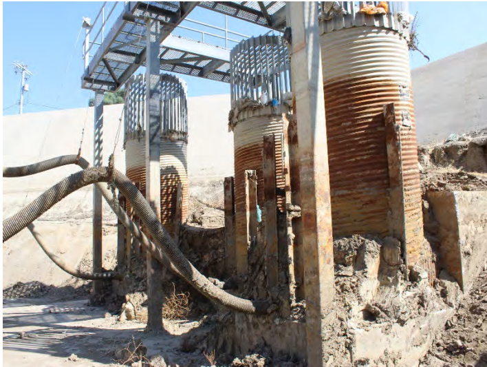
Photo 265: Terminal Basin Outlet Risers: October 20, 2020
