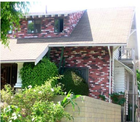
*It is inappropriate to cover wood siding or other details with vinyl, stucco, or other materials. It is inappropriate to repair wood siding by adding new material that does not match the original.*
