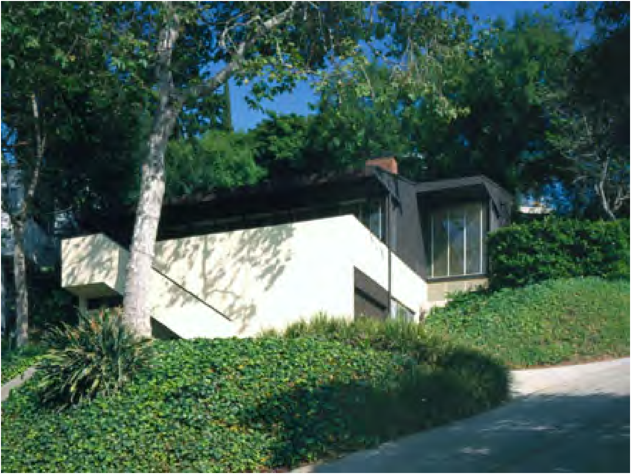
Bonnet House after siding was painted, 2256 El Contento Drive, Undated Photo (Unknown Photographer)
