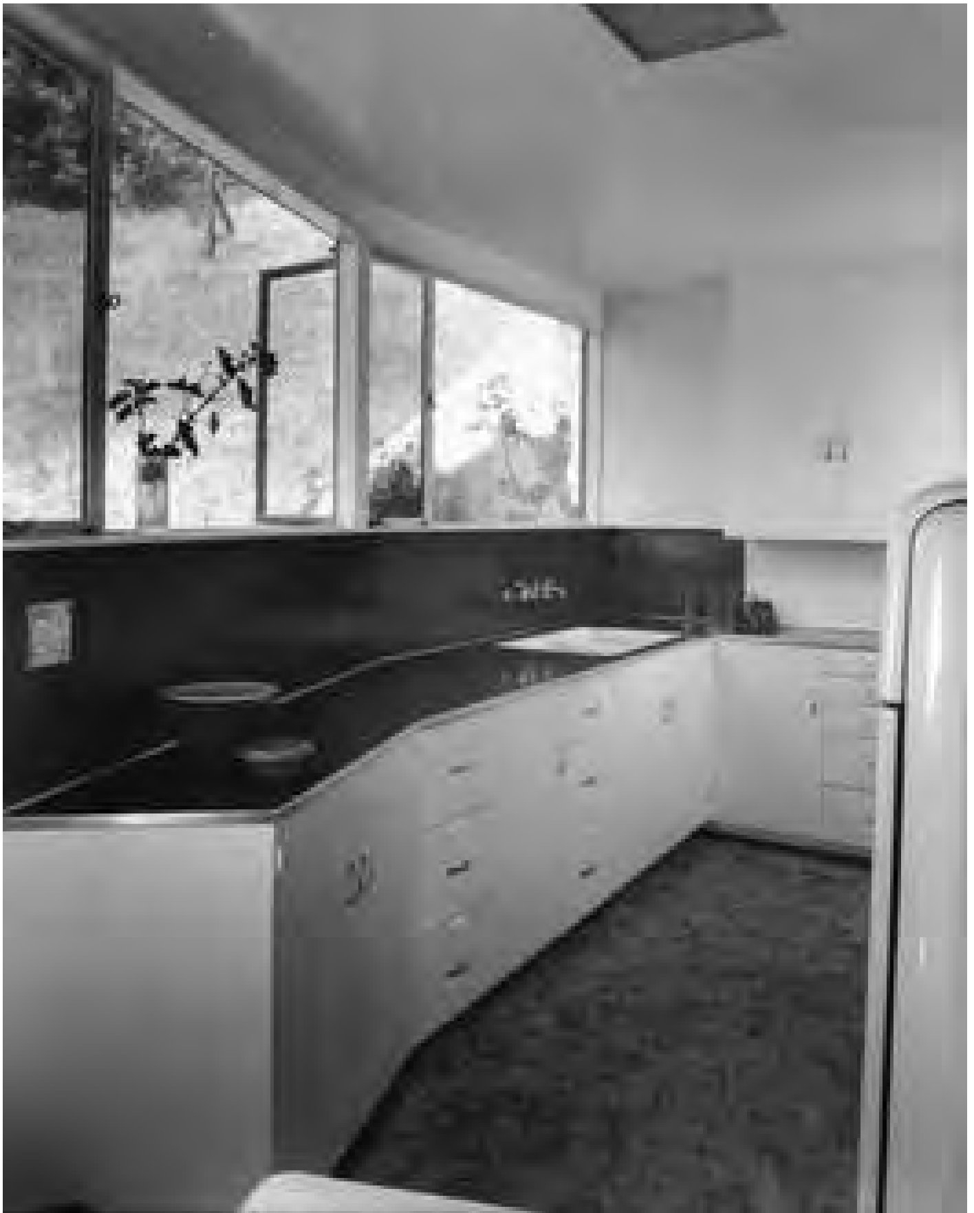
Bonnet House, original kitchen, 2256 El Contento Drive, circa 1942 (Unknown Photographer)
