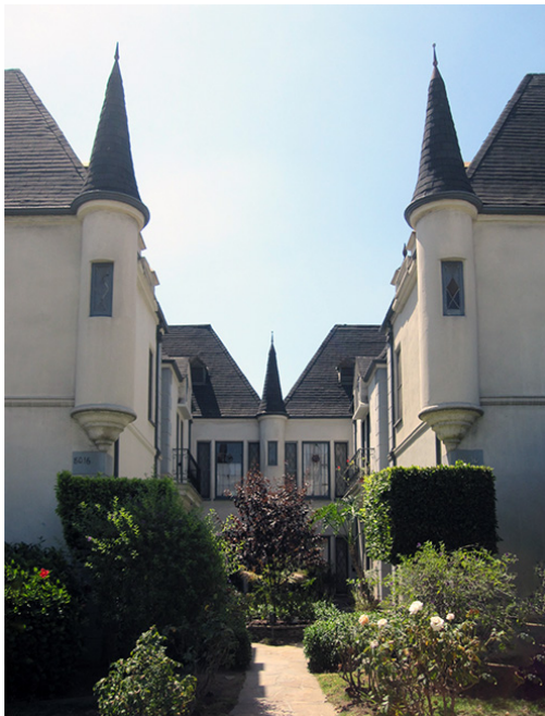
French Revival Courtyard Apartment at 8016 W Selma Avenue, Hollywood, 1937 (SurveyLA)
