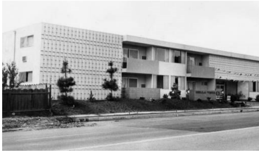
Bella Vista Apartments, 1963, altered; 17938 Burbank Blvd, Encino, (Valley Times Collection, Los Angeles Public Library)
