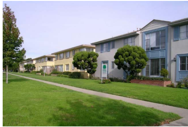
Mid-Century Modern and Minimal Traditional Apartments in the Barrington Multi-Family Residential Historic District, Mar Vista, 1953 (SurveyLA)
