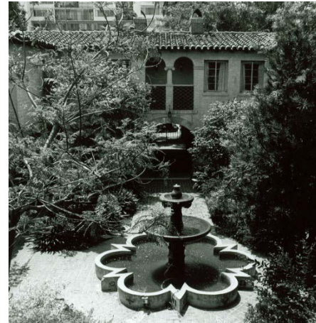
El Cabrillo Apartments, 1832-1850 N Grace Avenue, Hollywood, City Historic-Cultural Monument No. 773 (City of Los Angeles Office of Historic Resources)
