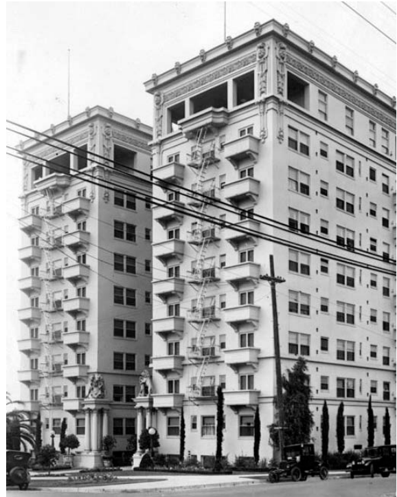
Beaux Arts Classicism/Mediterranean Revival Bryson Apartments at 2701 Wilshire Blvd., Westlake, City Historic-Cultural Monument No. 653 (Security Pacific National Bank Collection, Los Angeles Public Library)
