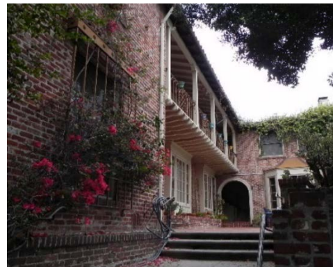
Spanish Colonial Revival Courtyard Apartment at 1972-1974 N. Palmerston Place, 1930, Los Feliz (SurveyLA)
