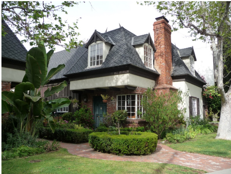
Tudor (late) Courtyard Apartments at 8227 Redlands Street, 1965, Playa Del Rey (SurveyLA)
