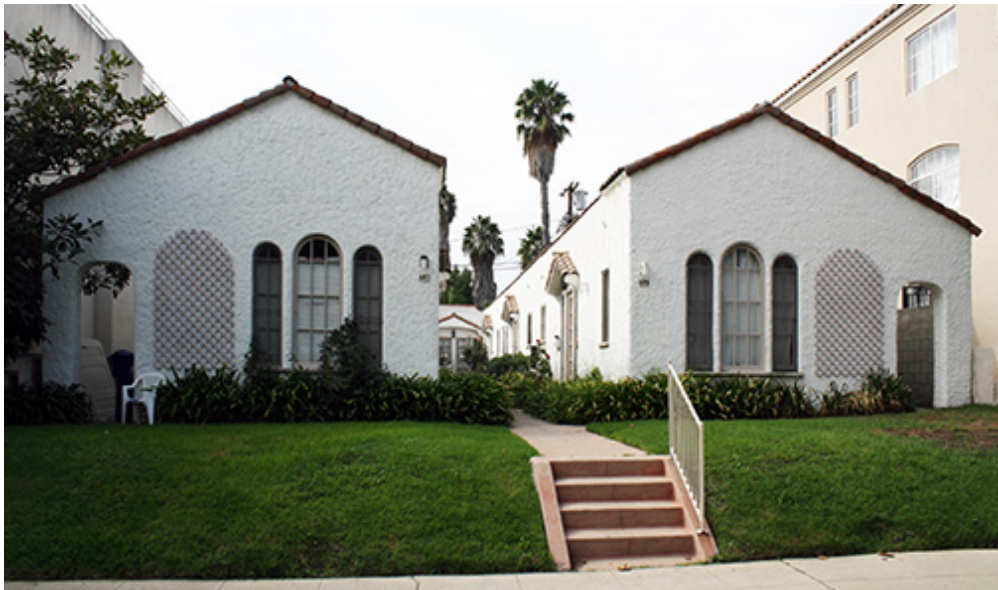
Spanish Colonial Revival Bungalow Court at 807-809 N Martel Avenue, Hollywood, 1926 (SurveyLA)
