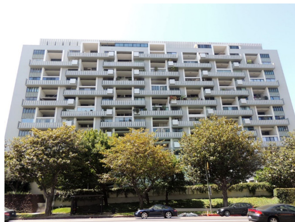
Mid-Century Modern Wilshire Terrace Apartments at 10375 Wilshire Blvd., Westwood, 1958 (SurveyLA)
