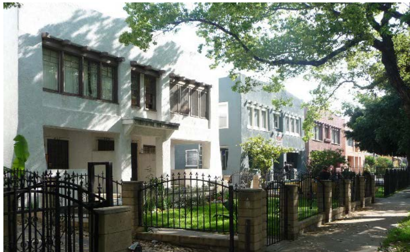
Spanish Colonial and Mediterranean Revival Apartments in Exposition Park Square Historic District dating from 1913-1928 (SurveyLA)
