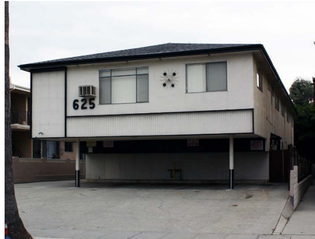
Contributor to the Hayworth Dingbat Apartment Historic District, 625 N Hayworth Avenue, Hollywood, 1958 (SurveyLA)
