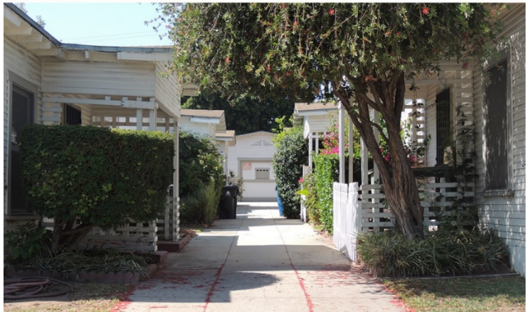
Craftsman Bungalow Court at 2320-2324 W Fair Park Avenue, Eagle Rock, 1922 (SurveyLA)
