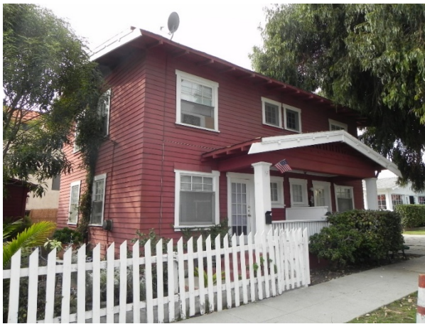
Two-story Craftsman Duplex at 519 W. 40 th Street, San Pedro, 1918 (SurveyLA)
