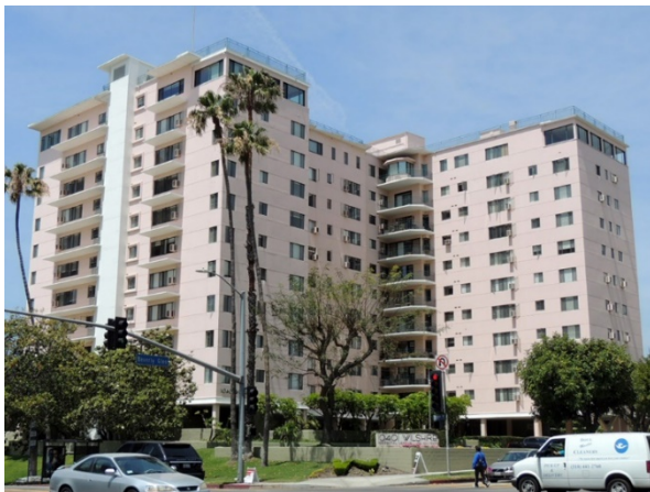
Mid-Century Modern Wilshire Manor Apartments at 10401 Wilshire Blvd., Westwood, 1951 (SurveyLA)
