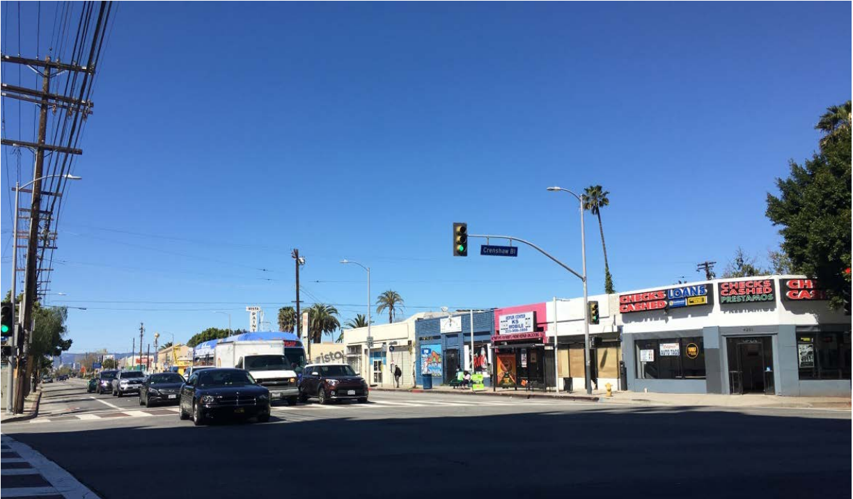
3. Neighboring properties on Pico Blvd., facing northwest.
