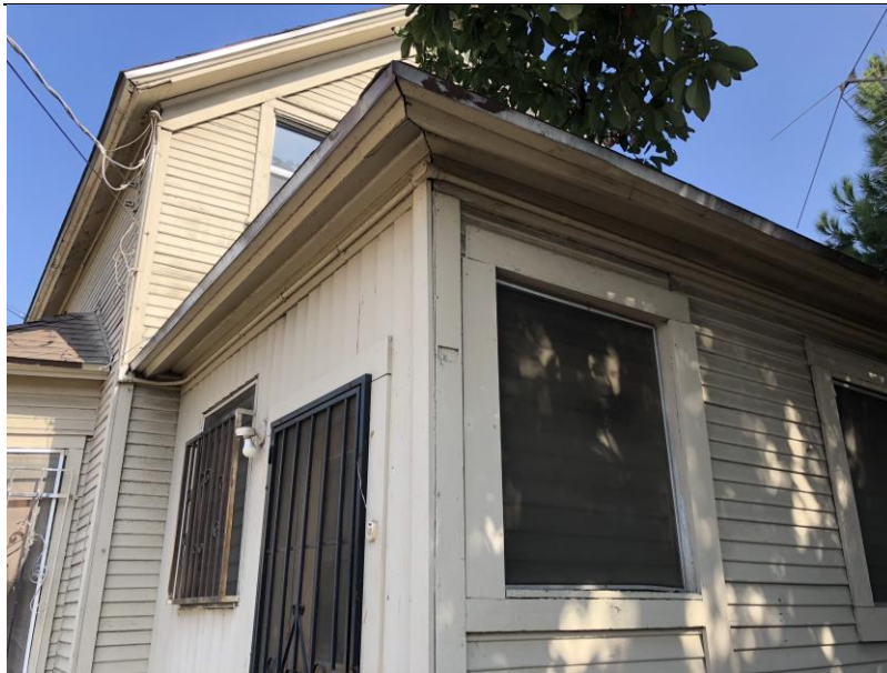
FIGURE 18: Southwest porch detail of altered siding and casing conditions
