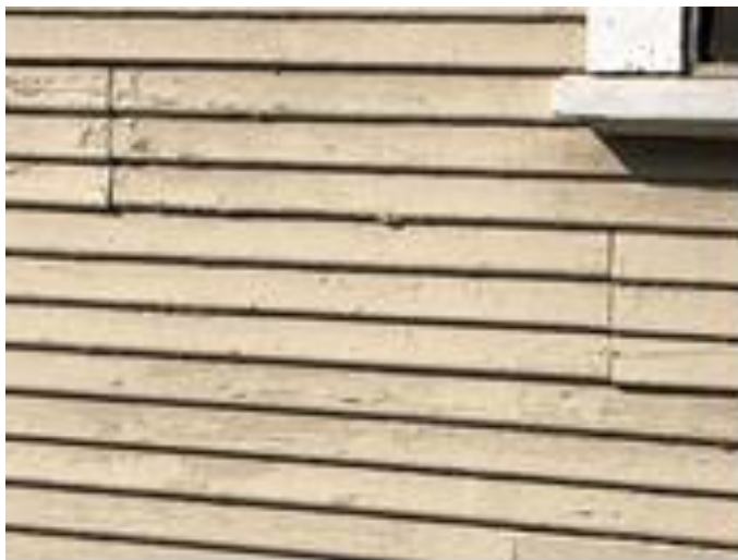
FIGURE 22: Tripled weatherboard detail using two faux joints; typical window sill detail
