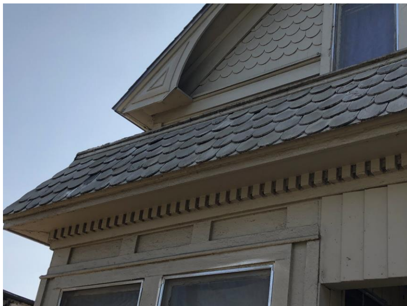
FIGURE 15: North façade detail of second floor porch, bay window head and gabled verge board end
