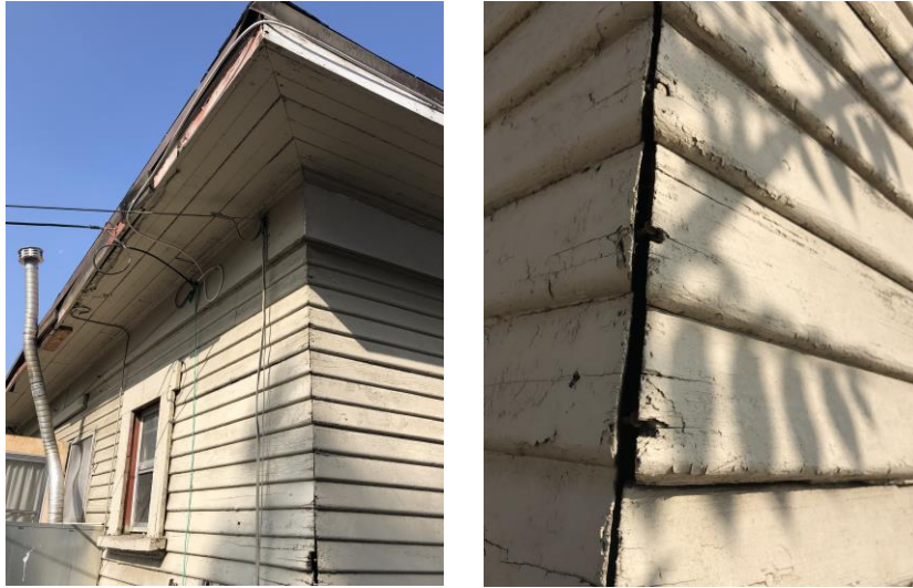
FIGURE 21: Southeastern corner with 2'6" projecting soffit; detail at mitred corner
