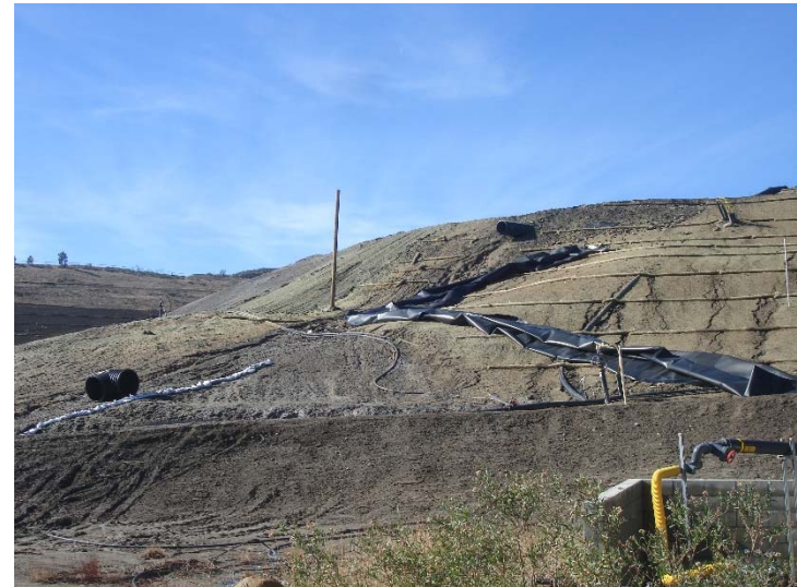
Photo 340: CC3B Slope Drainage Failure: January 10, 2018
