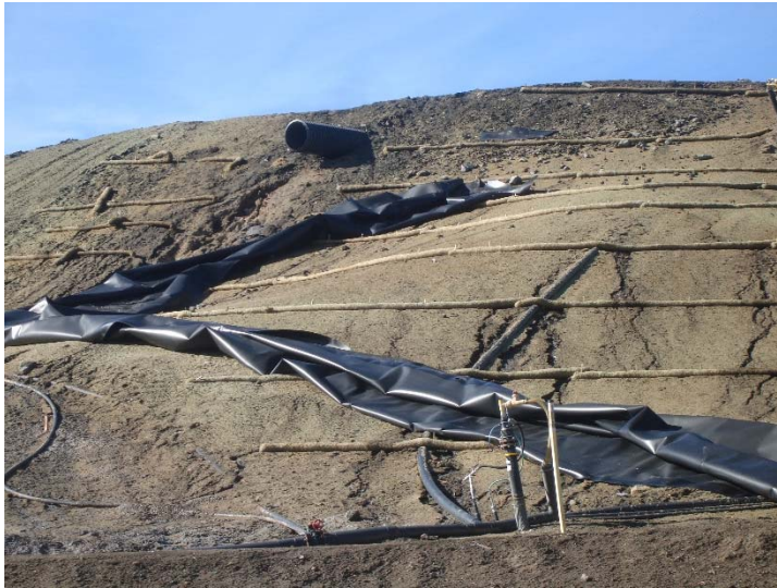
Photo 341: CC3B Slope Drainage Failure: January 10, 2018
