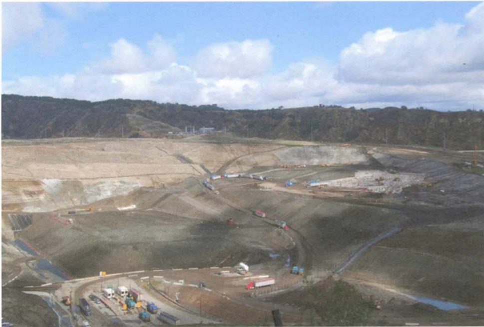
Photo 1 : Waste placement at Cell CC4
