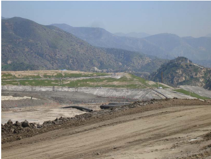
Photo 109: CC4A Part 1 with Posi Shell Slopes: March 29, 2018
