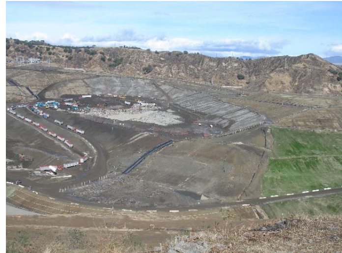
Photo 242: Closure Turf & Posi-Shell: January 10, 2018
