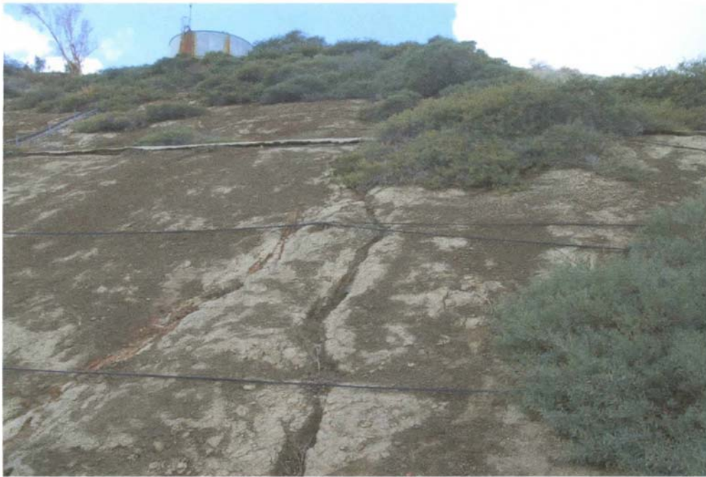
Photo 20: Undermined drainage channel on hillside near Flare 1
