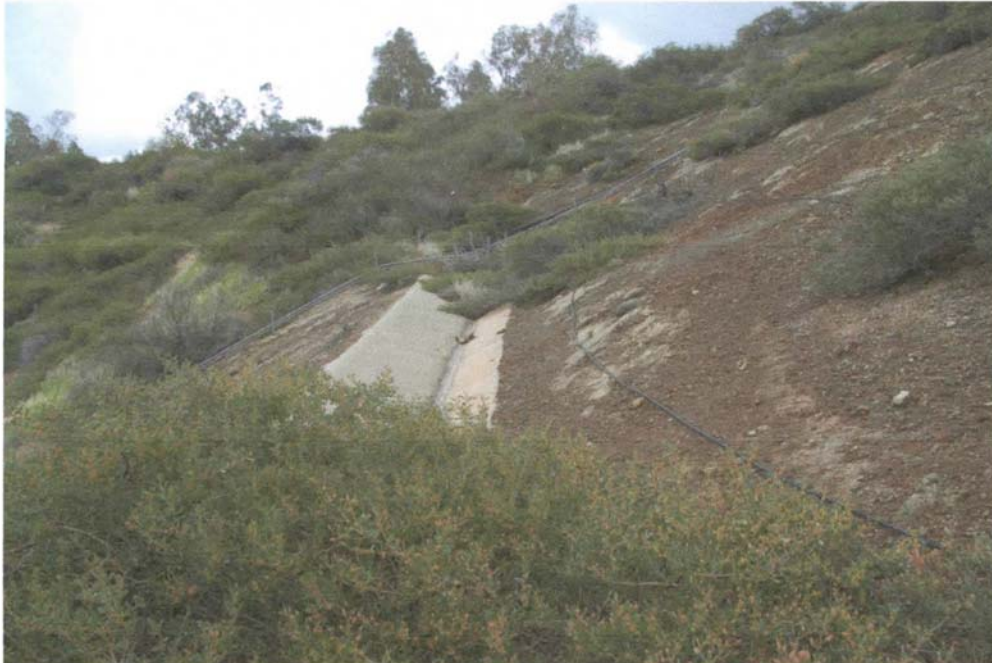
Photo 21: Sediment and vegetation in drainage channel on hillside near Flare 1
