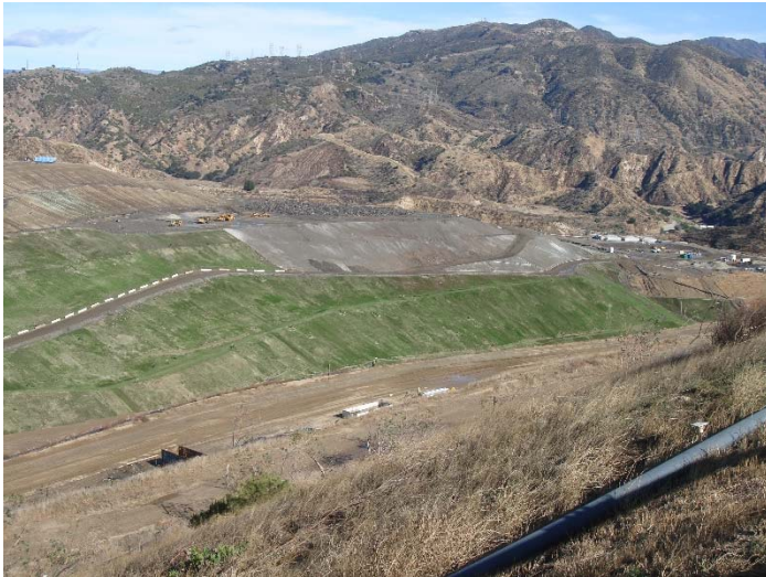
Photo 245: Closure Turf & Posi-Shell: January 10, 2018
