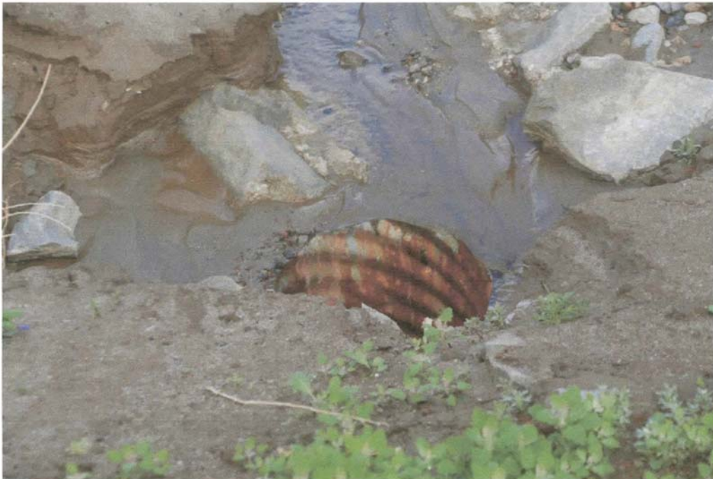
Photo 15: Unguarded intake to drain pipe in earthen basin at Cell CC3
