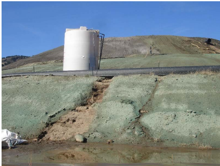
Photo 343: CC3B Slope Drainage Erosion: January 10, 2018
