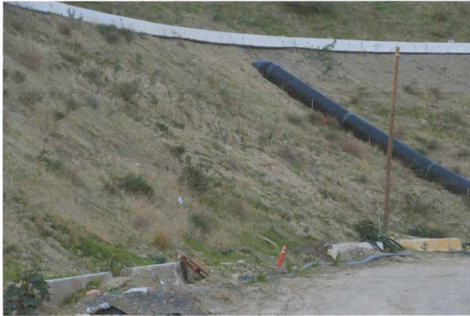
Photo 13: Sloughing Tilted Utility Pole on Embankment of Main Access Road near Entrance of Terminal Basin
