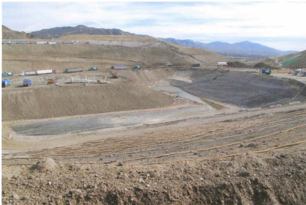
Photo 4: Water Channel Collection and Pond at Cell CC4 Phase 2
