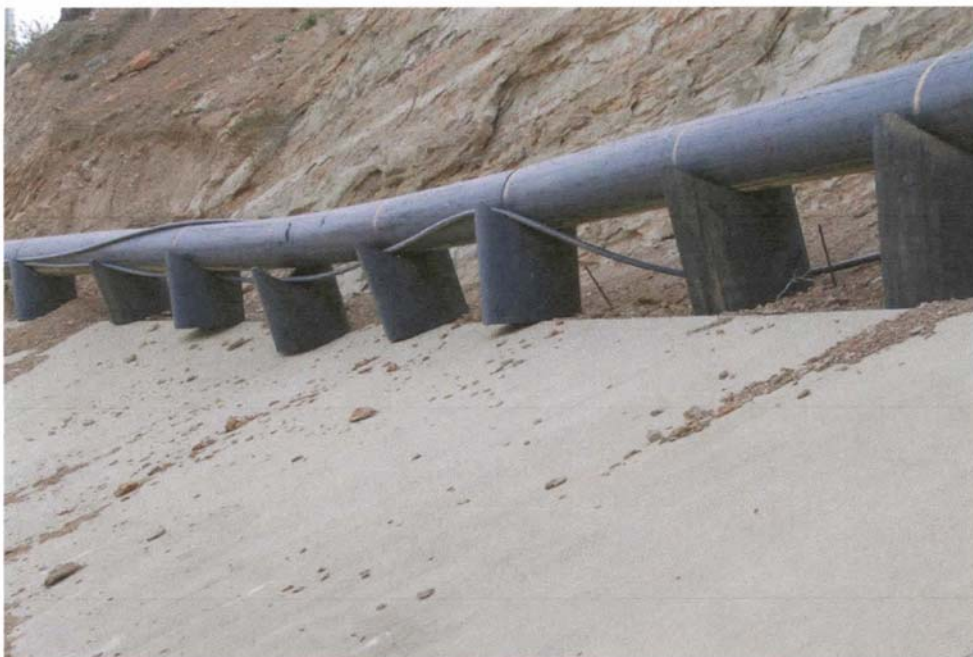
Photo 6: Leaning Supports of LFG Header to Flare 3 in Basin A
