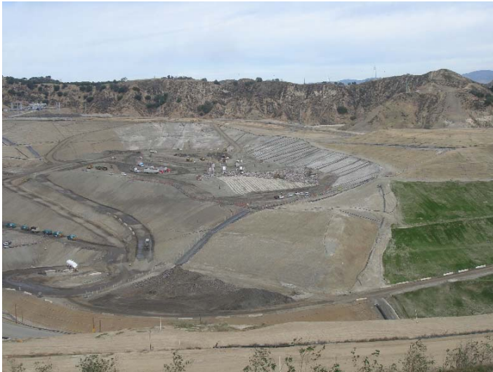
Photo 257: Closure Turf & Posi-Shell: January 30, 2018
