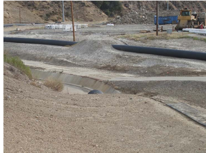
Photo 478: Plugged Drain at Flare 9-11 Access Road: January 30, 2018
