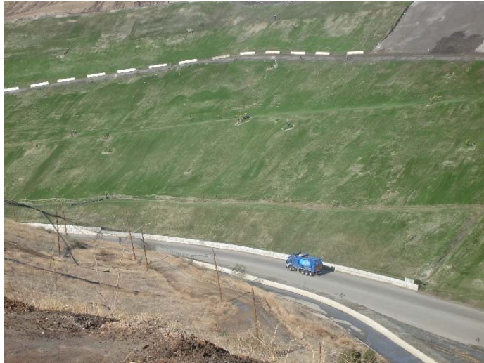
Photo 249: Closure Turf & Posi-Shell: January 10, 2018
