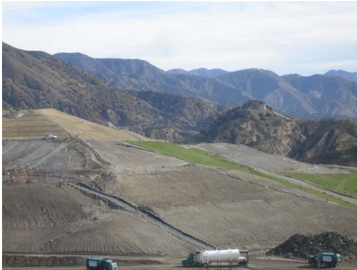
Photo 261: Closure Turf & Posi-Shell: January 30, 2018
