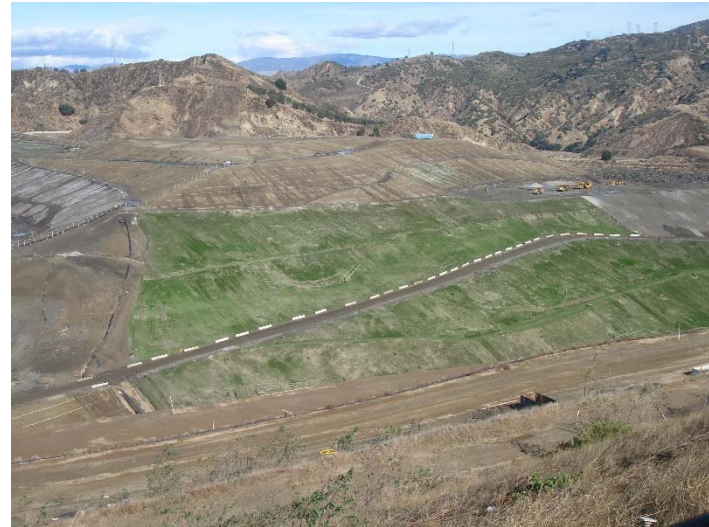
Photo 244: Closure Turf & Posi-Shell: January 10, 2018
