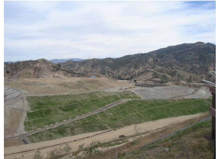
Photo 262: Closure Turf & Posi-Shell: January 30, 2018
