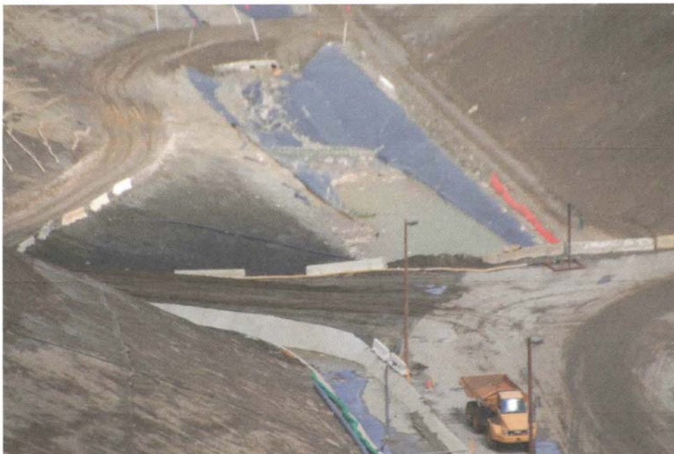
Photo 1 : Waste placement at Cell CC4
