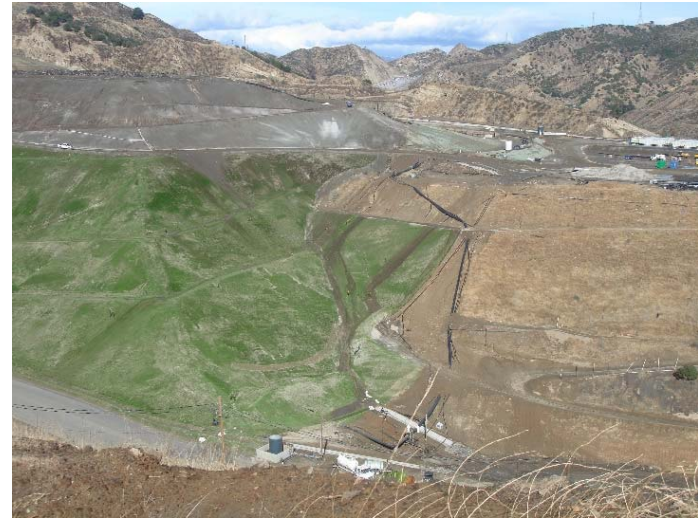
Photo 250: Closure Turf & Posi-Shell: January 10, 2018
