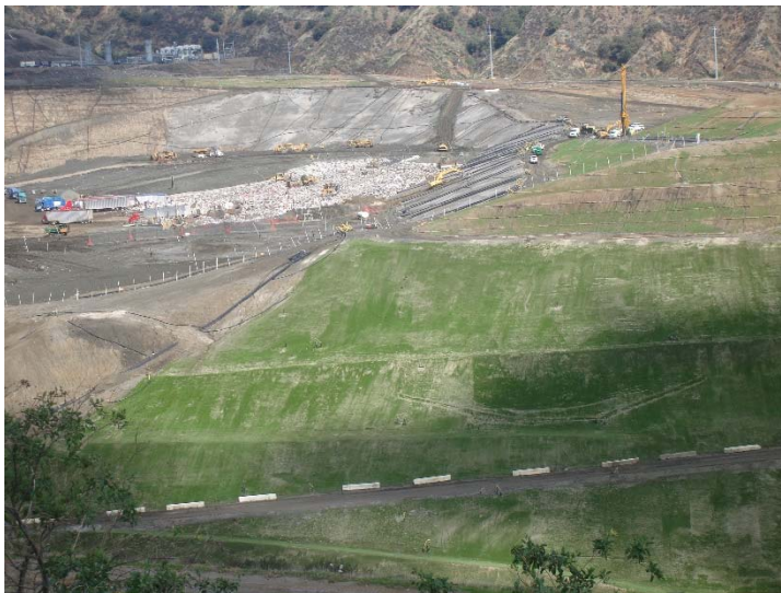
Photo 295: Posi-Shell and Closure Turf: March 14, 2018
