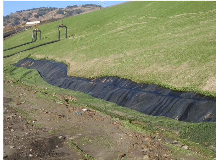
Photo 254: Closure Turf & Posi-Shell: January 10, 2018
