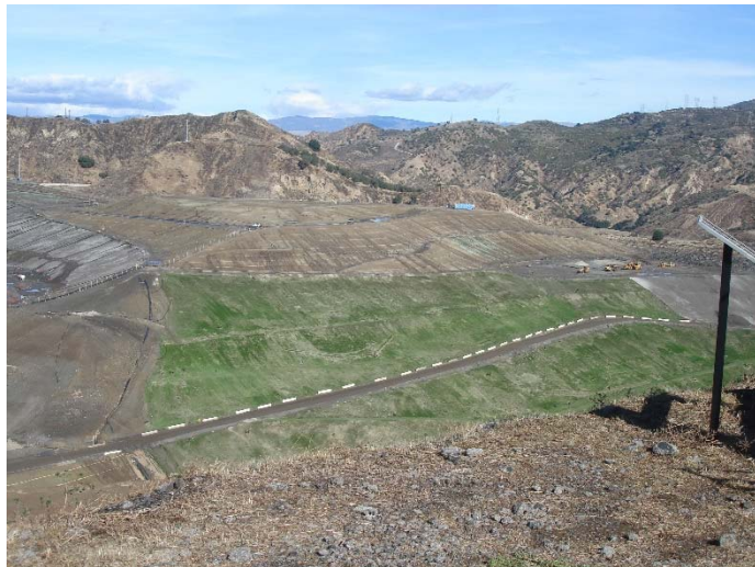
Photo 243: Closure Turf & Posi-Shell: January 10, 2018
