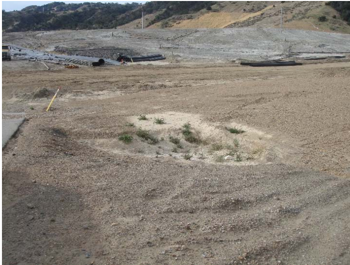
Photo 477: Plugged Drain at Flare 9-11 Access Road: January 30, 2018
