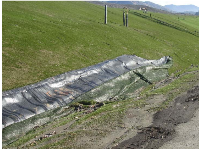
Photo 256: Closure Turf & Posi-Shell: January 10, 2018
