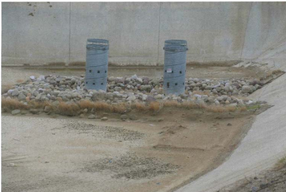
Photo 10: Sediments Accumulated in Basin B
