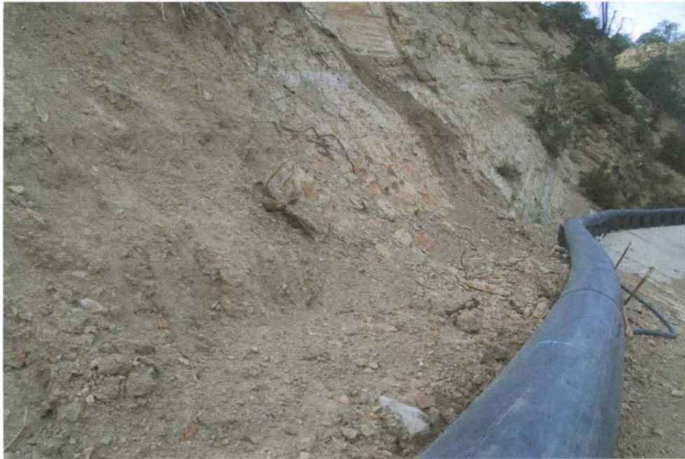
Photo 7: Sloughed Soil and Pushing Against f LFG Header to Flare 3 in Basin A
