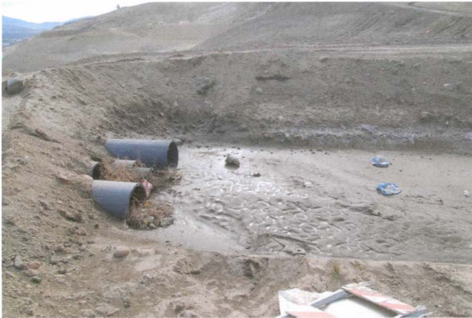
Photo 9: Sediments Accumulation Downgradient from Basin A – Pipes do not offer enough flow capacity
