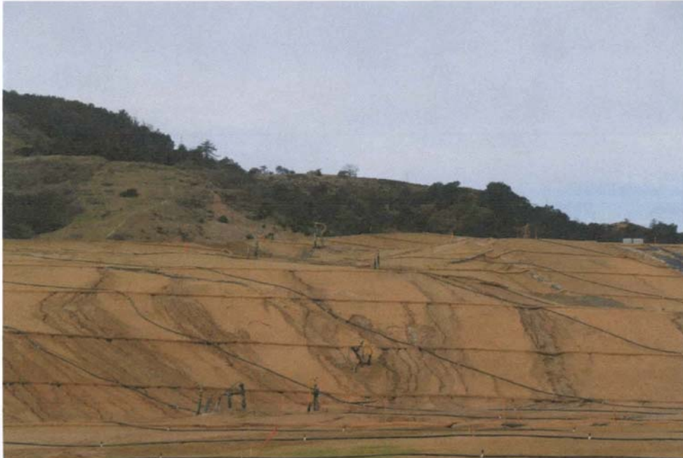
Photo 5: Gullies on Hydro seeded Slope – Note Gullies Under Wattles
