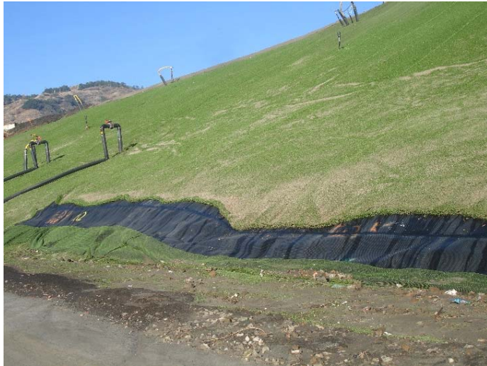
Photo 253: Closure Turf & Posi-Shell: January 10, 2018
