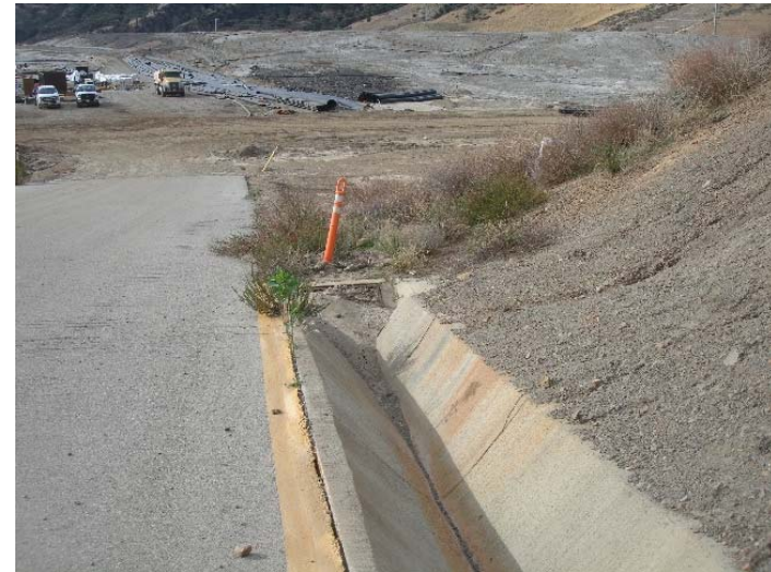
Photo 476: Plugged Drain at Flare 9-11 Access Road: January 30, 2018
