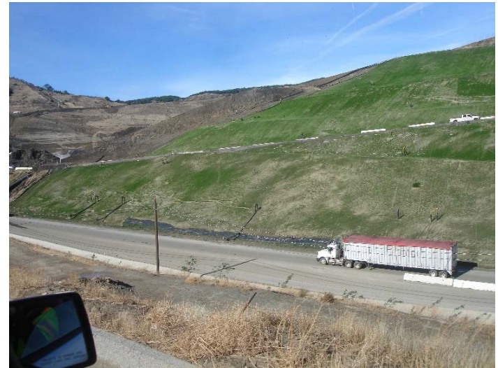
Photo 248: Closure Turf & Posi-Shell: January 10, 2018
