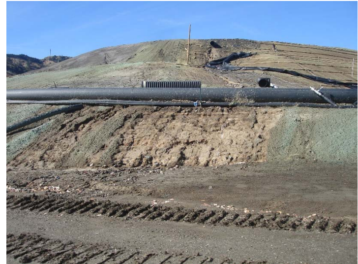
Photo 342: CC3B Slope Drainage Erosion: January 10, 2018
