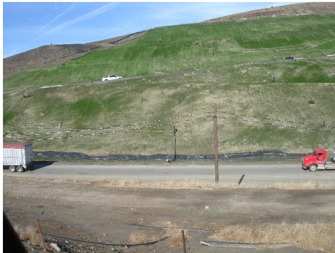
Photo 247: Closure Turf & Posi-Shell: January 10, 2018
