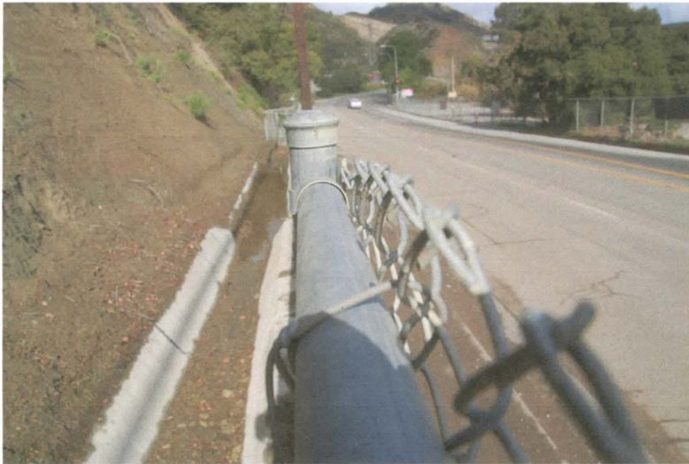
Photo 18: Soil in drainage swale on top of wall along San Fernando Road
