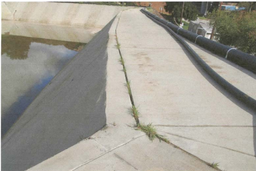
Photo 19: Gap between slabs at Terminal Basin
