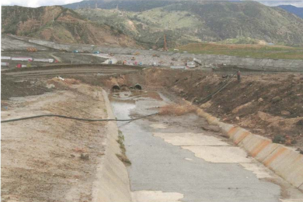
Photo 10: Sediments Accumulation Downgradient from Basin A – Pipes may not offer enough flow capacity
