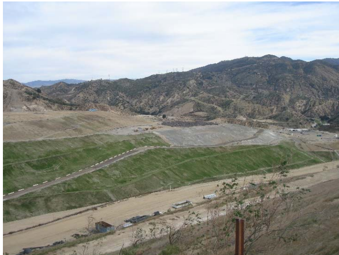
Photo 263: Closure Turf & Posi-Shell: January 30, 2018
