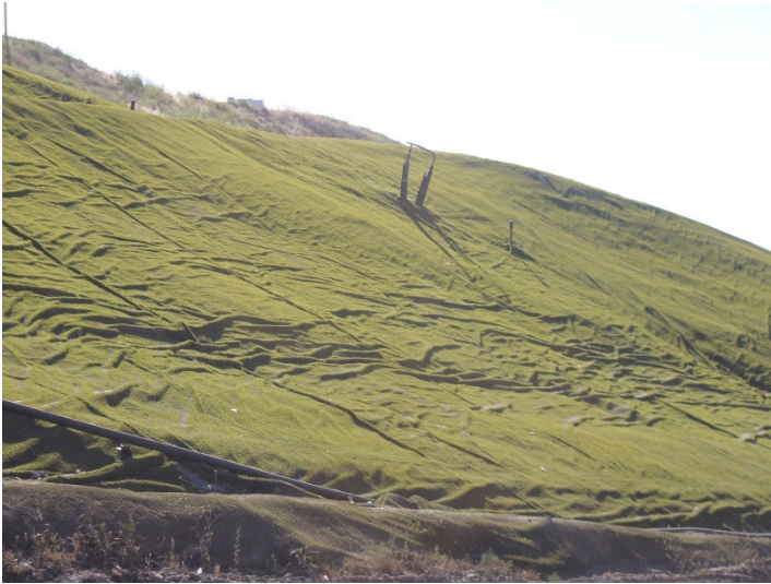
Photo 137: Closure Turf: June 21, 2023
