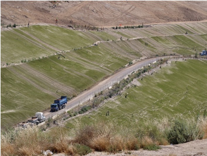
Photo 139: Closure Turf: June 21, 2023
