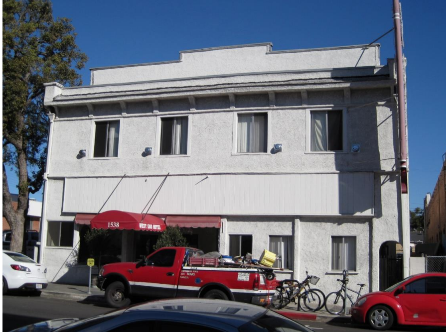
Business Block 1538 Sawtelle Boulevard (Photo by author)
