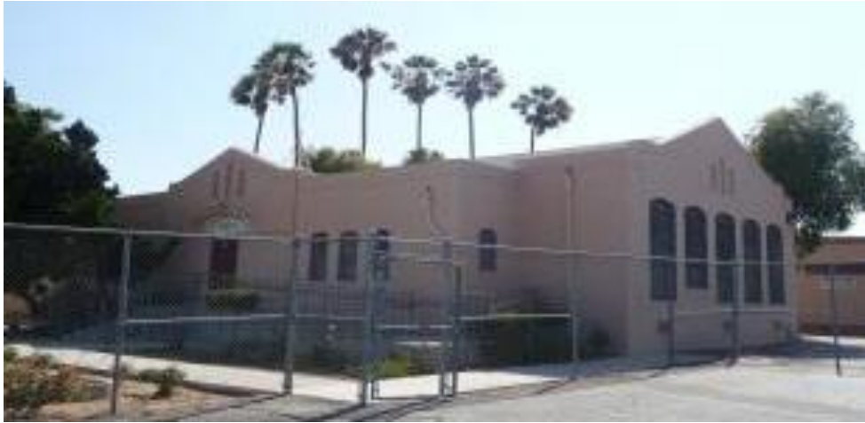
Current view of probable Hyde Park School building 6525 Eighth Avenue (SurveyLA)
