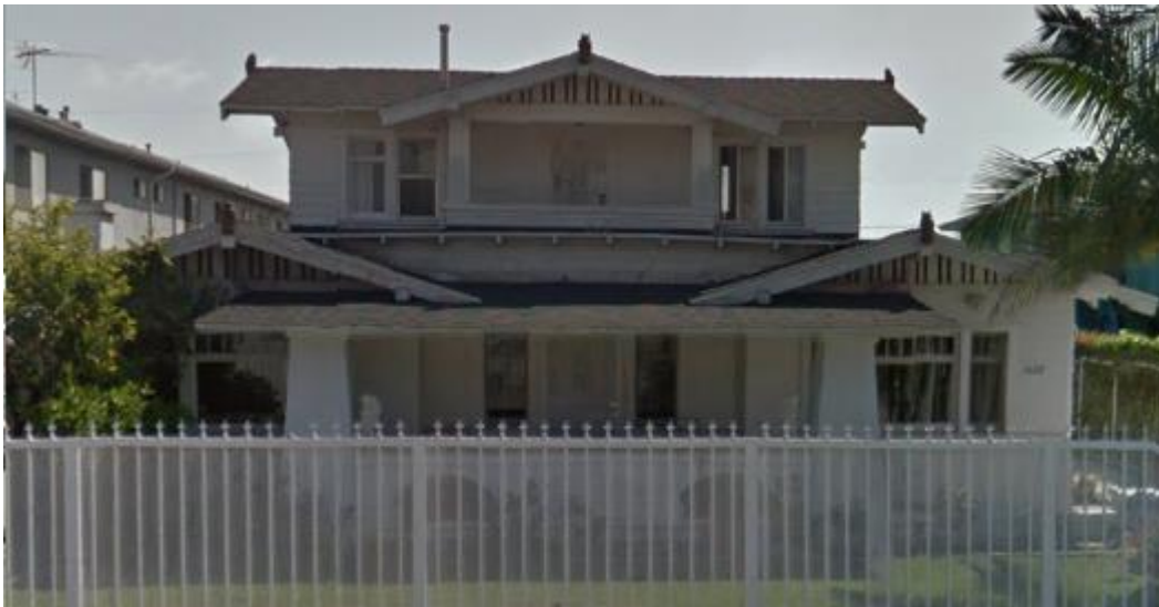
Residence 6122 South Victoria Avenue (©2015 Google Street View)
