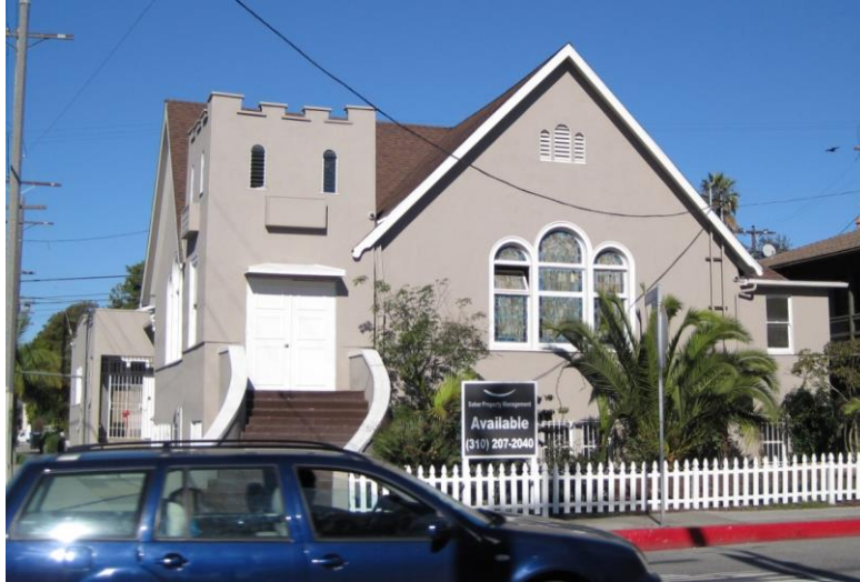
Christian Church Northeast corner of Rose Avenue and Hampton Drive (Photo by author)
