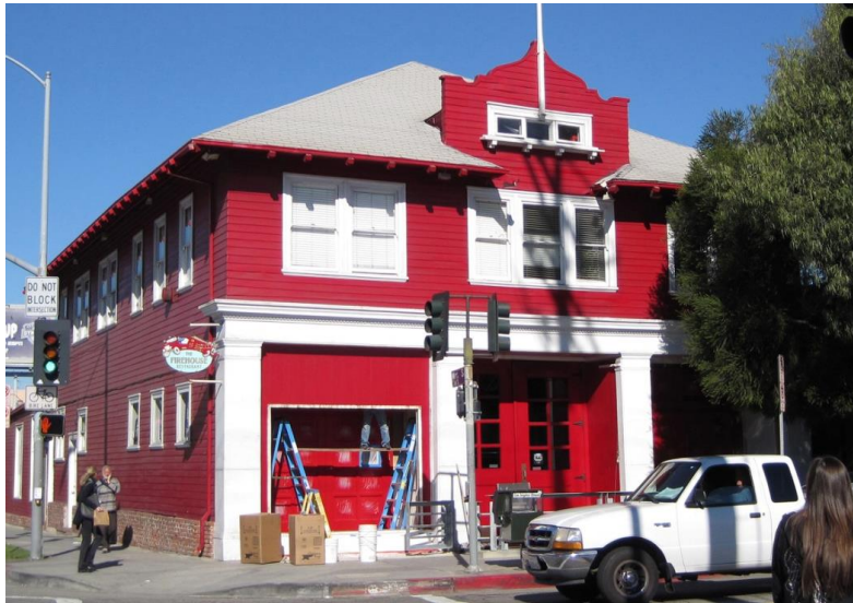
Venice Fire Station
