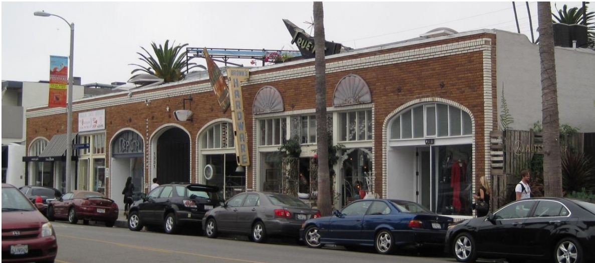
Bundy Building 1327-1335 Abbot Kinney Boulevard (Photo by author)
