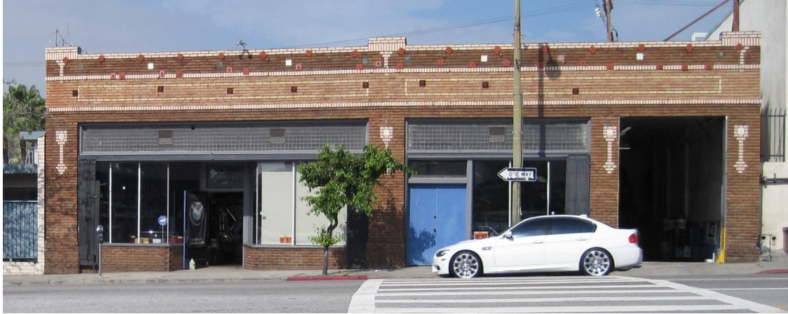
Business Block from the early 1920s 5041 Eagle Rock Boulevard (Photo by author)
