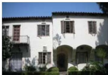
*These wood casement windows have thin, delicate grids and are recessed in the openings.*
