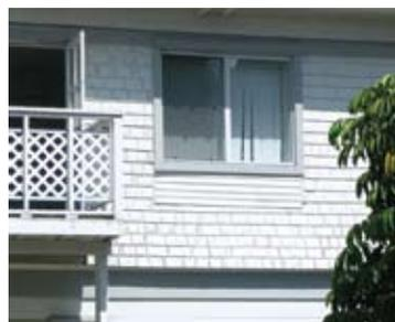
*The siding added to the bottom of the window does not match the original shingle siding.*
