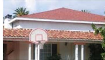
*Part of the original clay tile roof has been changed to asphalt shingle.*
