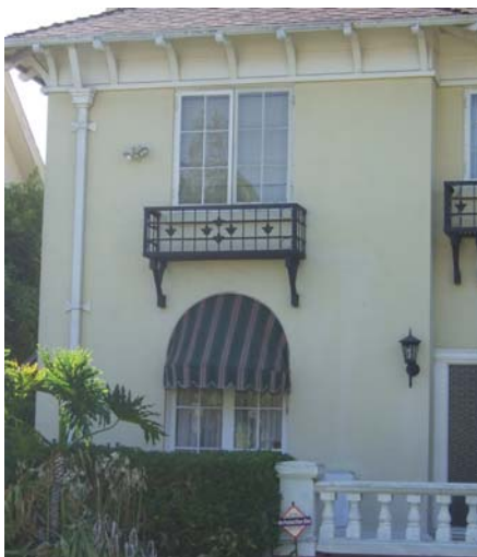
Awnings should be shaped appropriately for window openings and should be consistent with the architectural style of the house.
