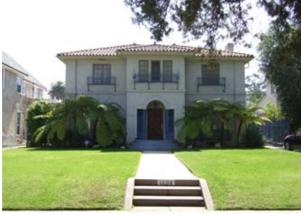
The front porch on this home has been enclosed and the appearance of the columns altered. Such changes diminish the character of the home and District.
