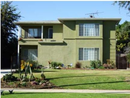
Porches serve an important function at a home's entryway that should be preserved. The enclosure of this porch has obscured the entry and barcaded the house from the streetscape.
