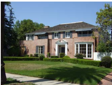
Architectural styles such as Colonial Revival, English Tudor Revival and Minimal Traditional would not ordinarily have a front porch but would often have a decorative crown and pilasters.
