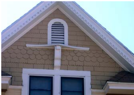
This home has specialty "fishscale" shingles. When repairing these shingles, it is important to "piece in" materials that match the original.
