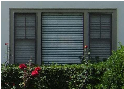
Fixed pane picture window flanked by 4 over 1 double-hung windows
