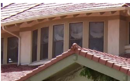
Curved window bay with five double-hung windows
