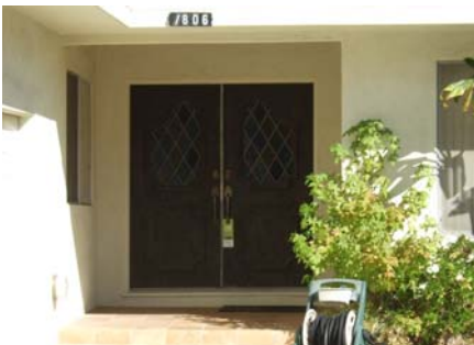
Though often found on Contemporary style homes, double doors are rarely found on the Period Revival, Craftsman and Prairie style homes in the District.
