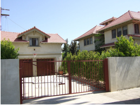
This carriage house retains original details included a dormer that may have at one point housed a hoist to an upper floor storage area. The homeowner has taken care to retain these features while converting the space for guest quarters.
