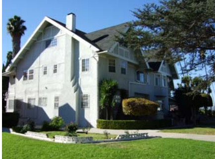
These replacement windows (on both the side and front of the house) have dramatically altered the character of the house and the surrounding district.
