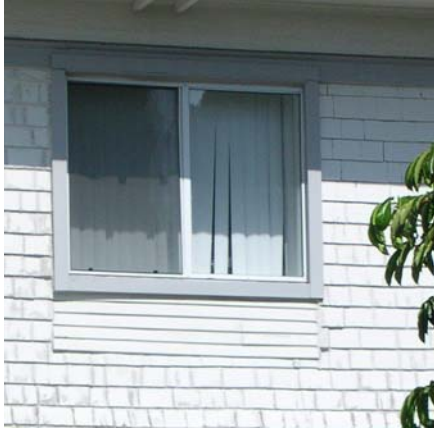
It is inappropriate to replace wood siding with siding that does not look the same as the original. It is important to use the same kind of wood, and to match the original in size, profile, and finish.
