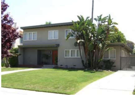
The single pane casement windows on this house maintain the simplicity that is intended by the architectural style.
