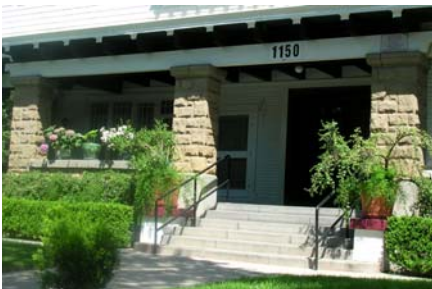
River rock is an important material used in Craftsman style homes and should be preserved. It is inappropriate to paint the river rock.
