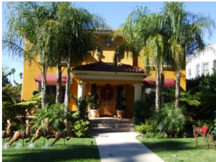
Materials such as styrofoam plant-on sills, faux-decorative plaster reliefs and mosaic tile are inappropriately applied to this home and diminish its historic integrity.
