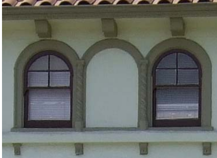
Decorative 4 over 1 arched windows
