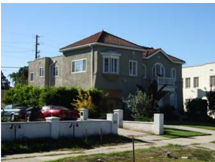
When re-surfacing a stucco home great care should be taken to match the appropriate texture, color and stucco mixture. The rough-texture and dark color of stucco on this home diminish its appearance.
