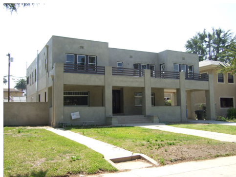
The International Style home at 1740 Virginia was remodeled from a Period Revival style in 1922 and is actually the oldest home in the District. The home was under restoration at the time of this photograph.
