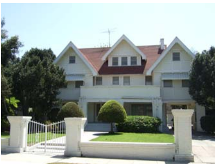
A third floor attic dormer. Few homes in the District feature front-facing dormers at the third floor.
