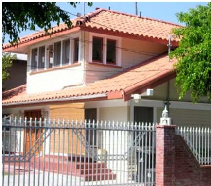
Inappropriate materials can also destroy the historic character of a structure. In this case, clay tiles should not be used on a Craftsman style home.
