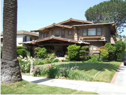
This home has decorative wood work, siding, and intricately carved rafter tails.
