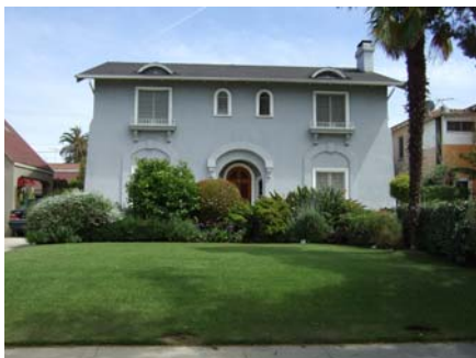
Though simple, the windows on this home are arranged in a pattern that is typical to homes of this style in the District and they are a significant character defining feature.
