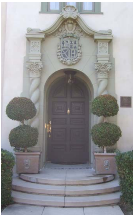
The highly ornate entryway with a single arched door is typical of the Spanish Colonial style and is a significant feature on the home.
